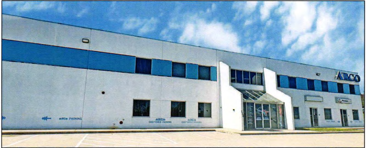
Figure 2: Street view of site.
