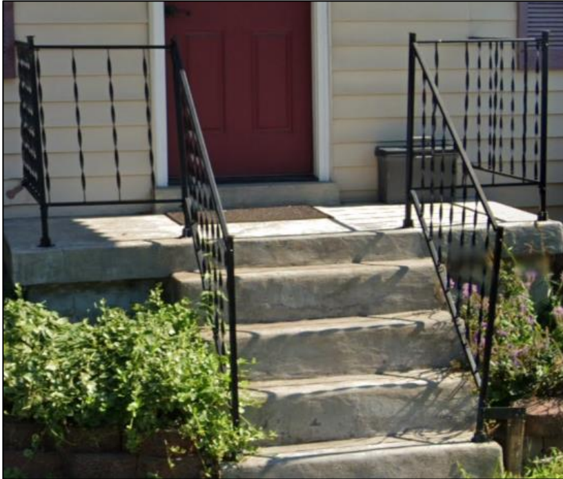
Figure 6: Previous aluminum railing on the property.
