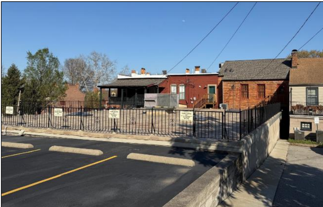
Figure 3: Rear of property and proposed location for addition.
