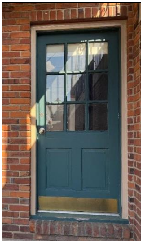
Figure 7: Rear door proposed for like-for-like replacement.
