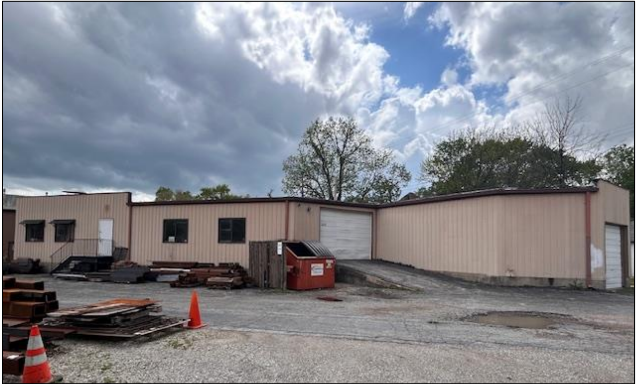
Figure 8: Existing metal-clad addition on north side of the property.
