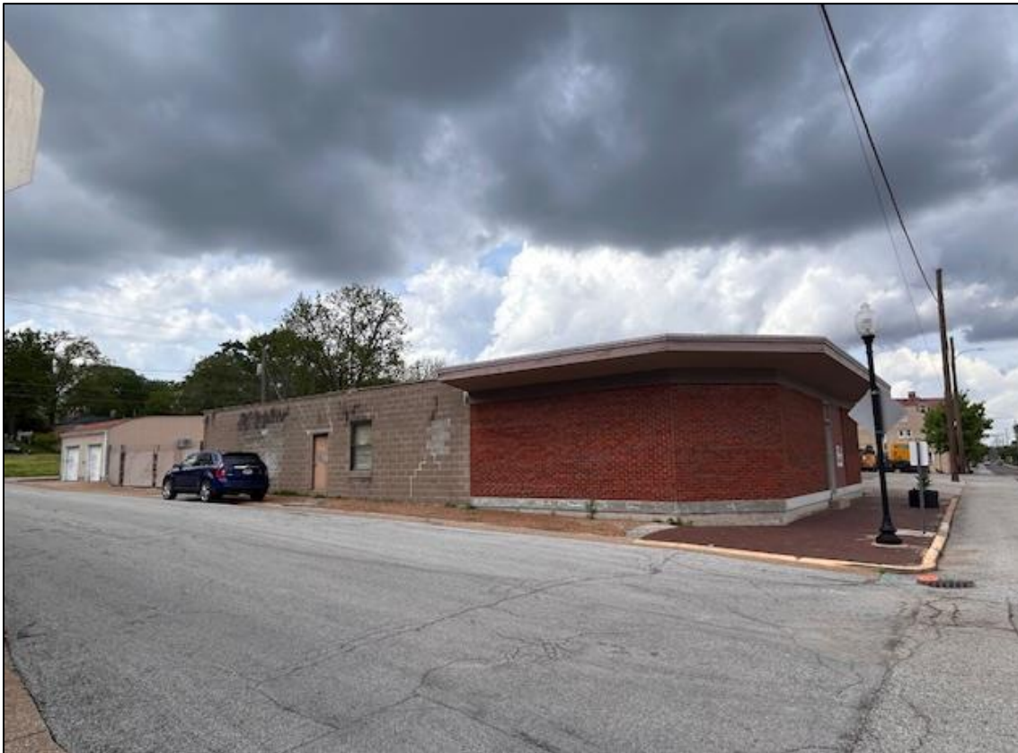
Figure 11: Property seen currently from Montgomery and North 2 nd Street intersection.
