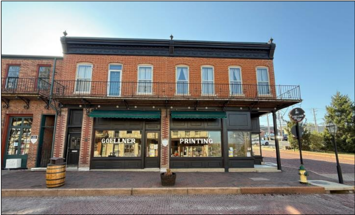
Figure 1: 301-305 South Main Street seen currently from South Main Street.
