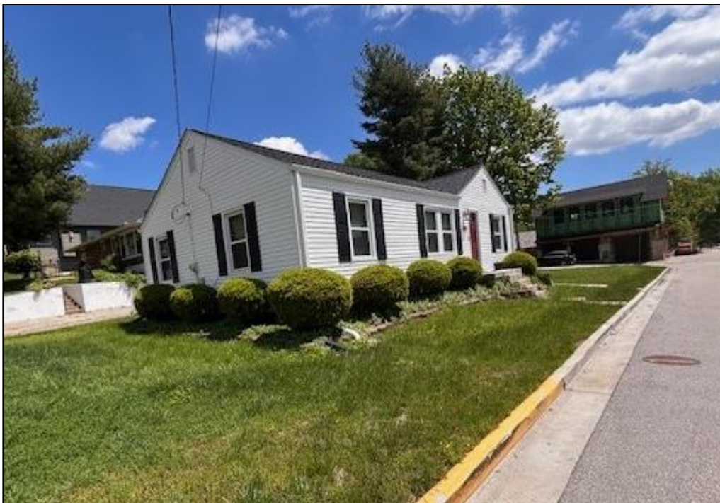
Figure 5: Porch seen from South 2 nd Street and Water Street intersection.
