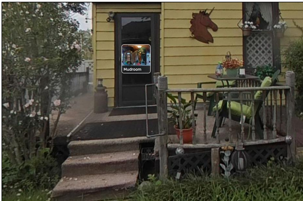
Figure 5: Previous rear deck on property.
