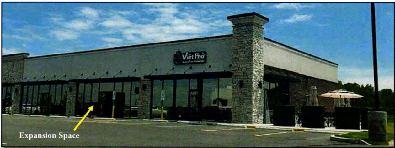
Figure 2: Street view of the building and tenant space.
