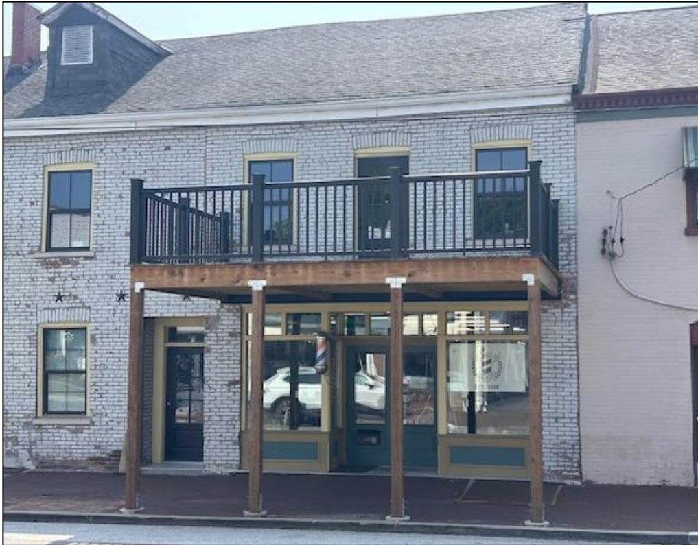
Figure 8: Example balcony at 918 North 2 nd Street.
