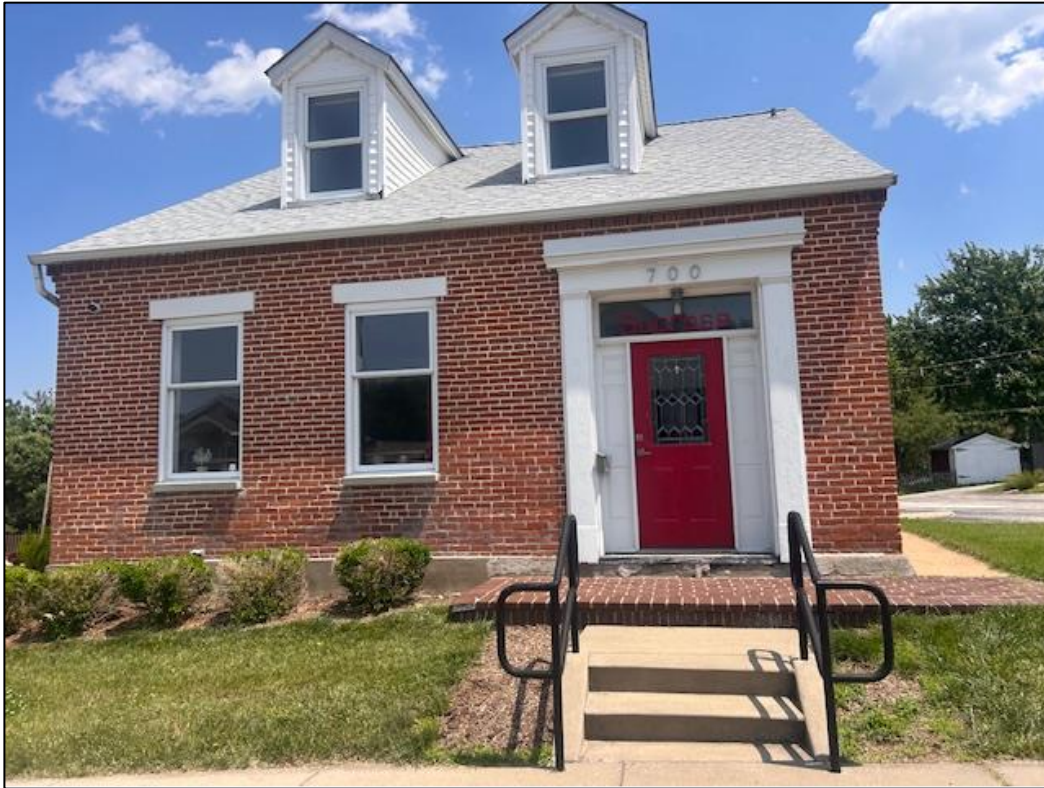
Figure 1: Front façade of subject property.
