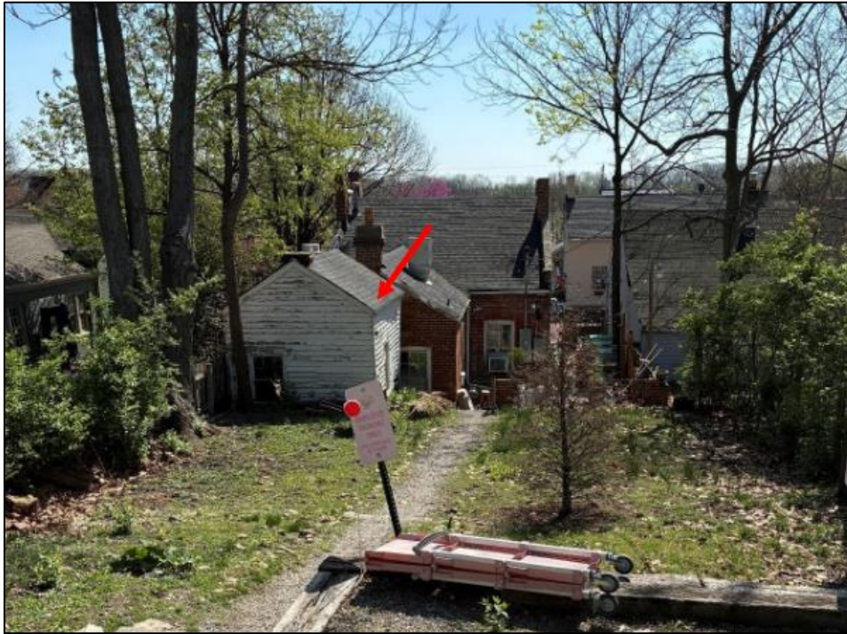
Figure 2: Subject structure seen from rear alley way.
