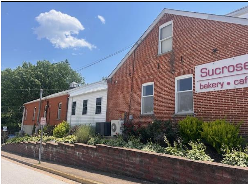
Figure 2: North elevation of the building along Perry Street.
