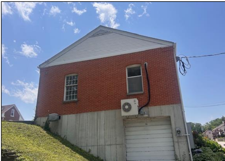
Figure 4: Rear of structure.
