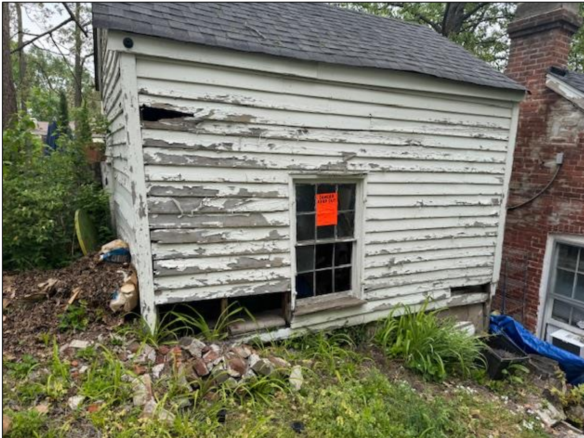
Figure 1: Subject structure in rear of property.
