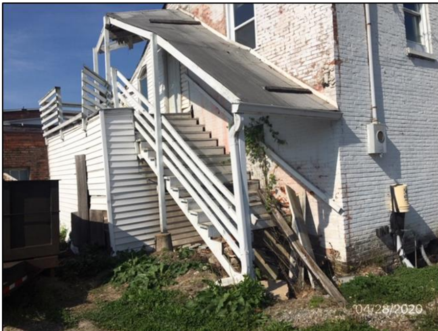
Figure 3: Subject property rear addition before demolition (April 28, 2020).
