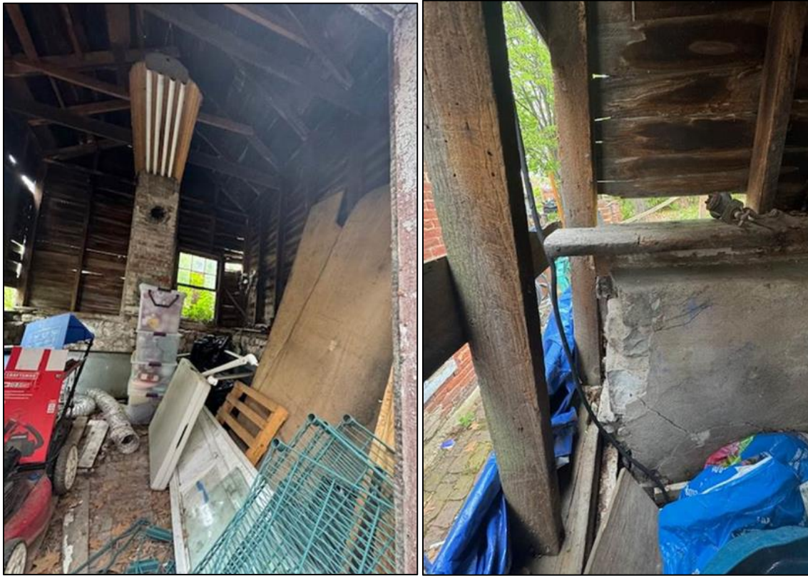
Figure 4: Photos of interior of the subject structure.
