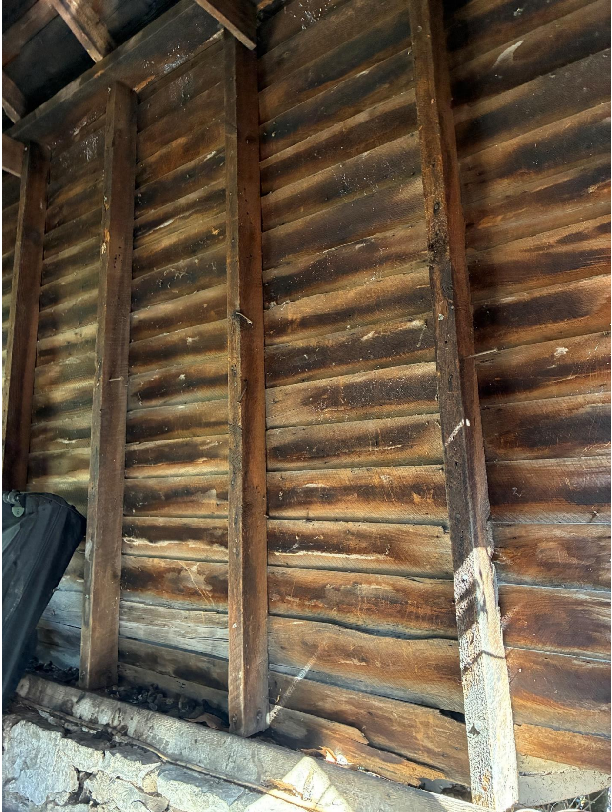
Photo 4: North wall structure & siding with circular kerfs. Siding exhibits evidence of hand planed laps
