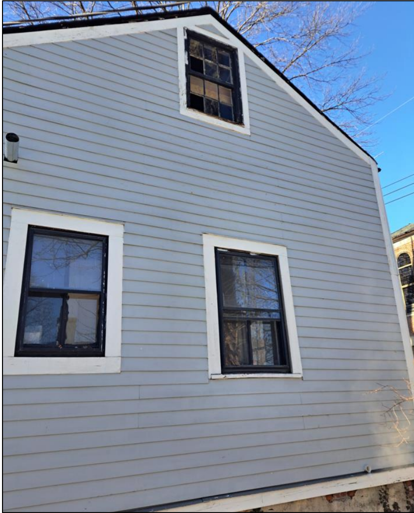
Figure 8: Previously approved siding seen on the property
