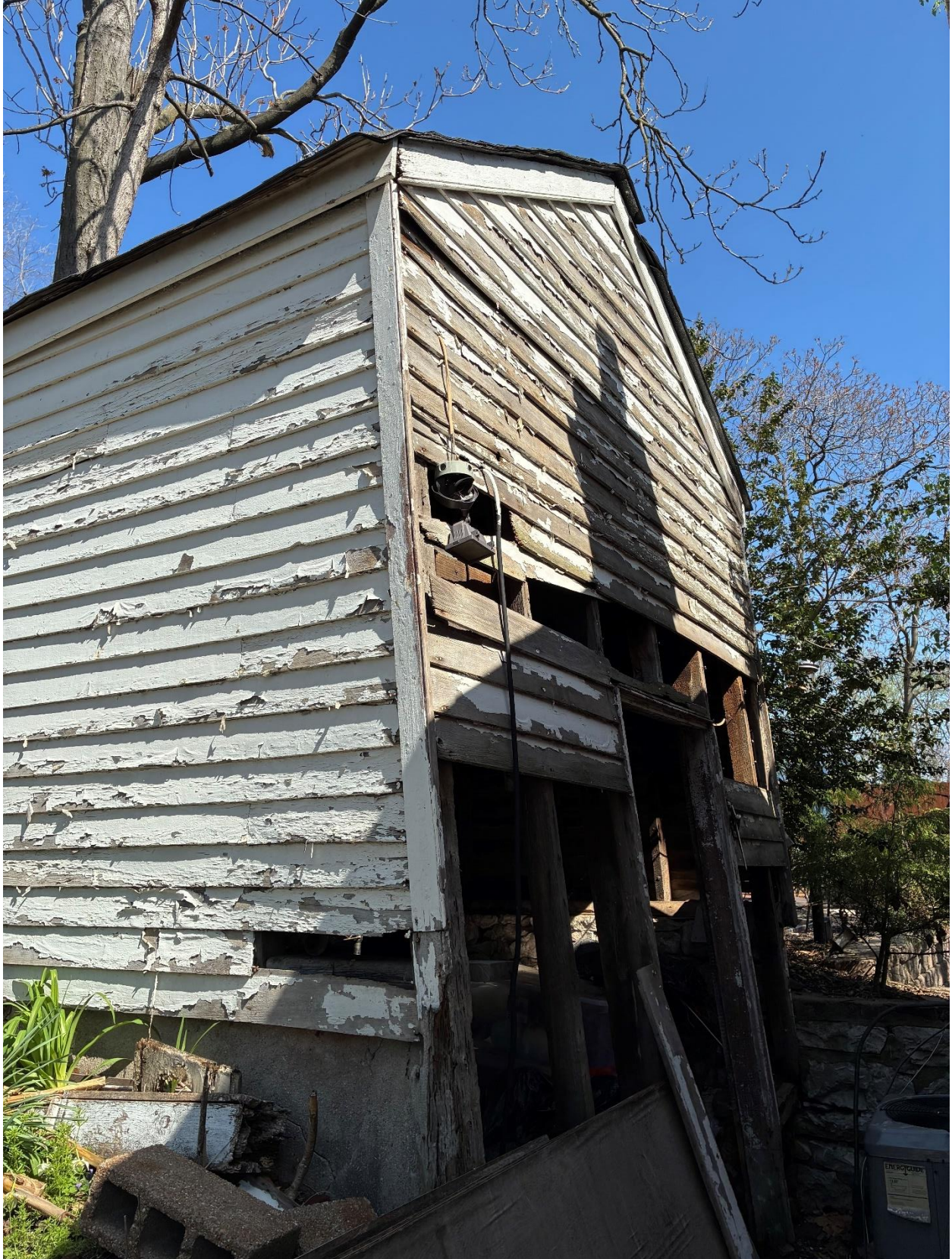
Photo 1: View facing north/northwest. Entrance and retaining wall visible right
