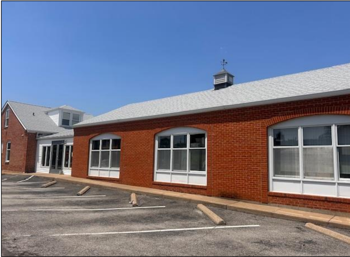
Figure 3: South elevation of the structure.
