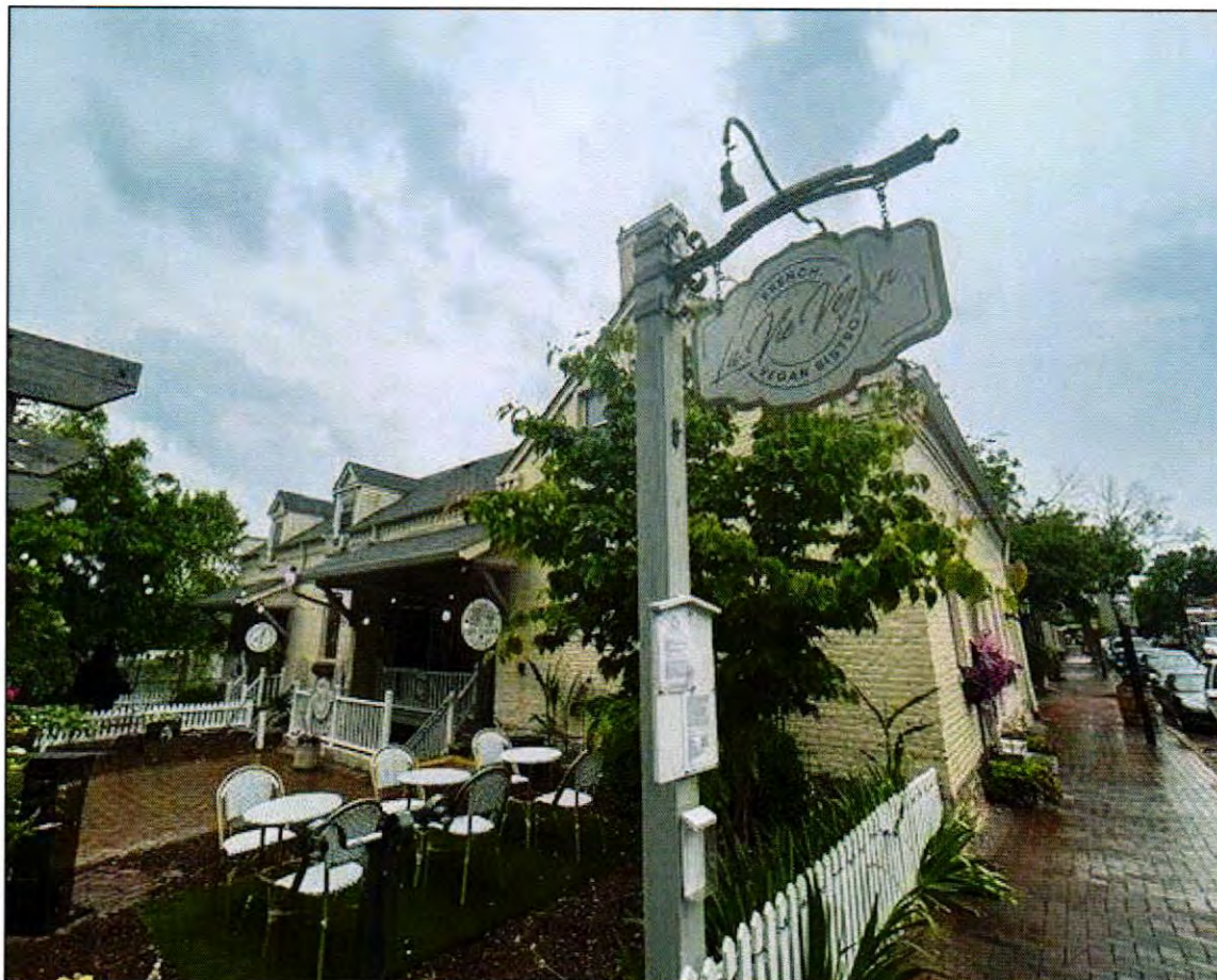
Figure 1: Subject property and restaurant seen from South Main Street.
