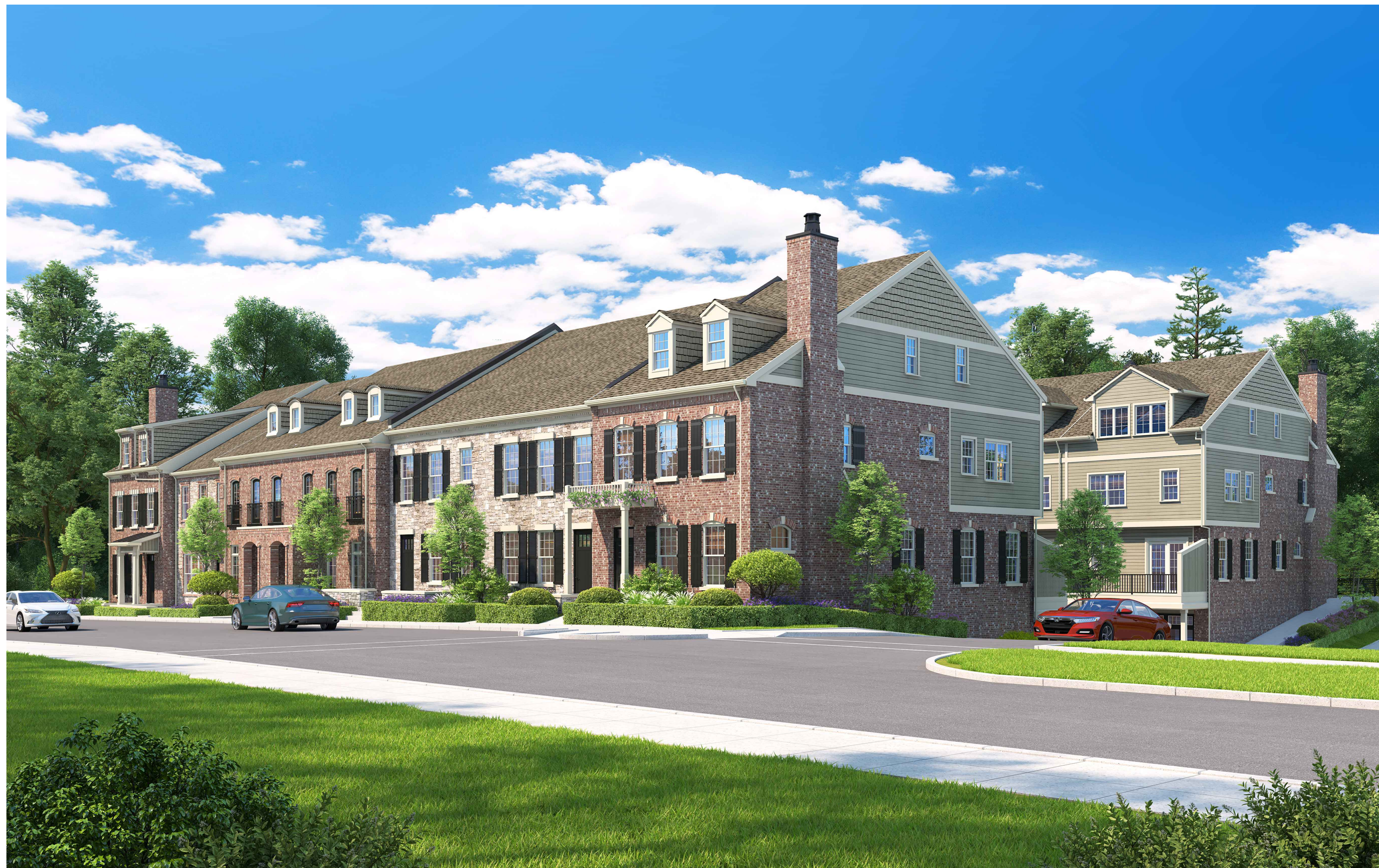
VIEW FROM THE SOUTHEAST NEAR SOUTH MAIN STREET AND BARBOUR STREET
