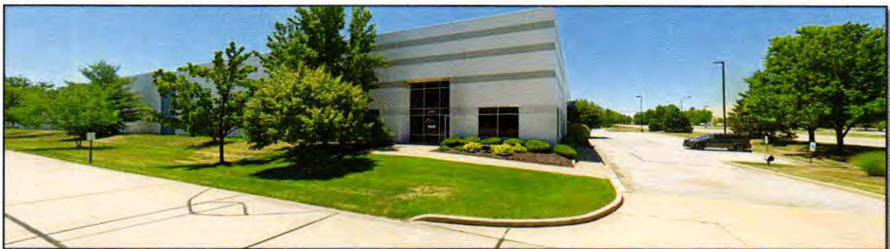
Figure 2: Street View of the Subject Property.
