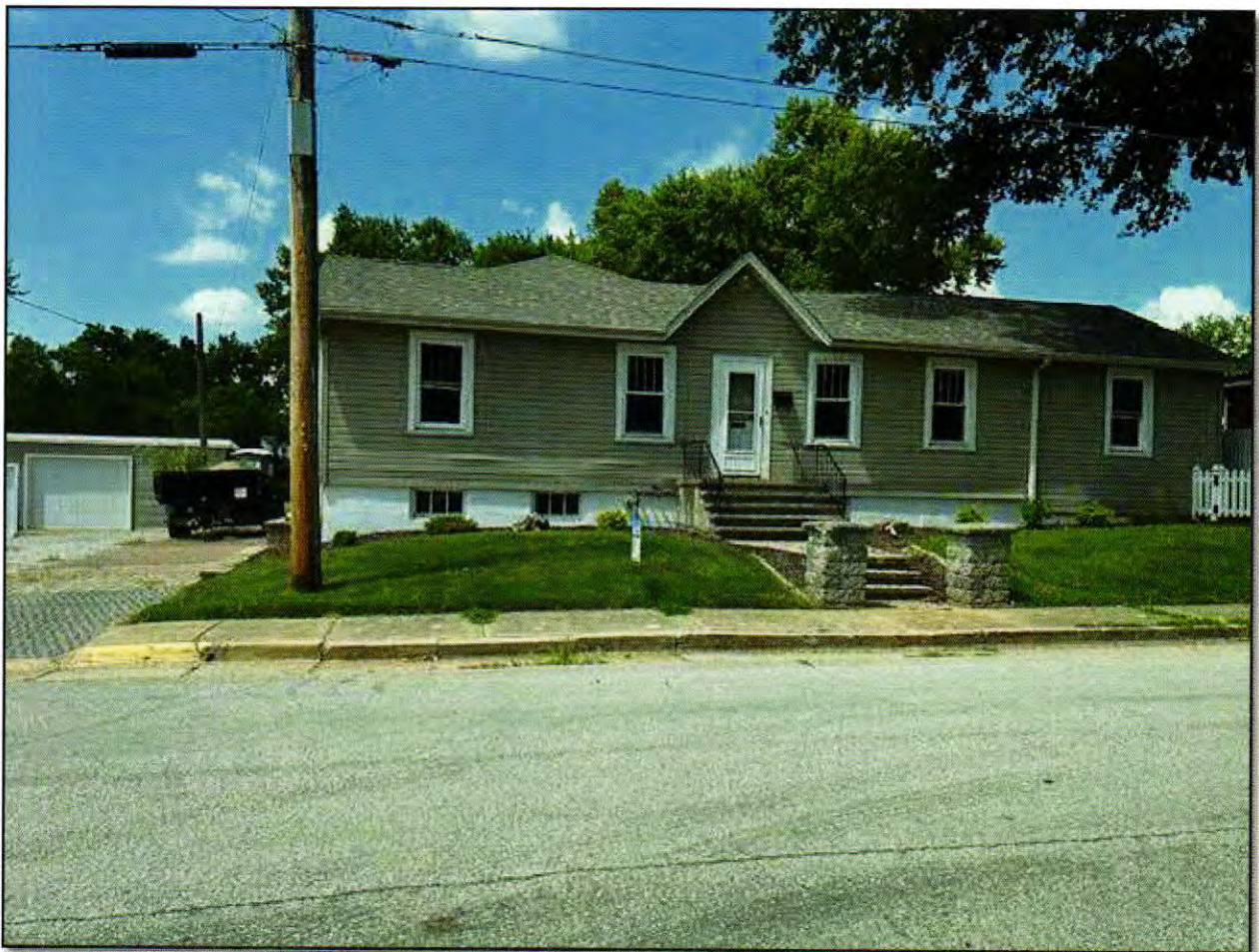
Figure 2: Street view of the Subject Property
