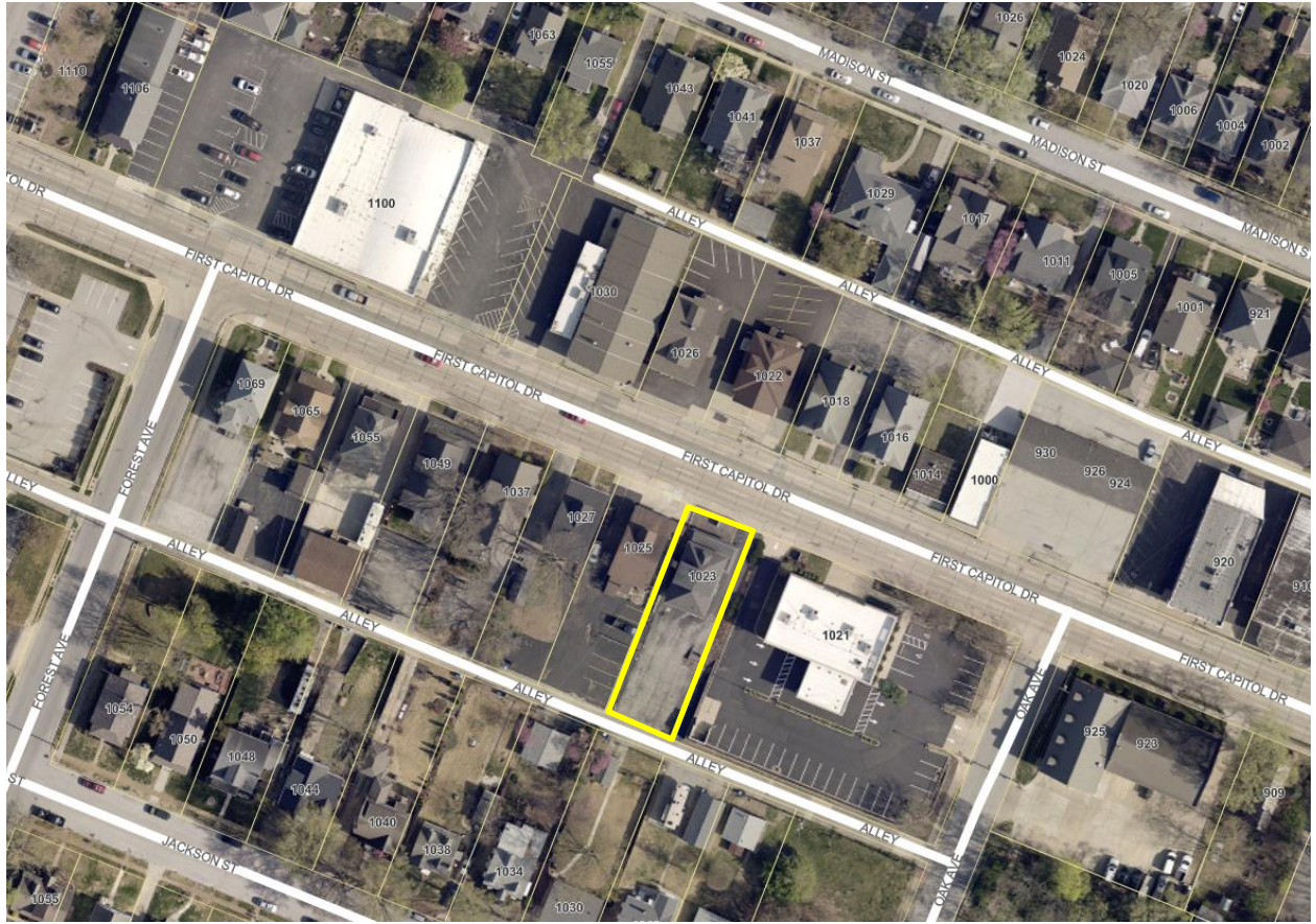
Figure 2: Aerial Photo of Subject Property
