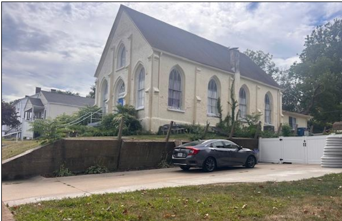
Figure 1: Location of retaining wall between properties.
