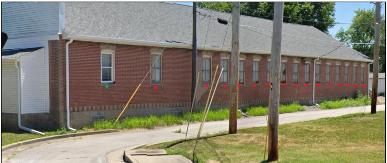
Figure 3: West façade windows to be covered shown with red dot, green to remain.
