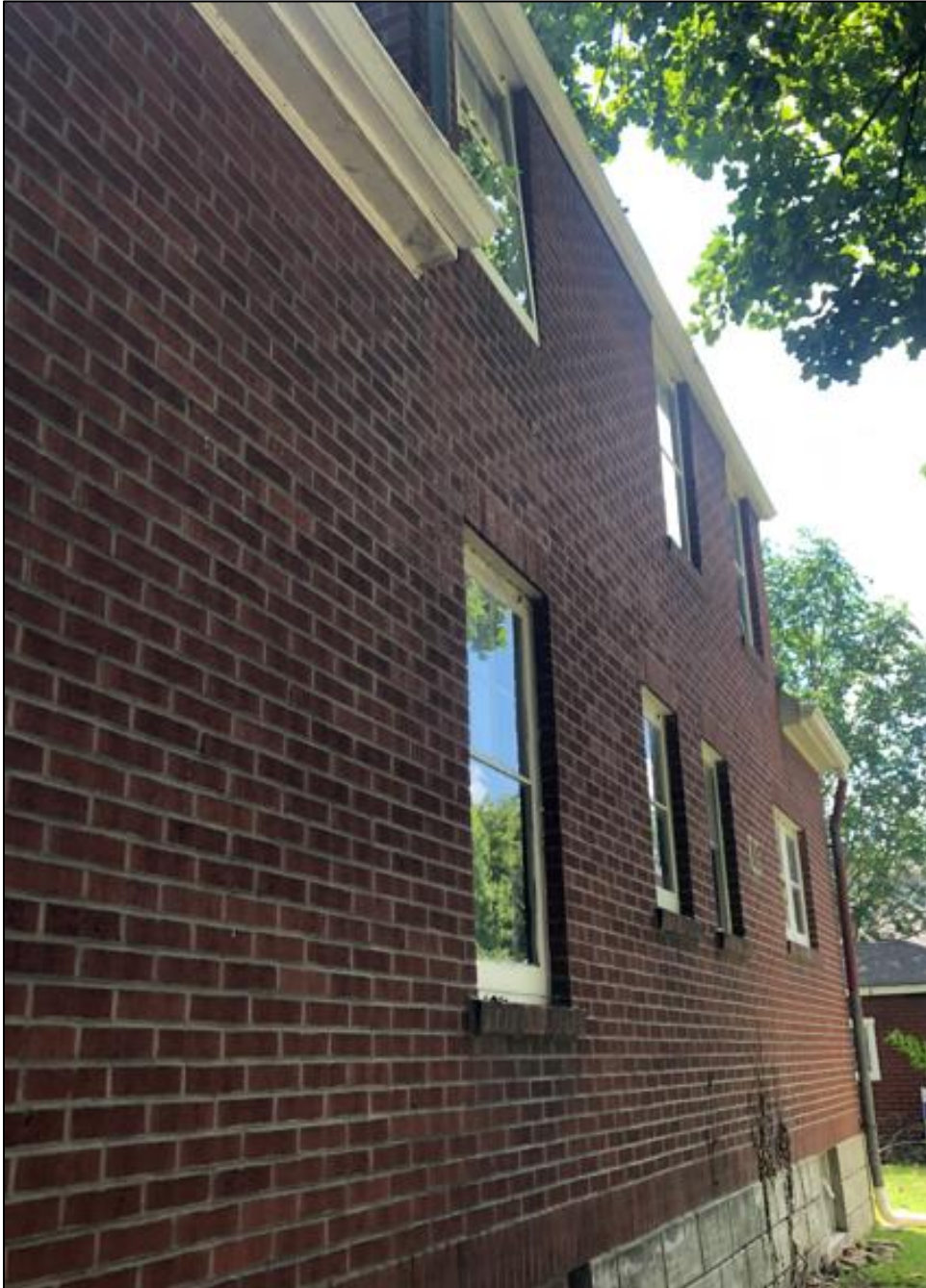
Figure 4: Rear façade currently.
