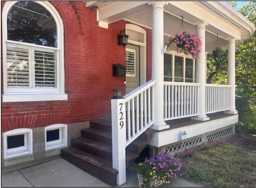
Figure 2: Existing steps condition and position.
