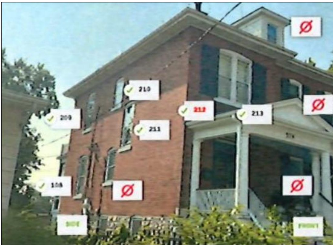
Figure 3: Subject windows for replacement.
