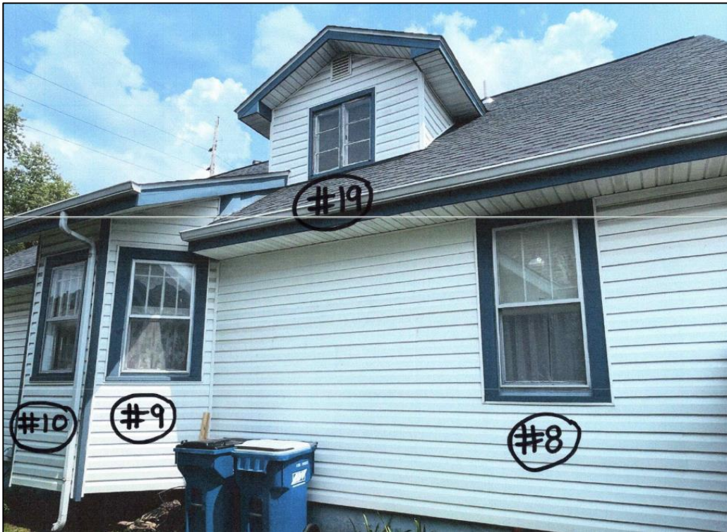
Figure 3: West elevation windows to be replaced.
