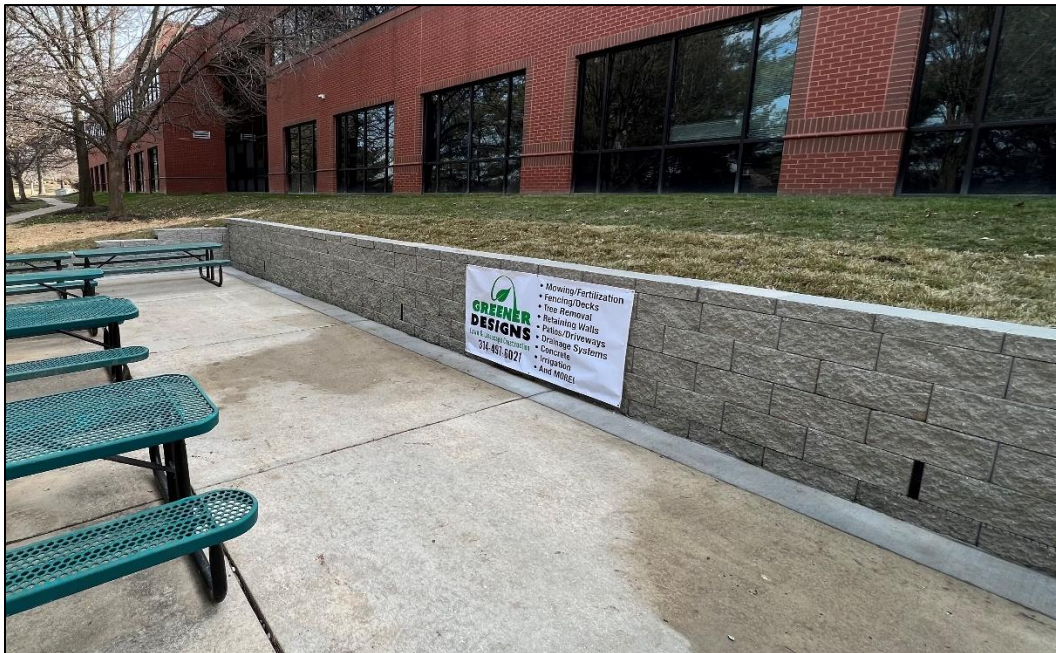
Figure 4: Retaining wall example.
