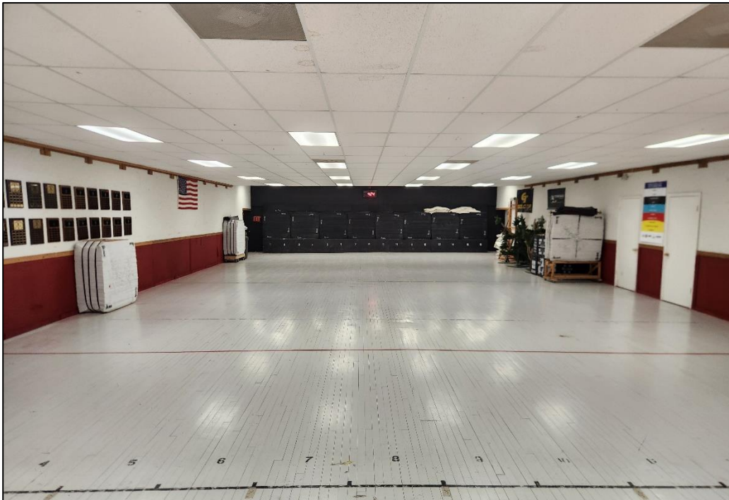
Figure 5: Interior photo showcasing windows covered by interior wall.
