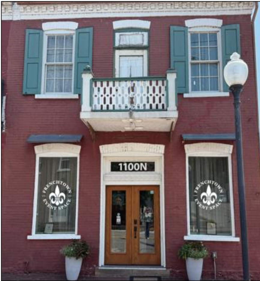
Figure 5: Proposed window signs (not to be utilized in this project due to surpassing allowed signage area).
