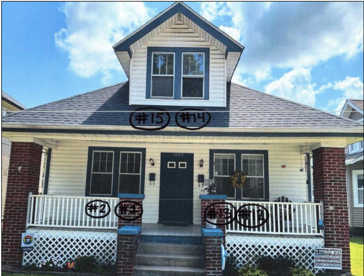
Figure 2: Front windows to be replaced on the dwelling.
