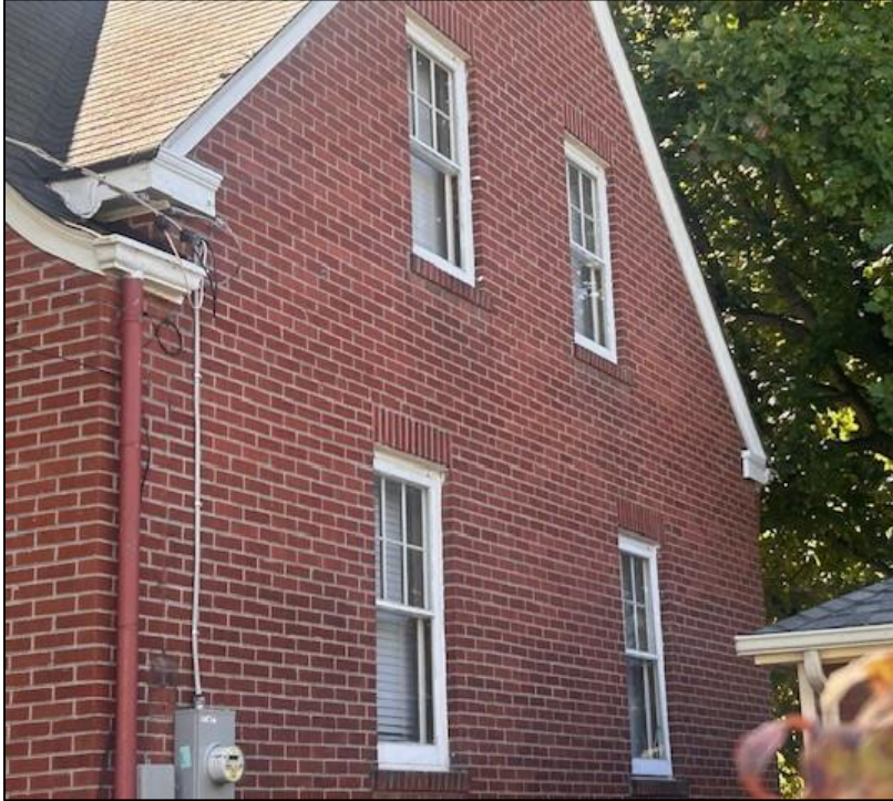
Figure 2: North façade windows as seen currently.
