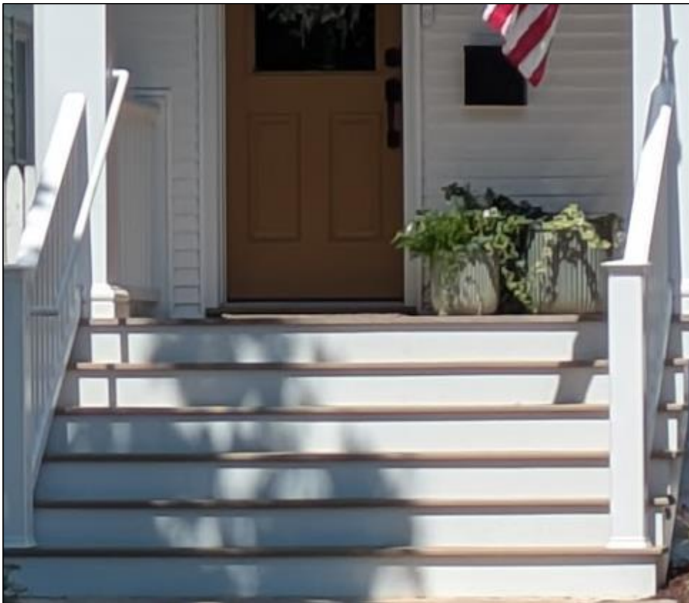
Figure 5: Steps example at 718 Clark Street.
