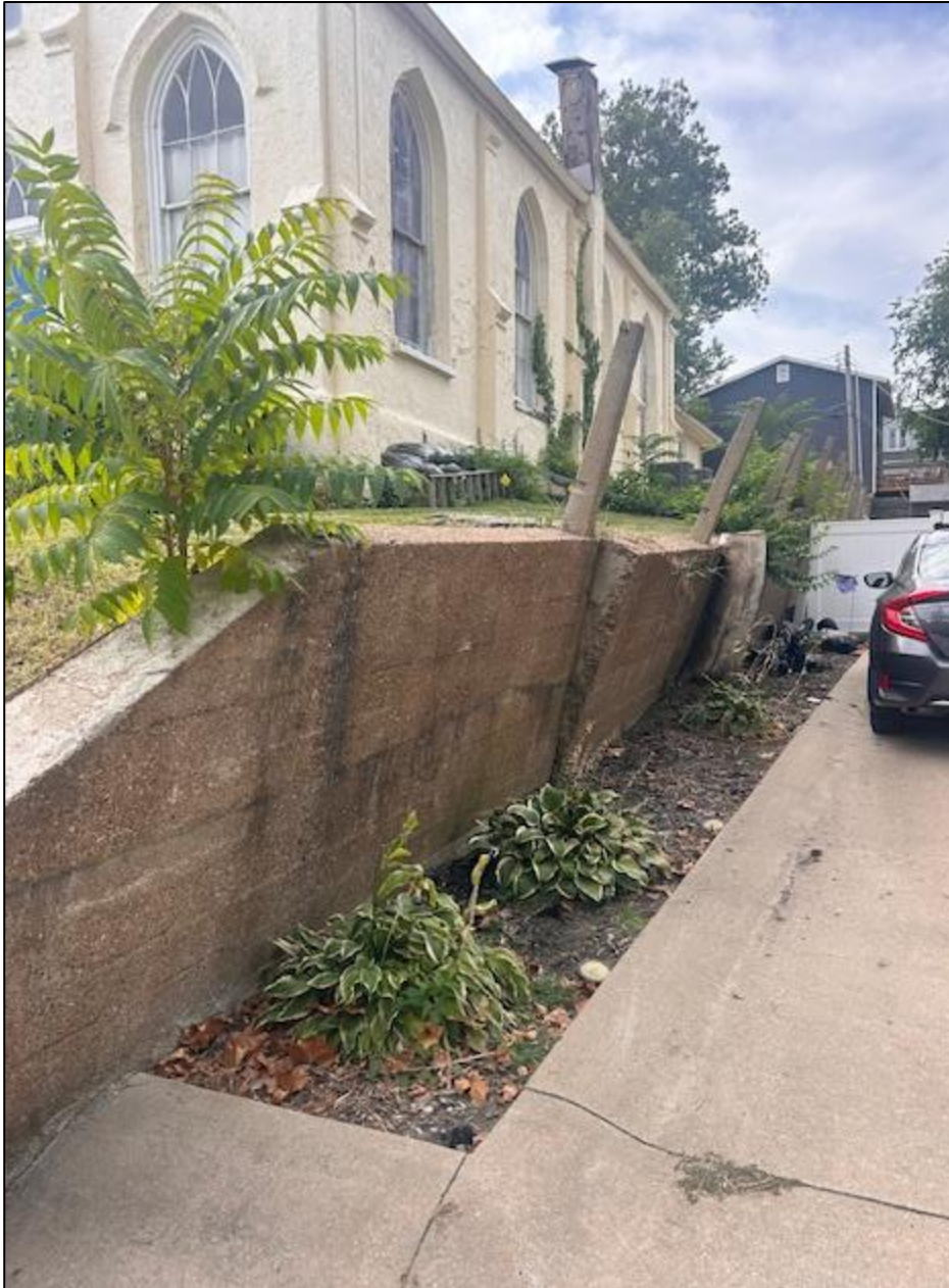
Figure 2: Retaining wall's current state.
