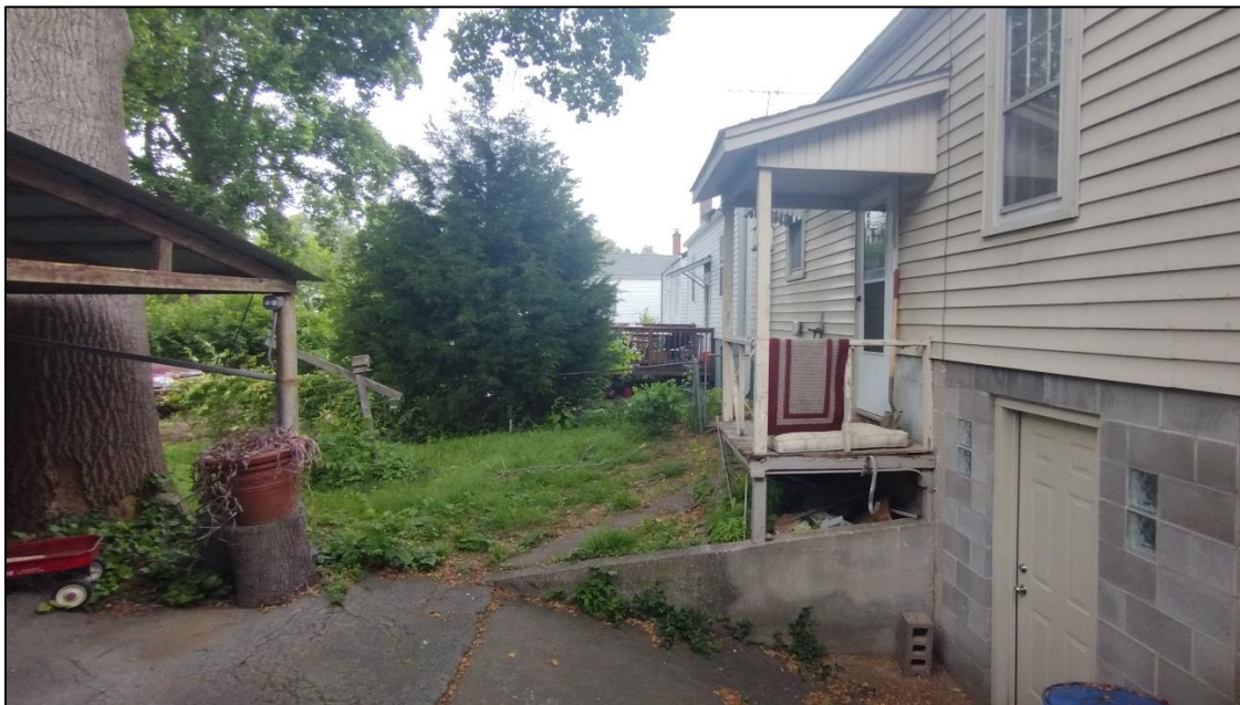
Figure 2: Existing rear yard showcasing existing deck and carport structure.
