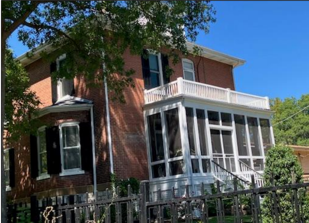
Figure 2: The rear façade of the property seen from Pike Street.
