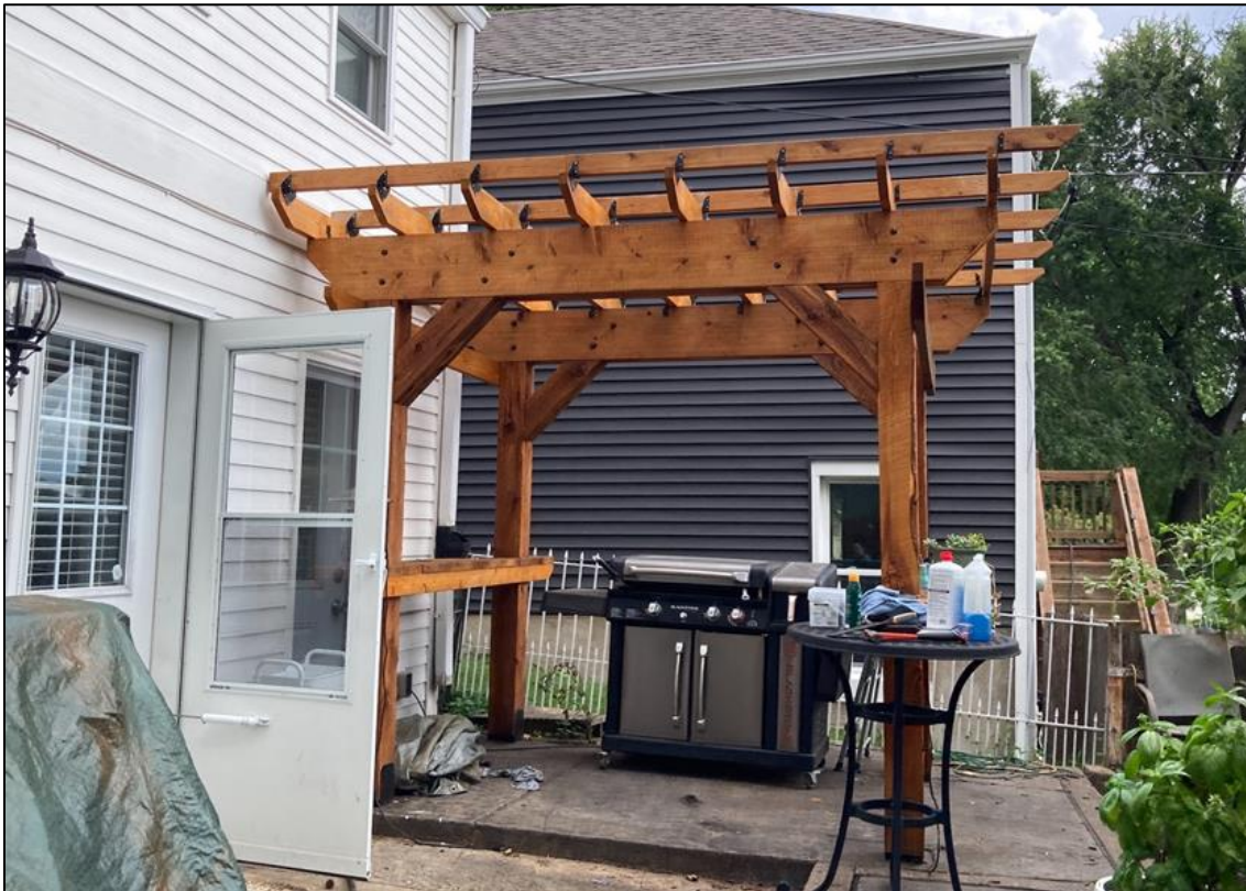
Figure 2: Subject after-the-fact pergola in the rear of property.
