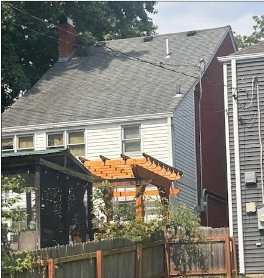
Figure 3: Pergola and additional accessory structure seen from alley
