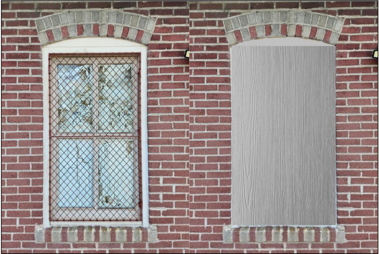
Figure 4: Example of existing v. proposed window opening.
