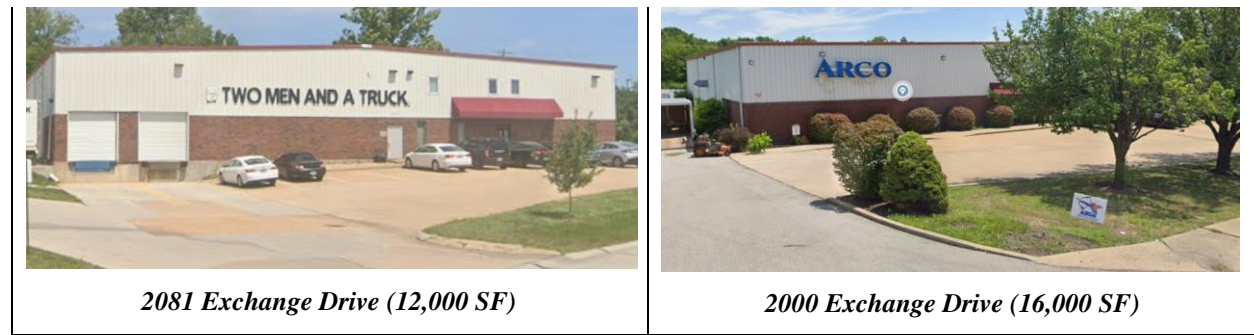
Figures 8-9: Surrounding buildings over 10,000 SF.
