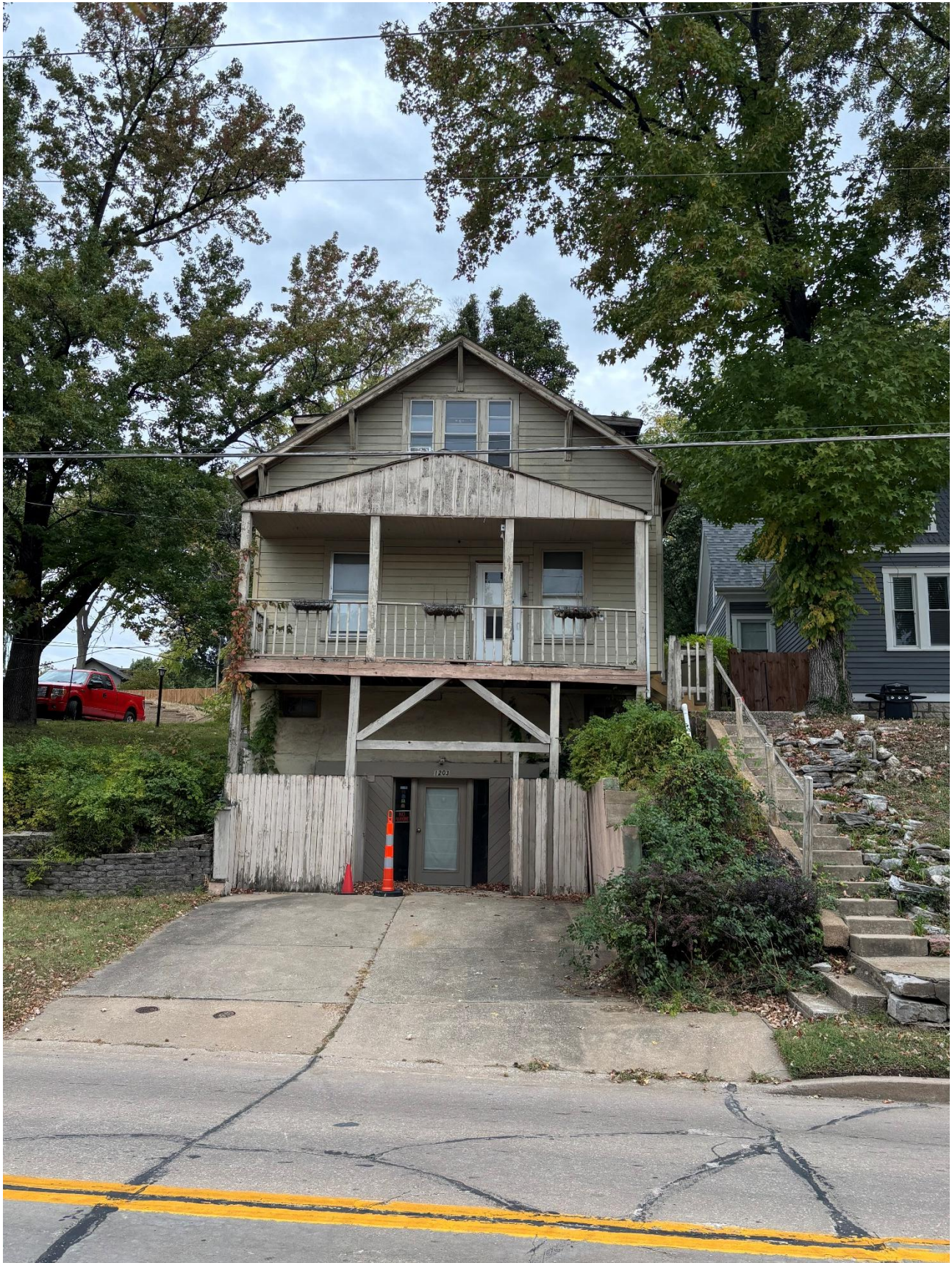
Existing Photo, Oct. 2025 – View From South Main Street, photo shows wood front porch/deck most likely not original to home construction. Alteration to the basement level to add storefront entry, also not original to home.
