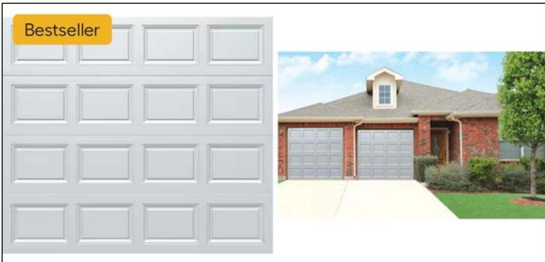
Figure 8: Garage door example.
