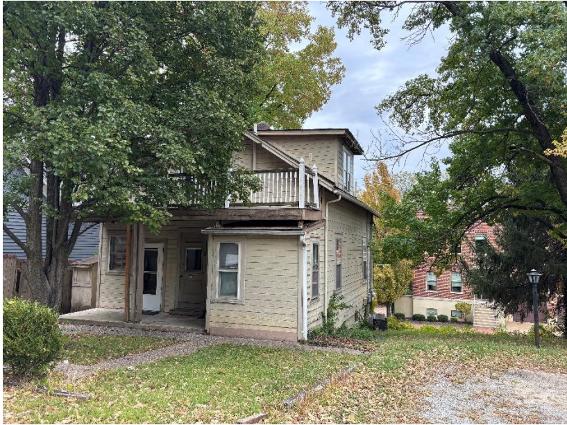
Existing Photo, Oct. 2025 – View from Rear & south side, photo shows rear addition to home
