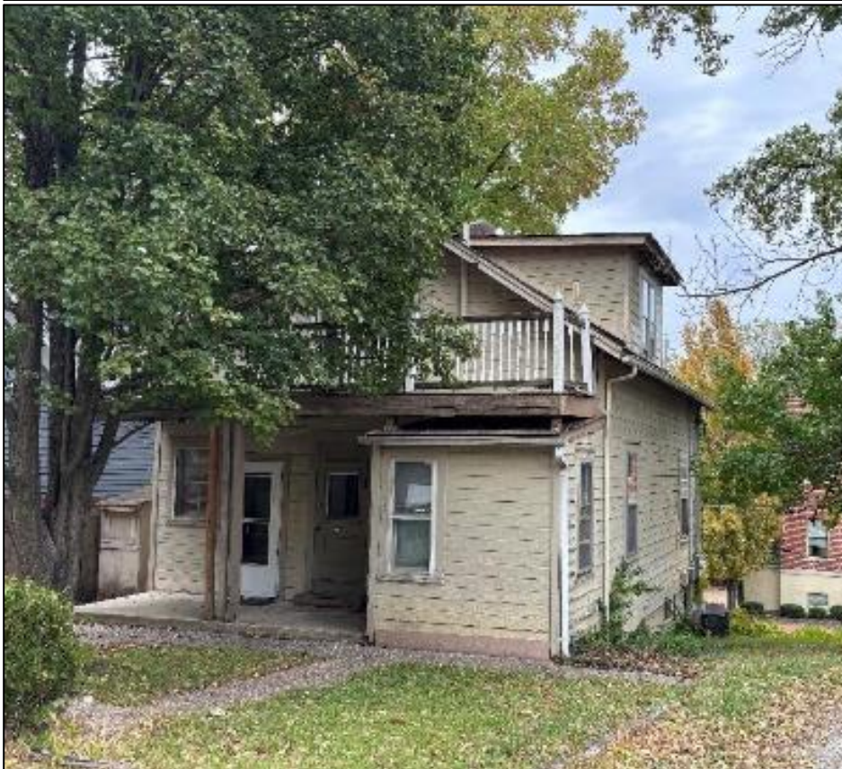
Figure 3: Rear of subject structure seen currently.
