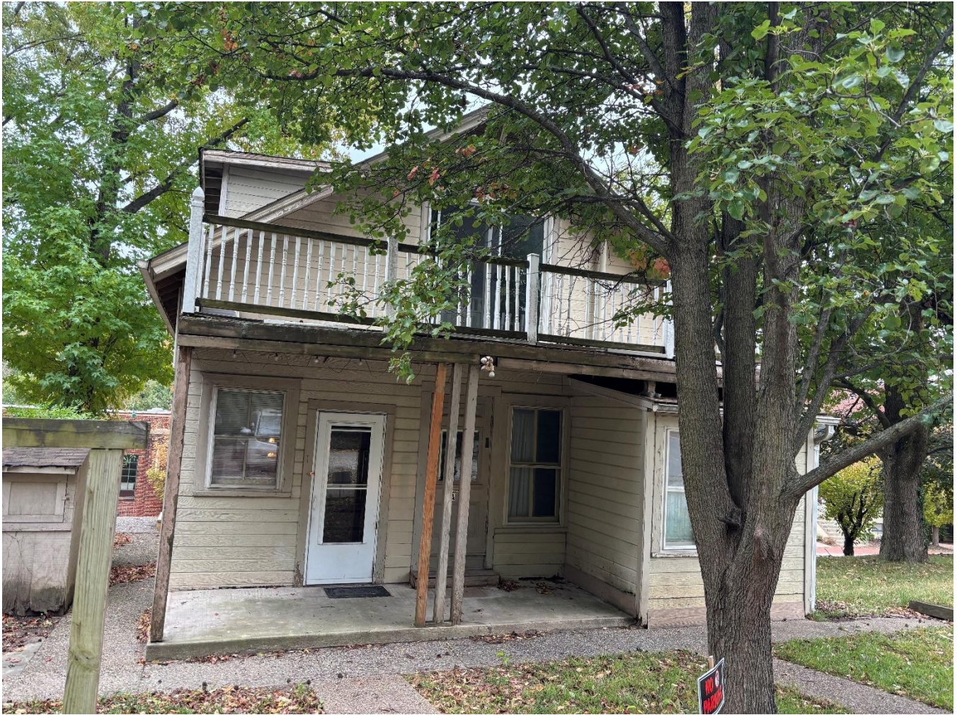
Existing Photo, Oct. 2025 – View from Rear, photo shows sliding glass door & upper-level deck, features that were most likely not original to the home. 2/2 wood windows at first level may be original.
