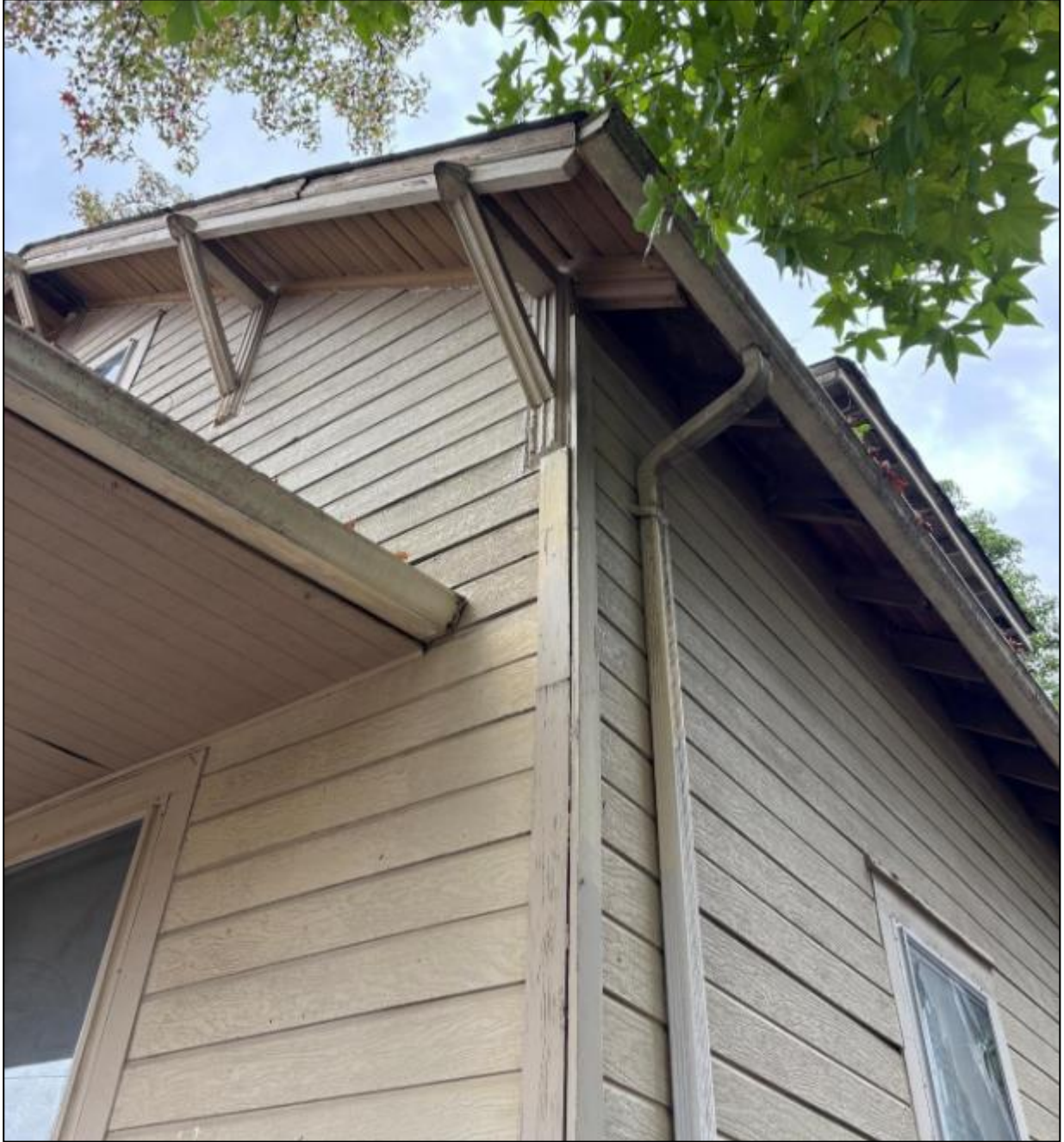
Figure 4: Existing photo detailing non-original siding & other non-original details.
