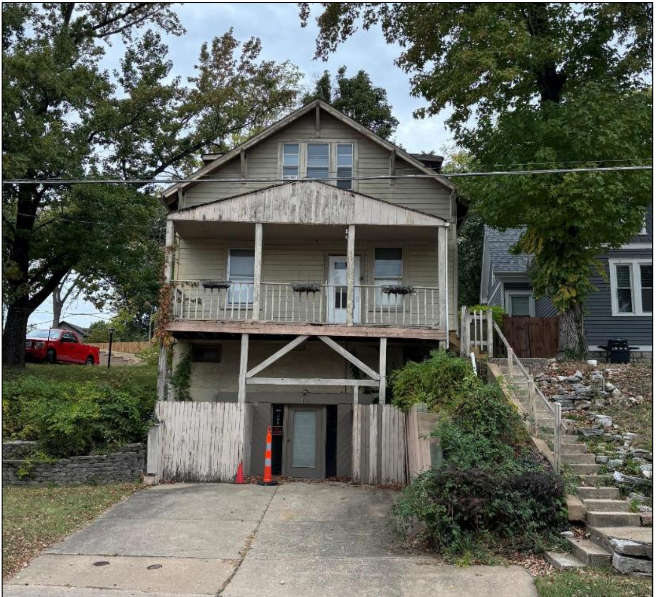
Figure 2: Subject structure seen from South Main Street currently.
