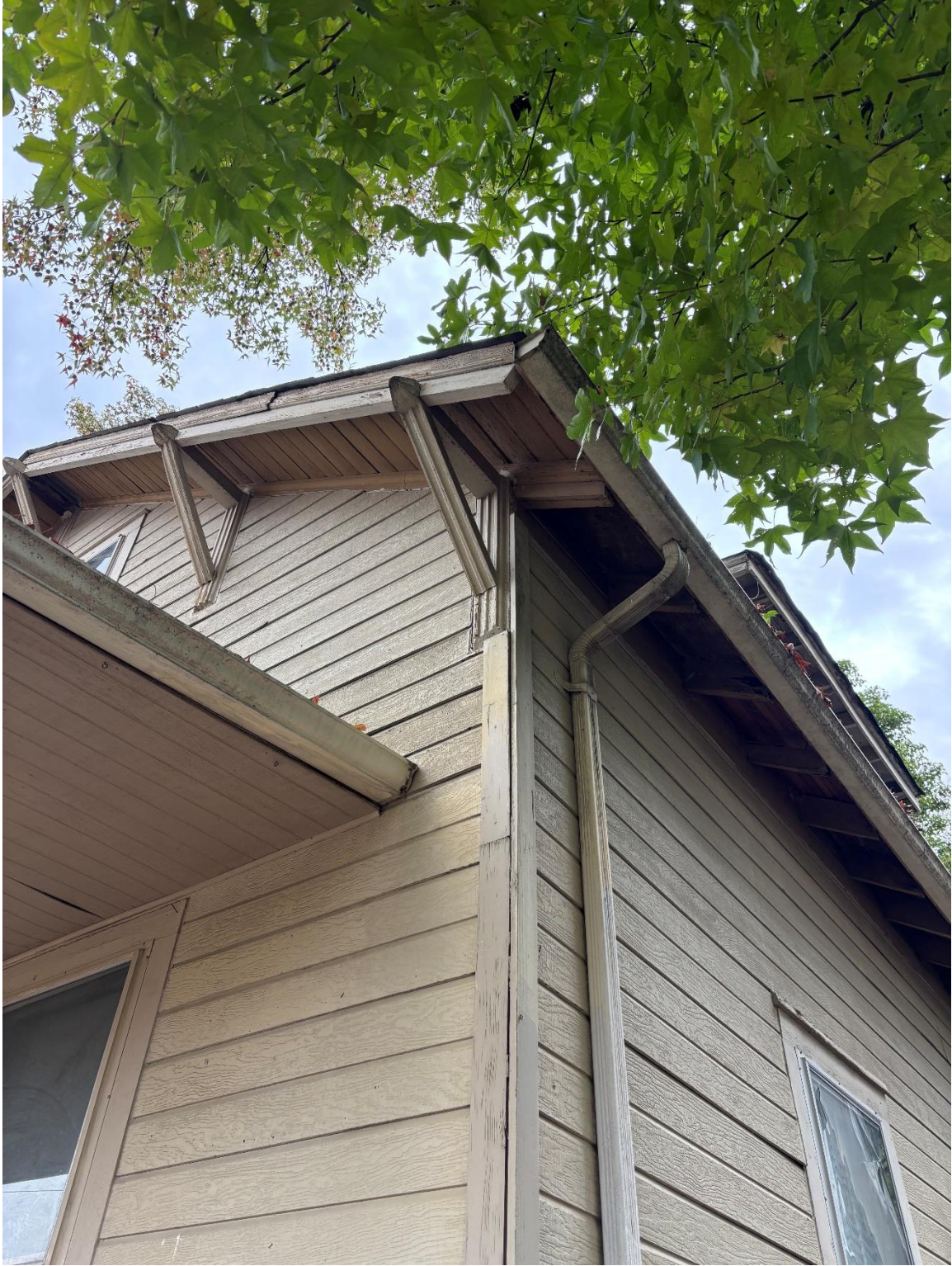
Existing Photo, Oct. 2025 - detail showing wood grain siding (not original to home), decorative gable braces & exposed rafter tails (most likely original to home construction)
