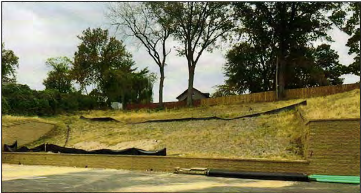
Figure 3: Existing conditions of the subject property.
