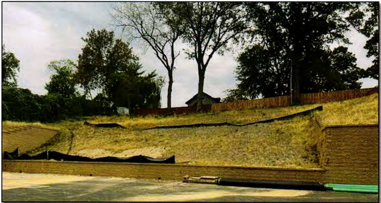
Figure 3: Existing conditions of the subject property.
