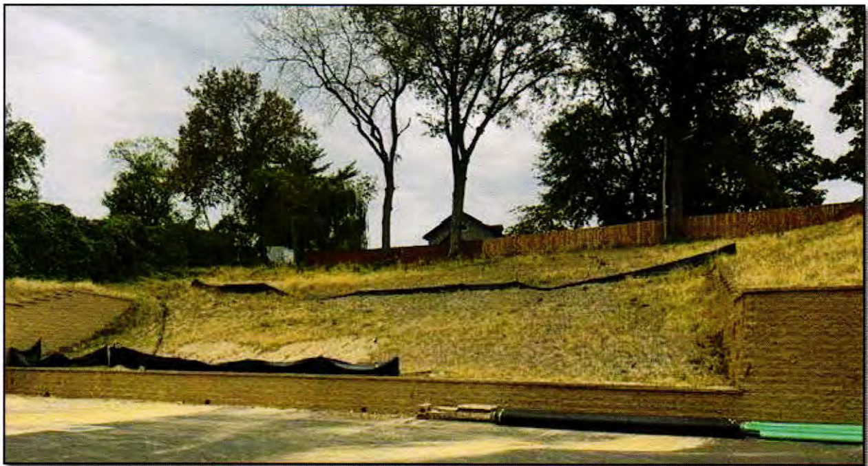
Figure 3: Existing conditions of the subject property.
