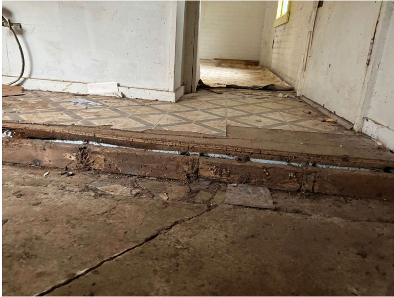
Interior Conditions - B
