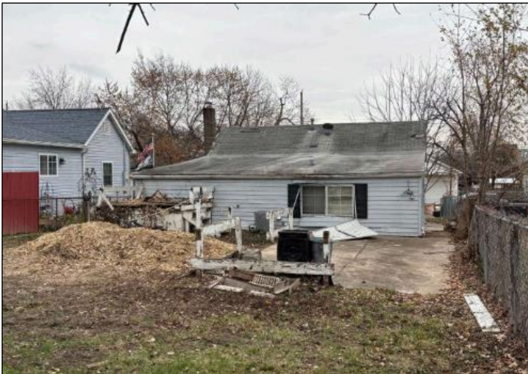
Figure 3: Rear view of subject dwelling.
