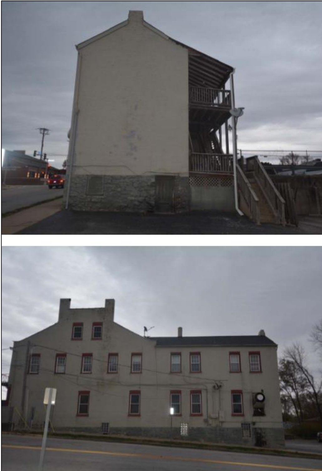
Figure 2: Existing south and west elevation of the structure.
