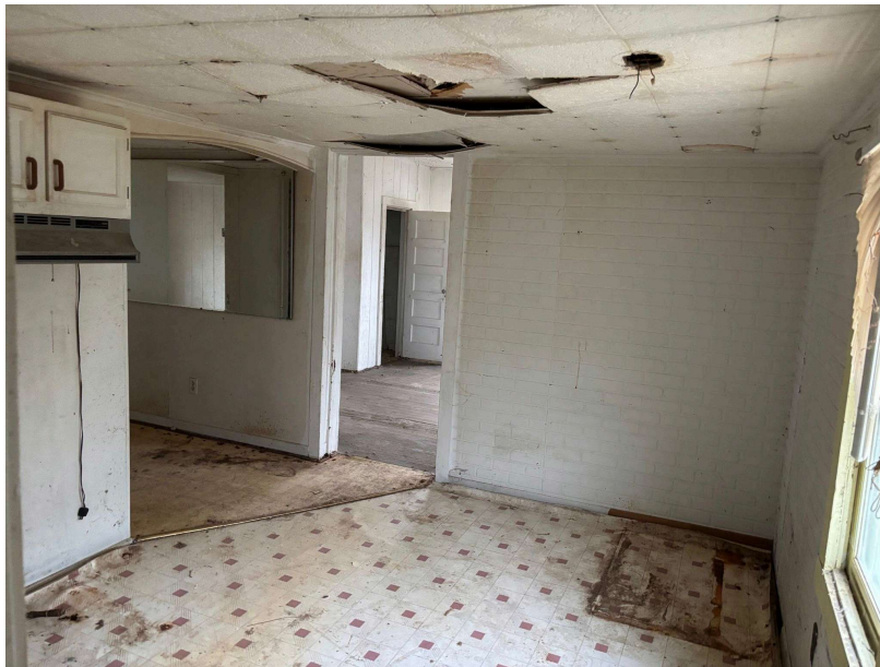
Interior Conditions - A
