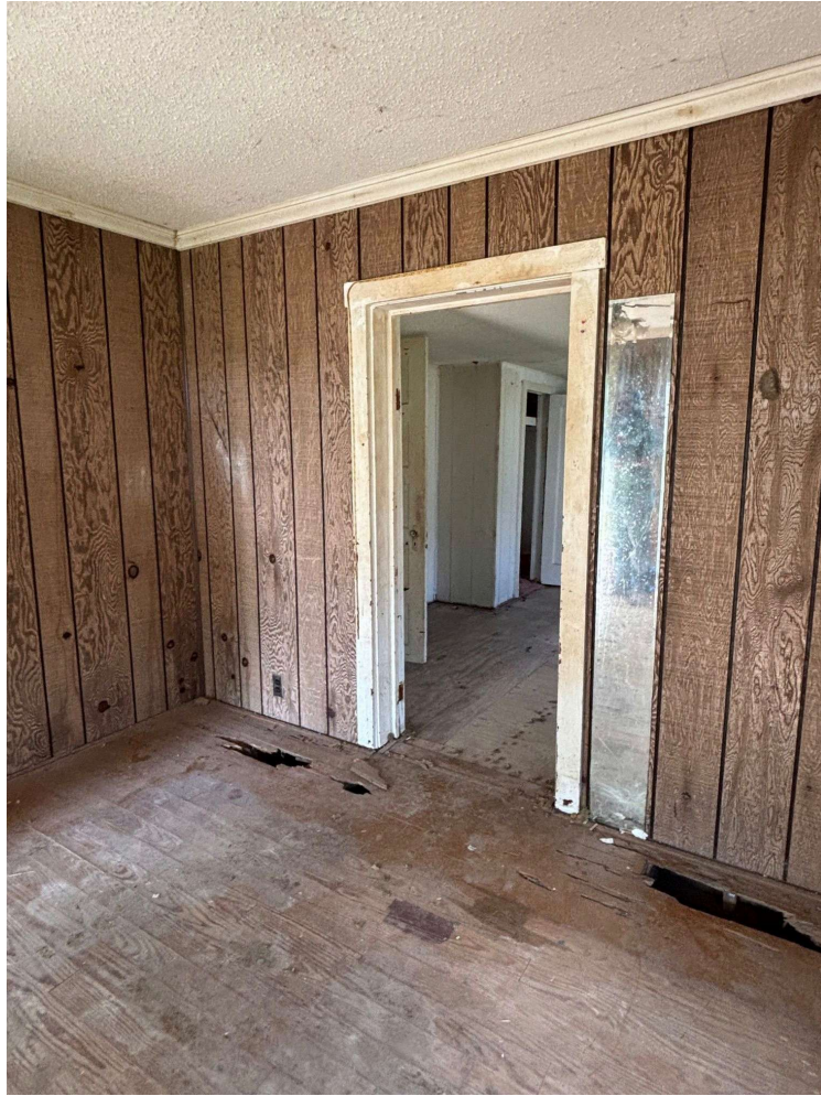
Interior Conditions - D
