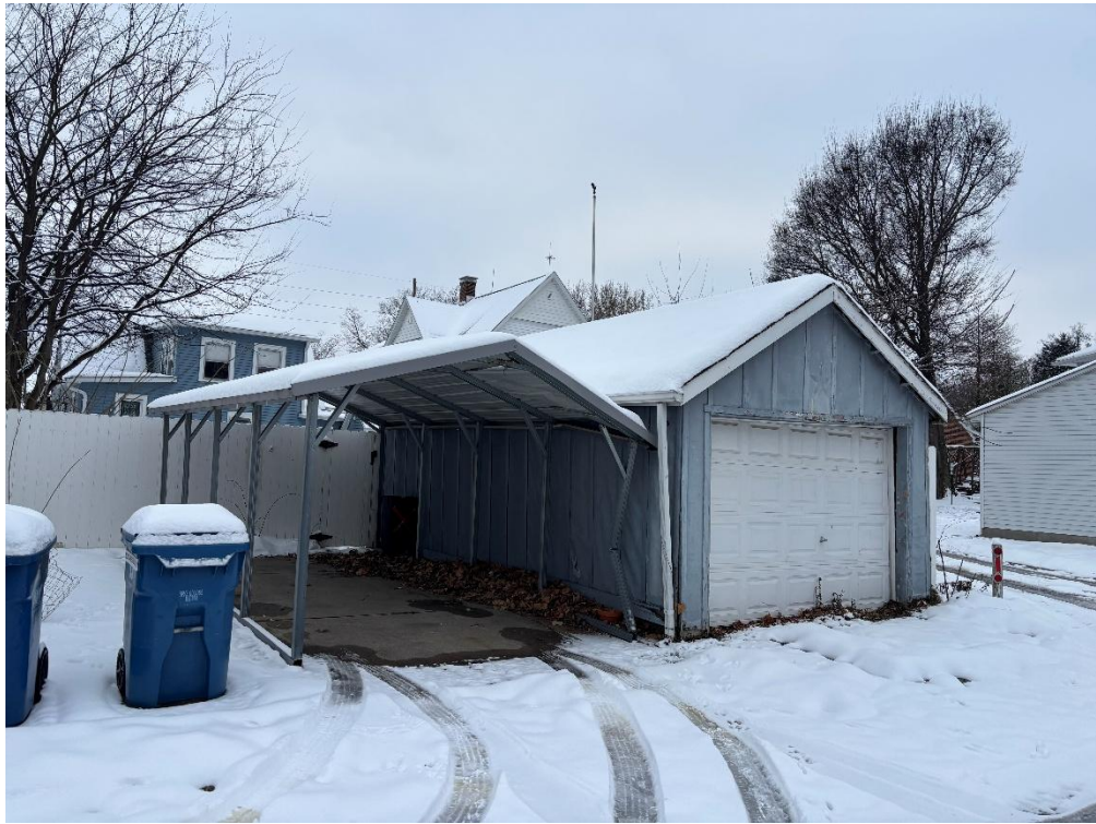
Existing Photo, Dec. 2025 – Garage View from Alley 2
