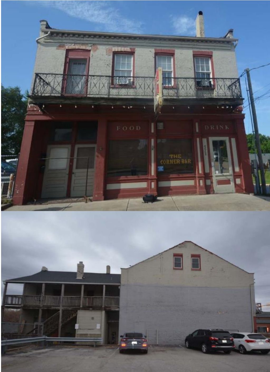
Figure 1: Existing north and east elevation of the structure.
