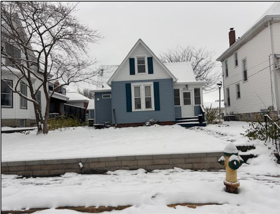
Figure 1: Subject property seen from Madison Street.
