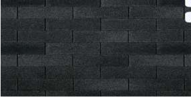
Figure 4: Roof material example.
