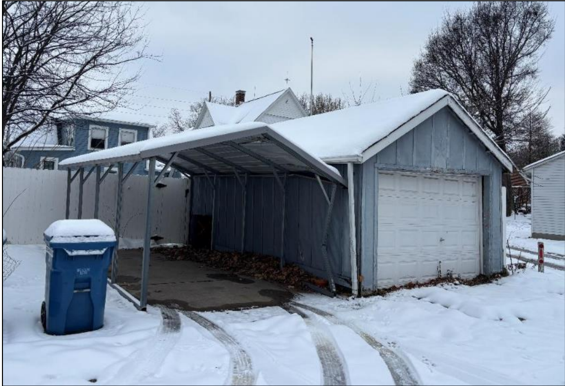
Figure 3: Additional photograph of subject structures.
