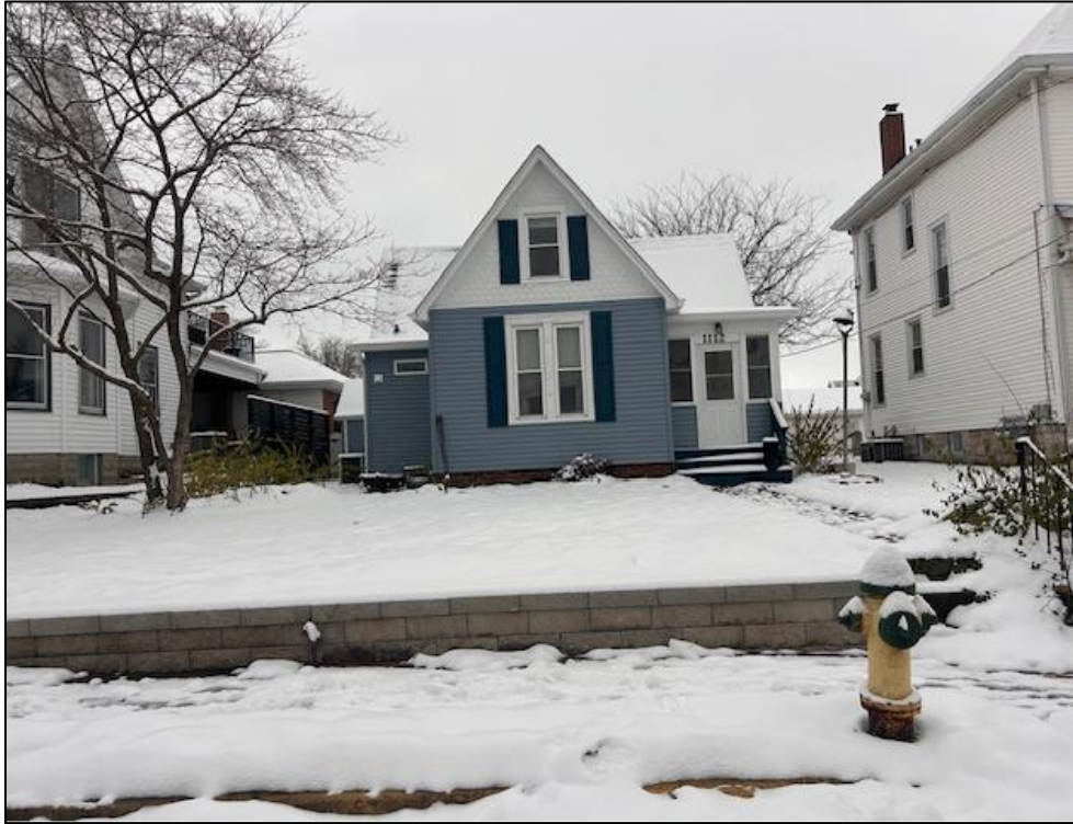
Figure 1: Primary structure on the subject property.
