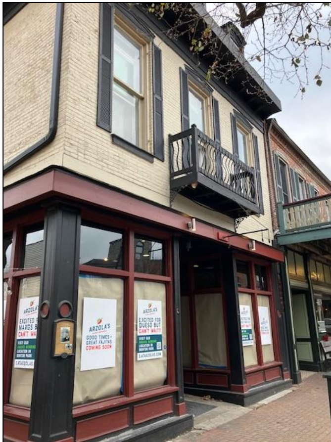
Figure 2: Current Front Façade.
