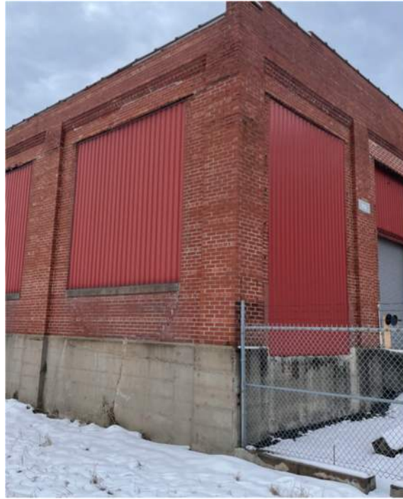
Image 6: Northern Section Eastern Stem Wall Construction
