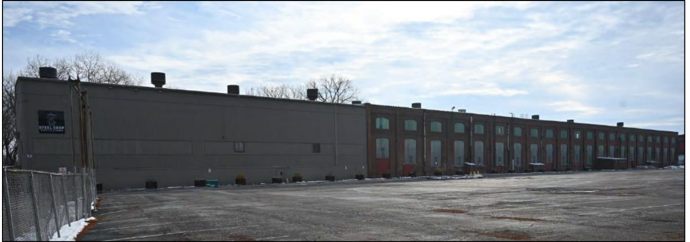
Figure 2: Building 90 seen from North 2 nd Street (grey area is the 1954 addition).
