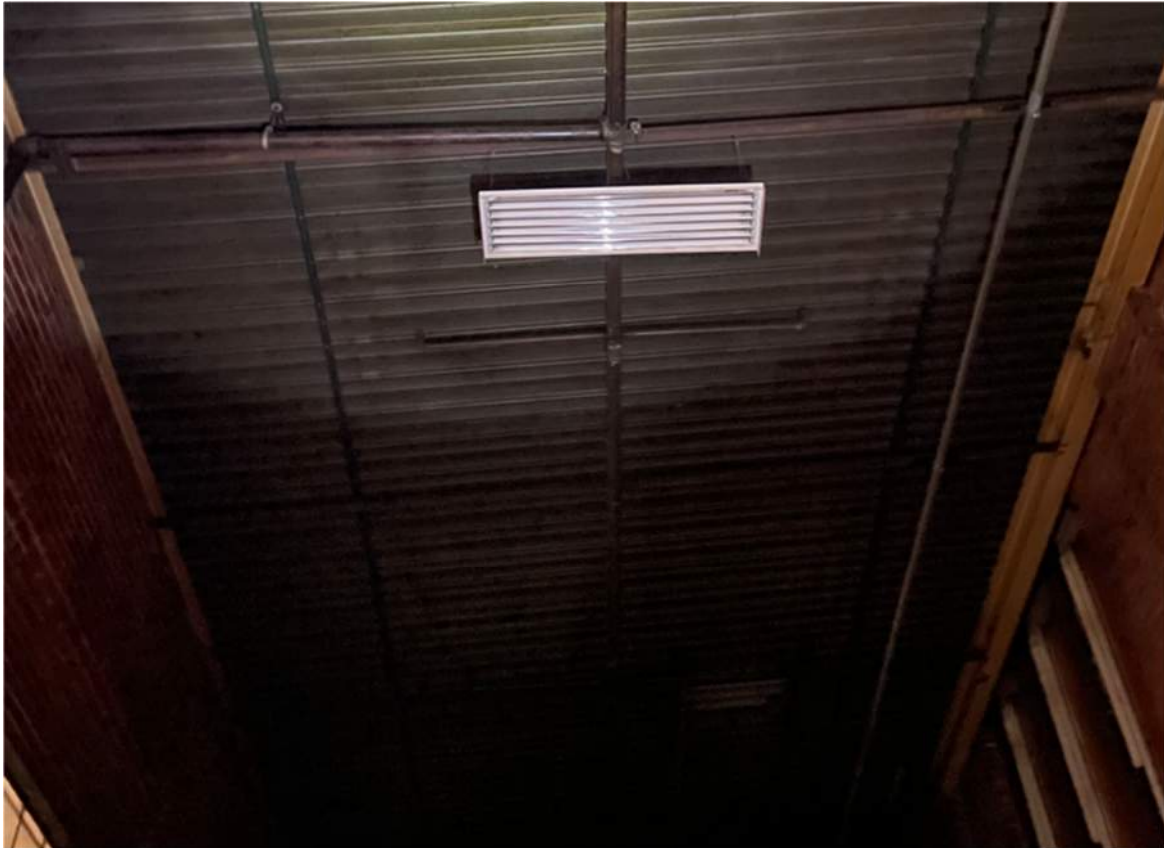
Image 8: Northern Infill Area Metal Deck Roof Between Existing Buildings.
