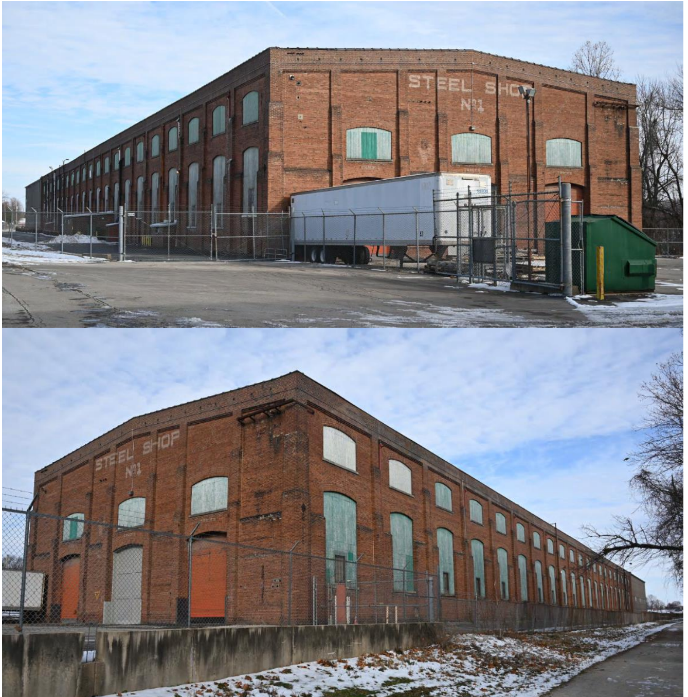
Figure 1: Building 90 seen presently (looking north).
