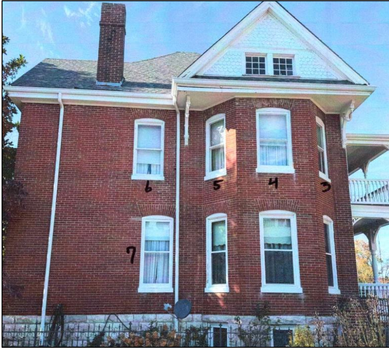
Figure 3: Windows #3 through #7 for replacement.
