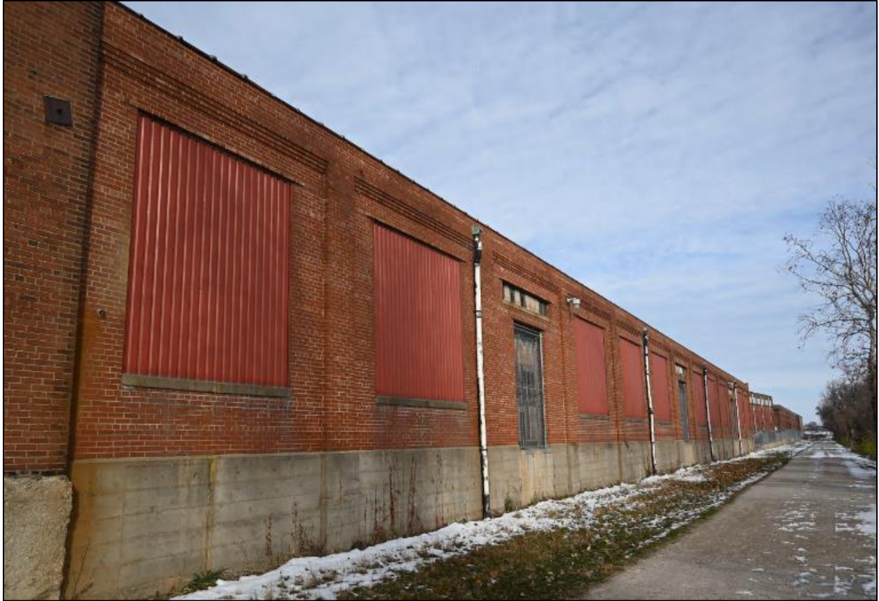
Figure 5: Northern portion of Building 91a to remain (seen from KATY Trail).
