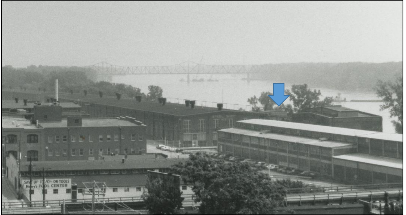
Figure 7: Historic photograph featuring the roof of 91A
