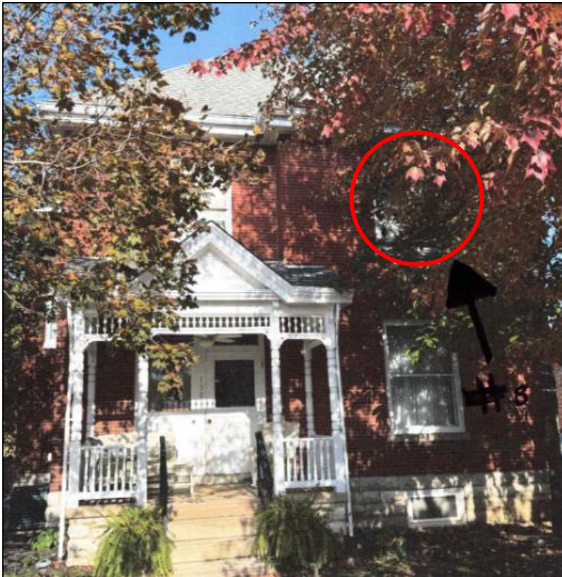
Figure 4: Windows #8 for replacement.
