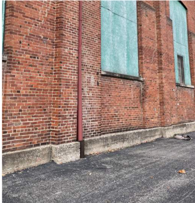
Image 3: Typical Foundation Stem Wall Construction of Southern Building Section
