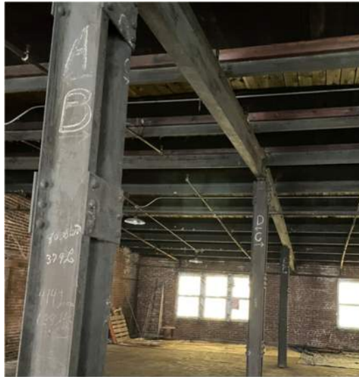
Image 3: Southern Section Roof Framing
