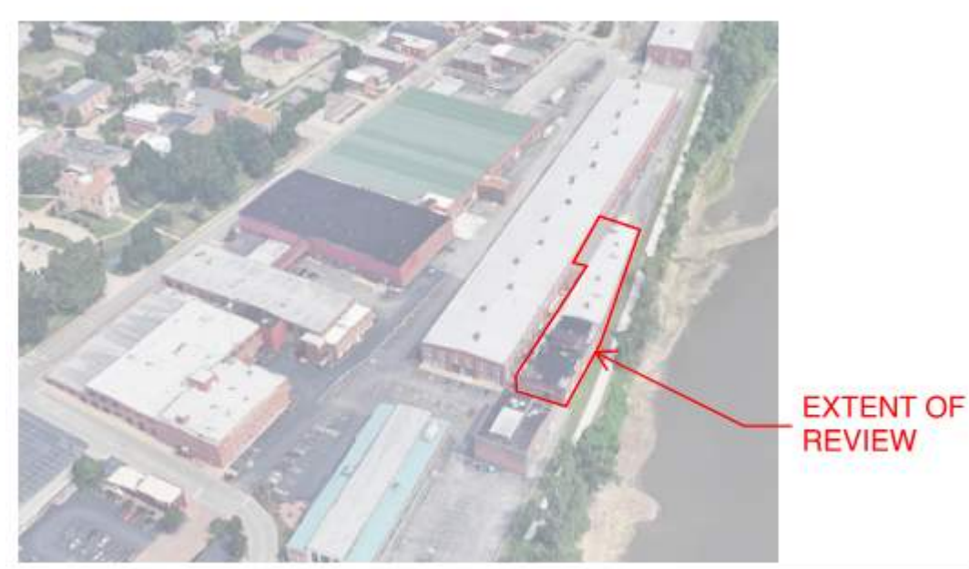
Image 1: Extent of Assessment Review
