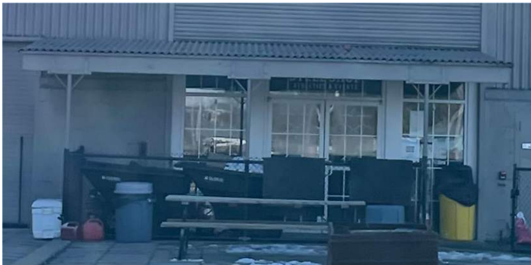
Image 8: North Entrance Canopy
