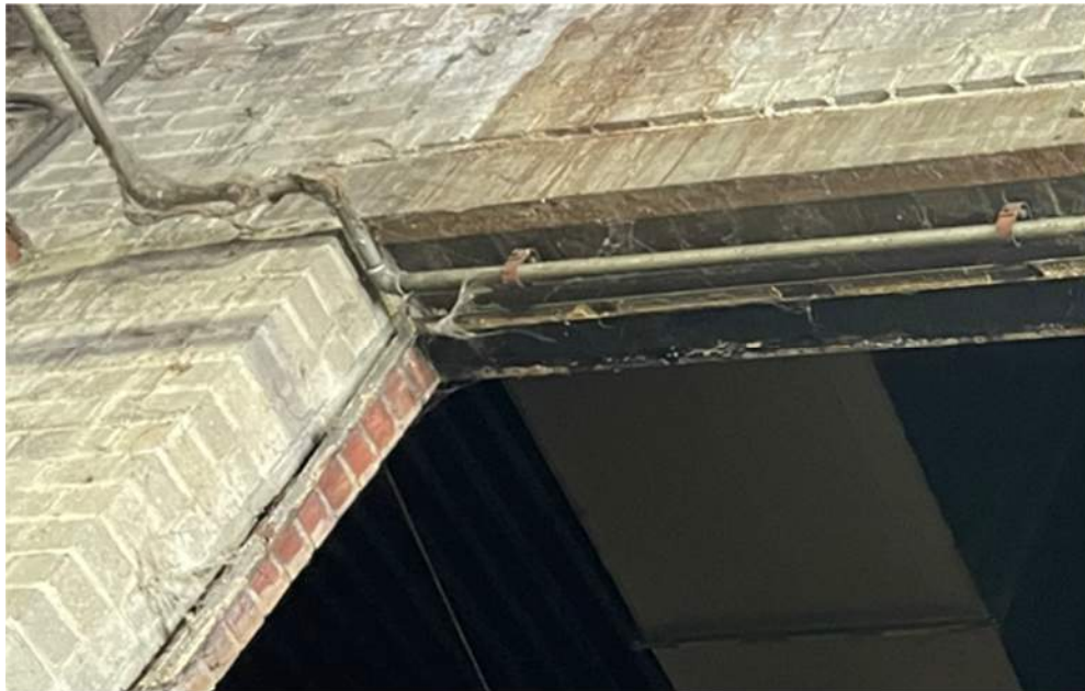
Image 7: Northern Section Wall Opening Lintel
