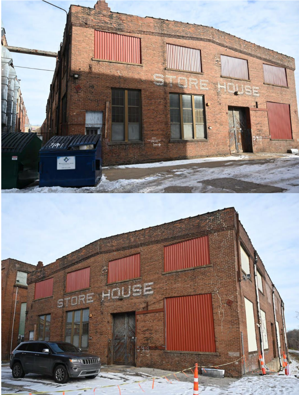
Figure 1: Building 91A “Store House” seen presently (looking north).
