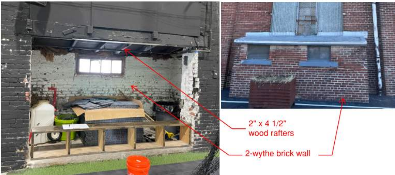
Image 5: Southern Building Western Shed Construction
