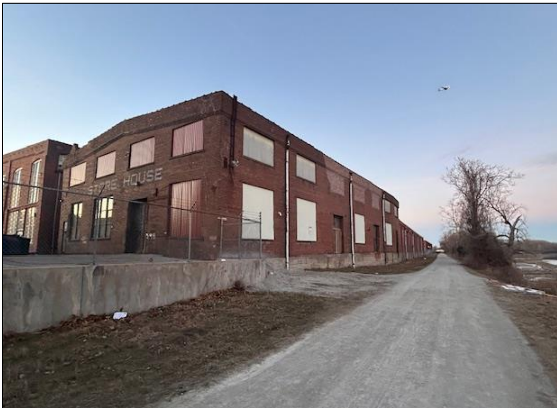
Figure 8: Additional photo of subject structure from KATY Trail (looking north).
