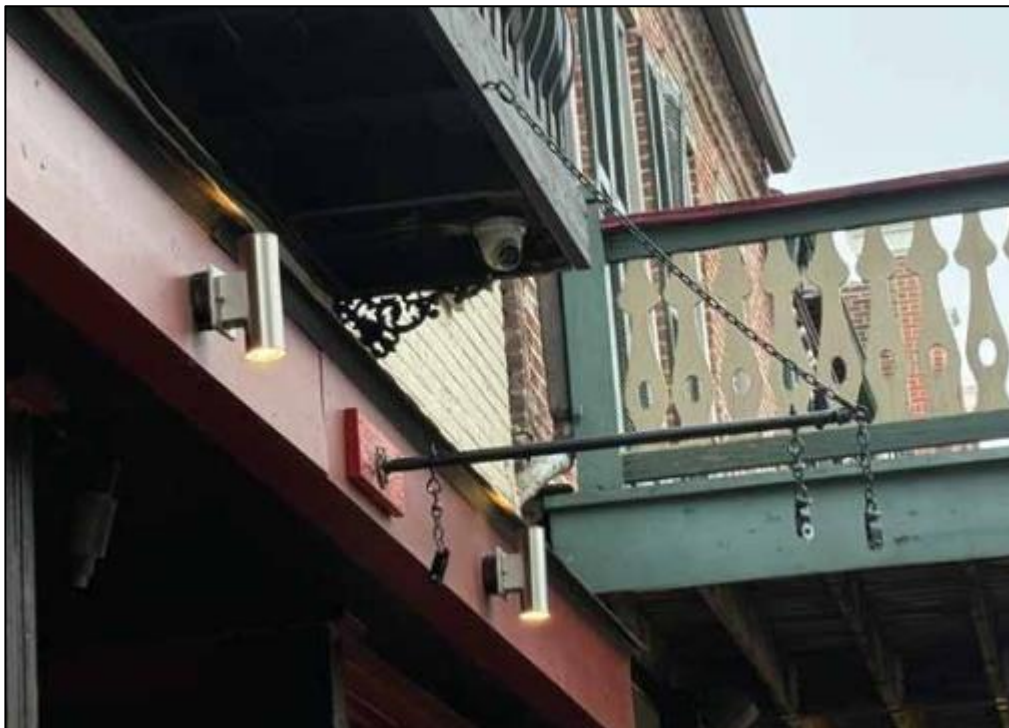
Figure 3: Existing black bracket and chains.
