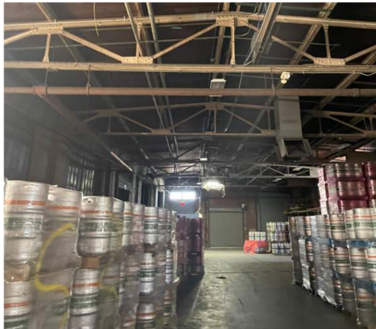
Image 5: Northern Section Roof Framing
