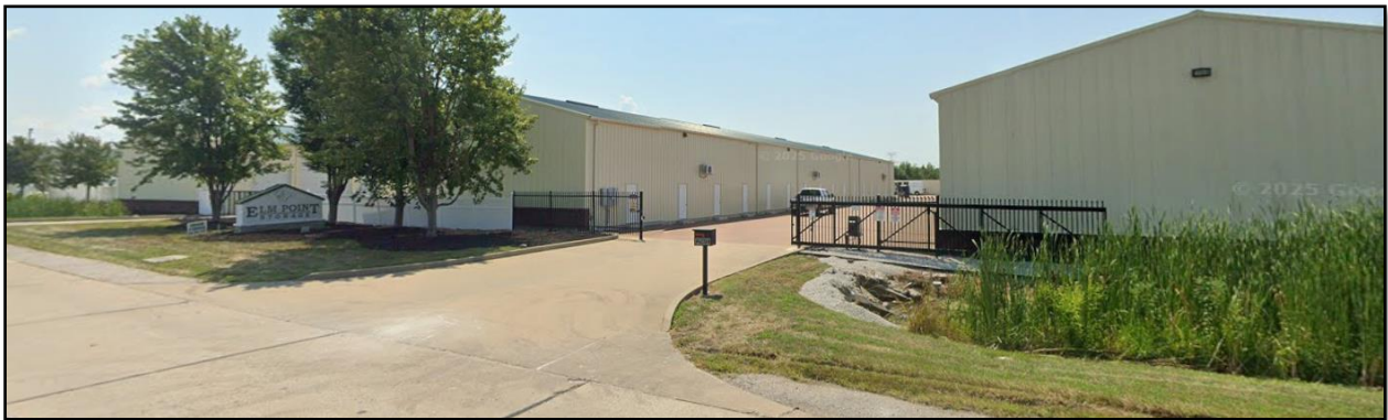
Figure 4: 2901 Elm Point Industrial Drive
