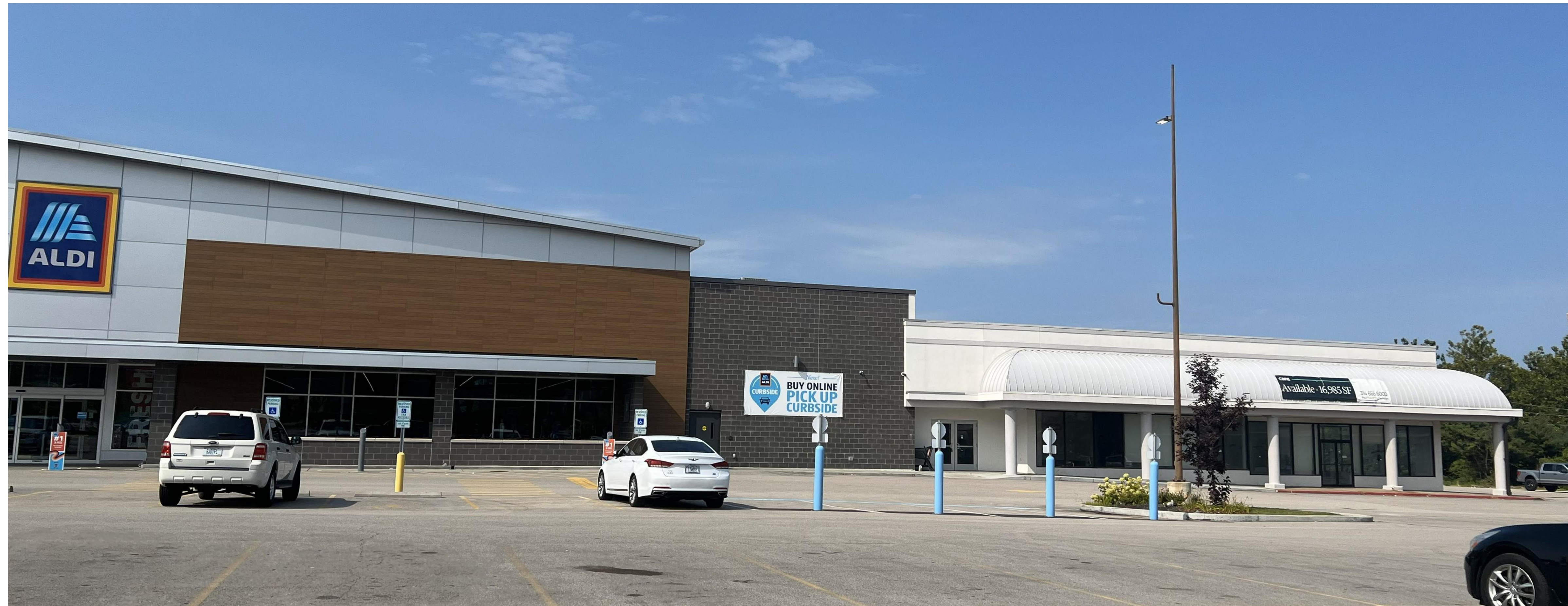
2 | EXISTING CONDITION PHOTO PZ-1 | NOT TO SCALE
