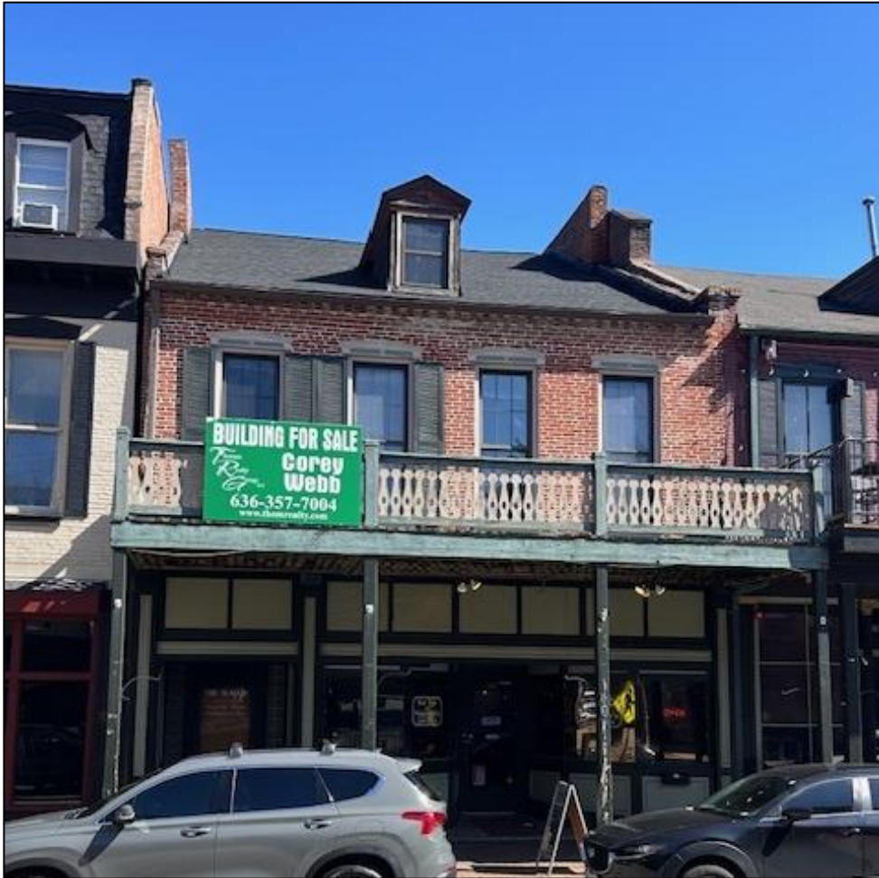
Figure 1: Building seen currently from Main Street.
