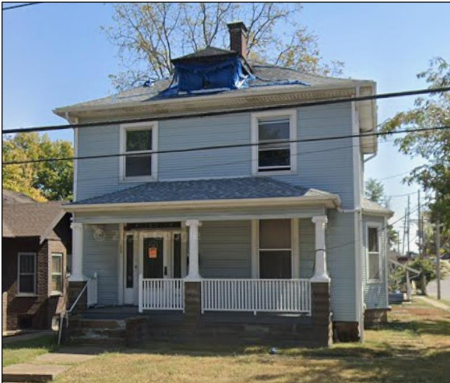
Figure 1: Subject structure seen before rehabilitation.
