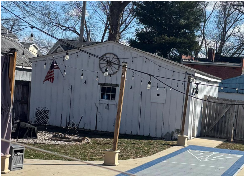
Existing Photo, Feb. 2026 – Garage View from rear yard
