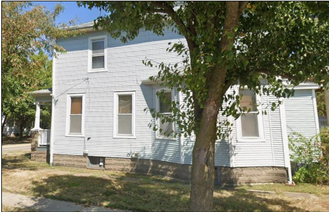
Figure 2: Windows on Monroe Street side previously.
