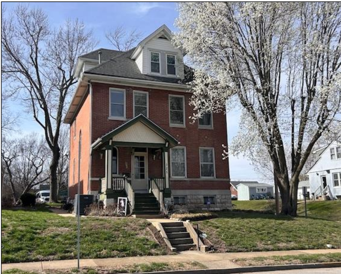
Figure 1: 725 North 4 th Street seen presently.
