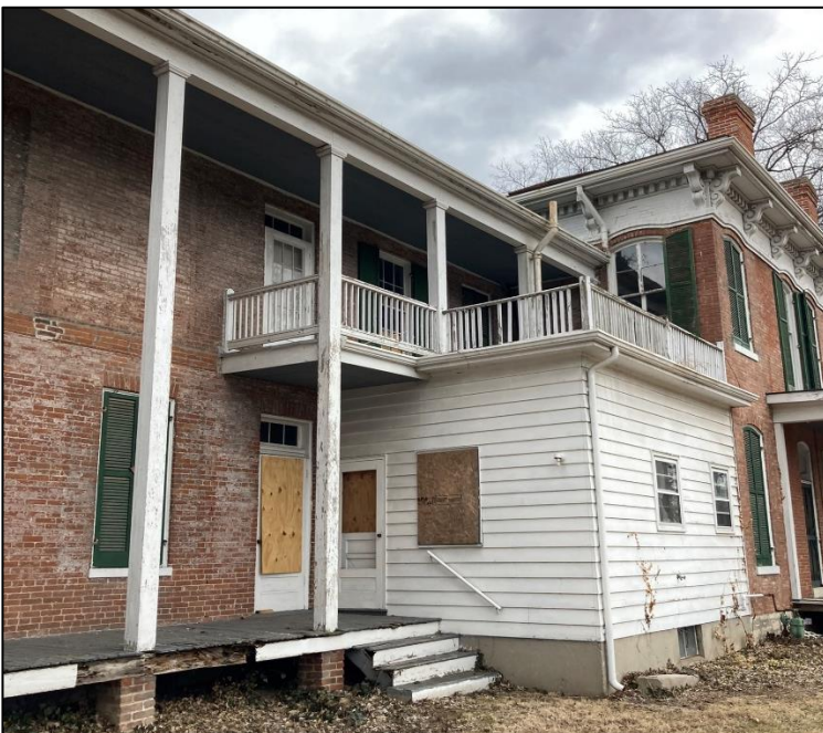
Figure 3: Frame addition on south elevation.
