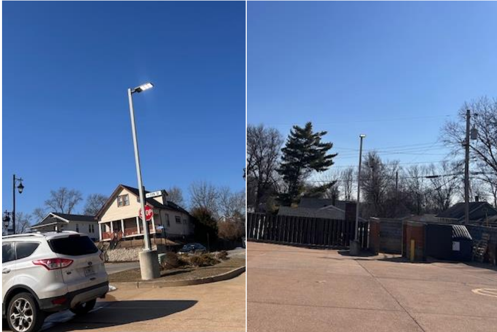
Figure 3: Two parking light poles on south side of structure.
