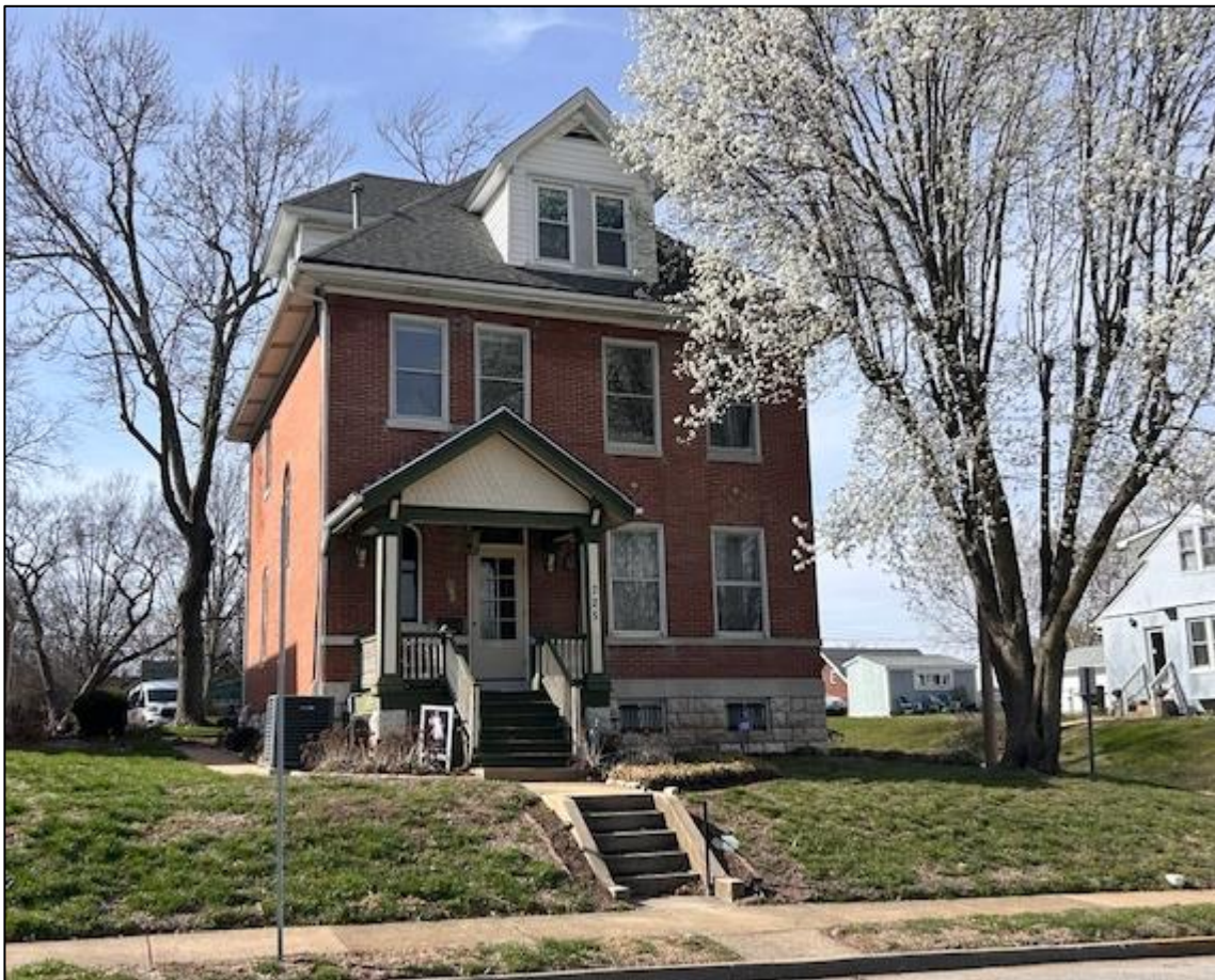
Figure 1: 725 North 4 th Street seen presently.
