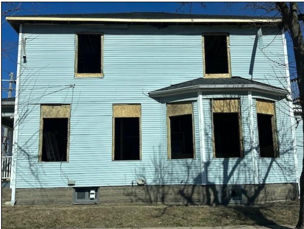
Figure 3: Window openings being altered.
