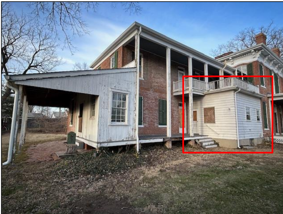
Figure 1: South elevation showcasing 1978 frame addition.
