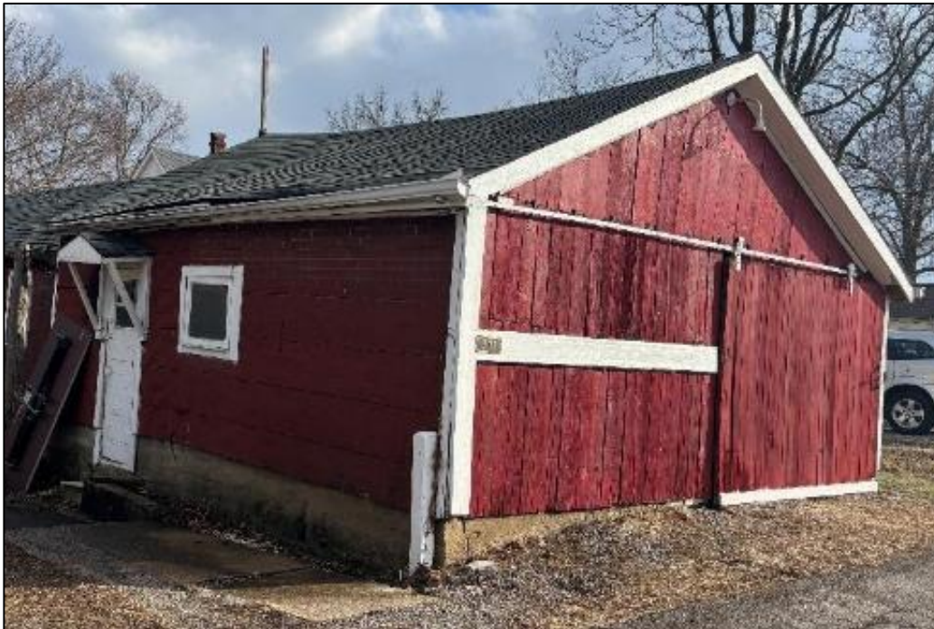
Figure 3: Subject detached garage in the rear of the property.
