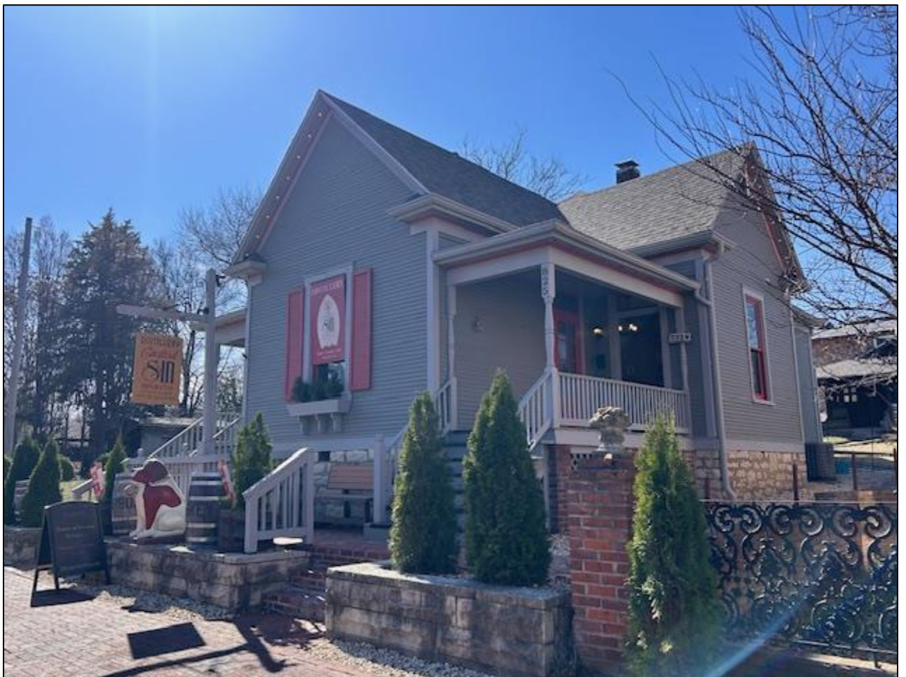
Figure 1: Primary structure seen from South Main Street.
