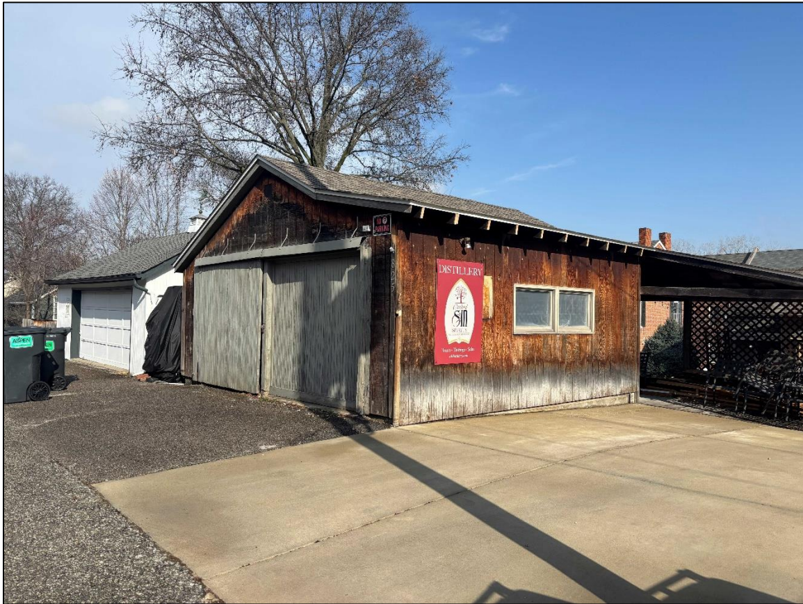
Figure 7: Garage seen currently from rear alleyway.
