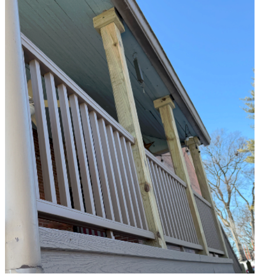
Railing type/color to be installed to Replace existing treated wood.
