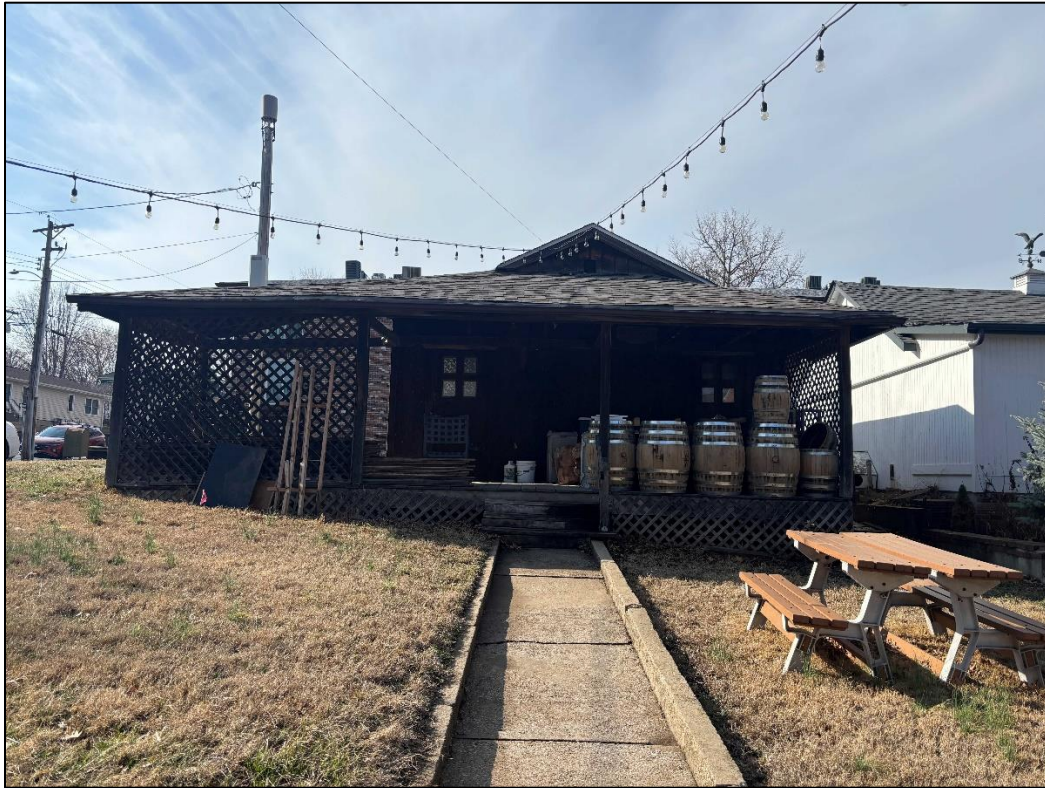
Figure 5: Rear garage currently with porch and roof covering.
