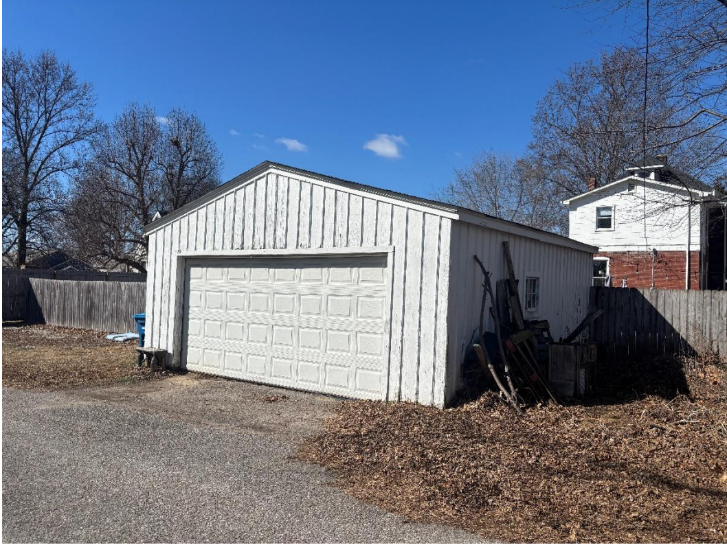
Existing Photo, Feb. 2026 - Garage View from Alley
