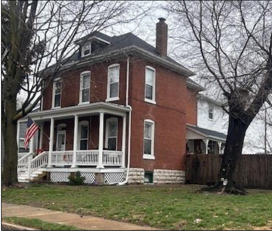
Figure 5: 912 South 4 th Street seen from the road.
