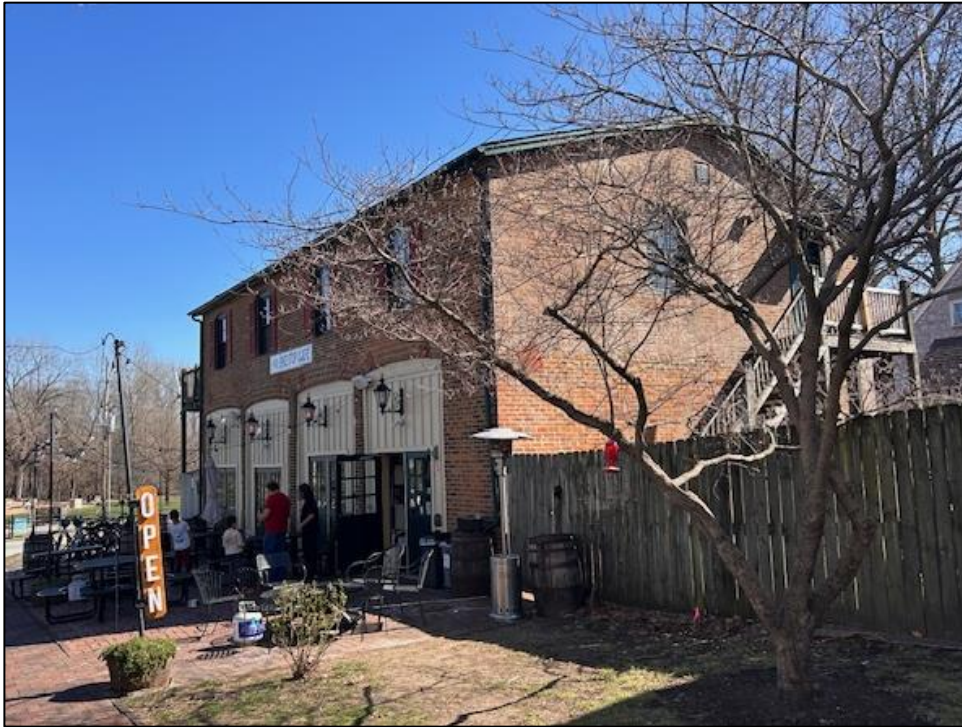
Figure 1: Subject building seen from Perry Street walkway.
