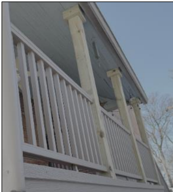
Figure 4: Replacement railing example.
