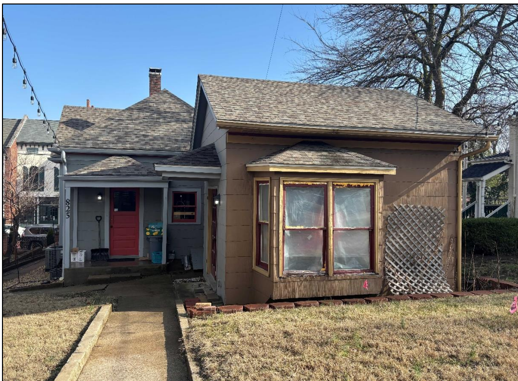
Figure 6: Rear addition on primary structure.
