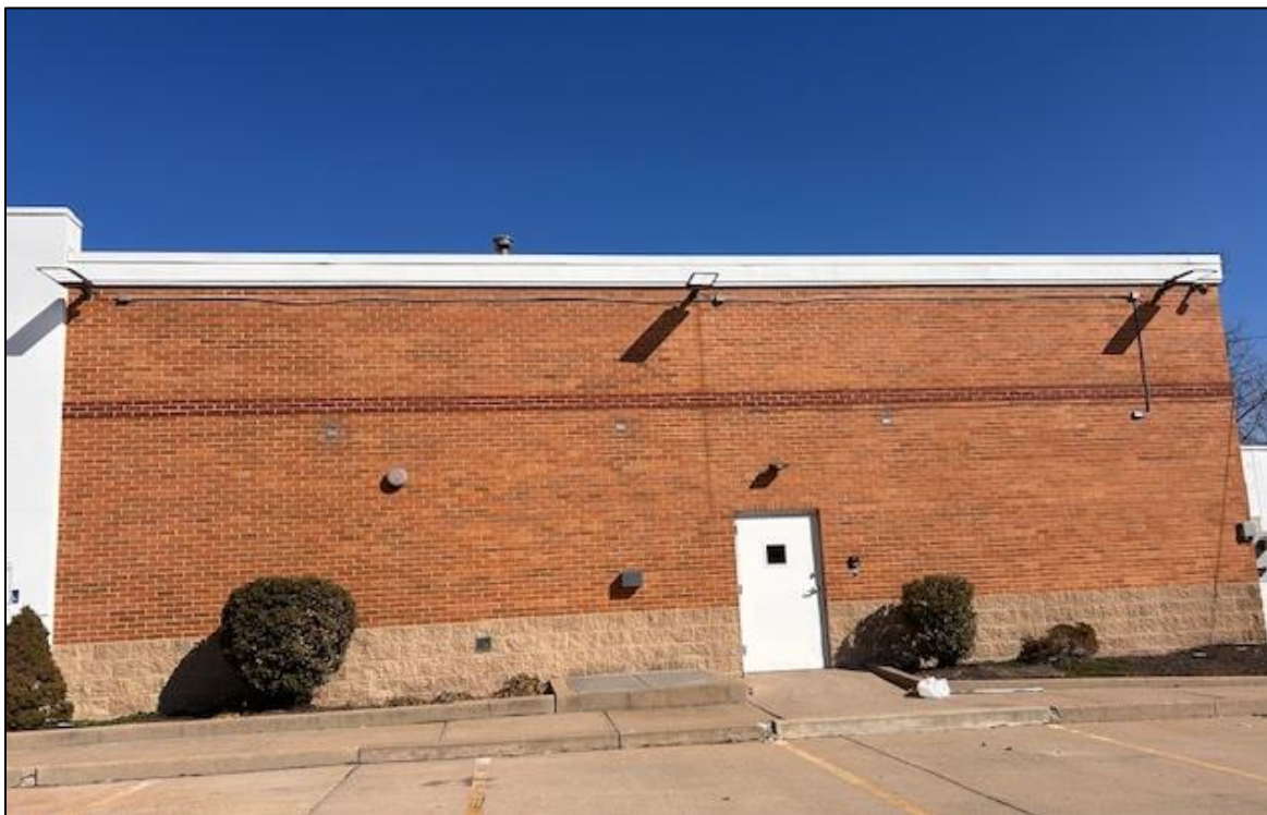
Figure 2: Existing light locations on the south side of structure.
