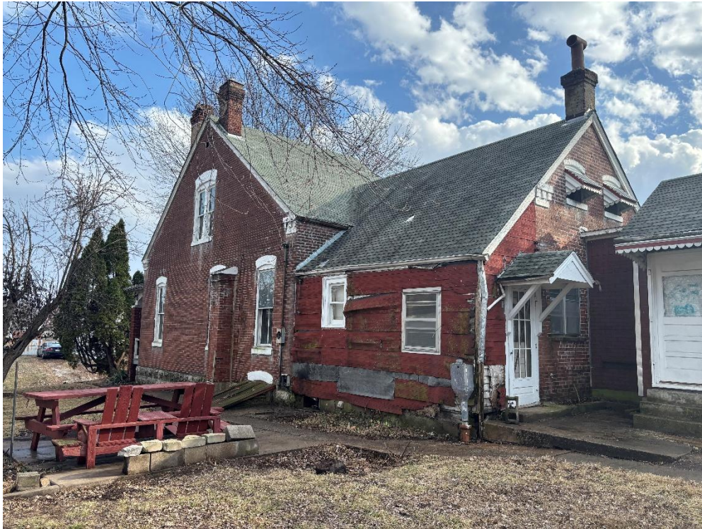
Existing Photo, Feb. 2026 – View of house from side yard looking southeast. Original 1890 structure shown to left. Likely masonry addition at rear of house to the right with wood porch depicted in 1909 & 1917 Sanborn maps infilled. To the far right is the start of the addition requested to be demolished.
