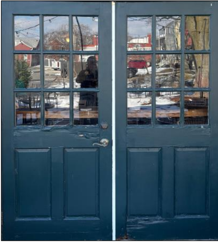
Figure 5: Existing doors example.
