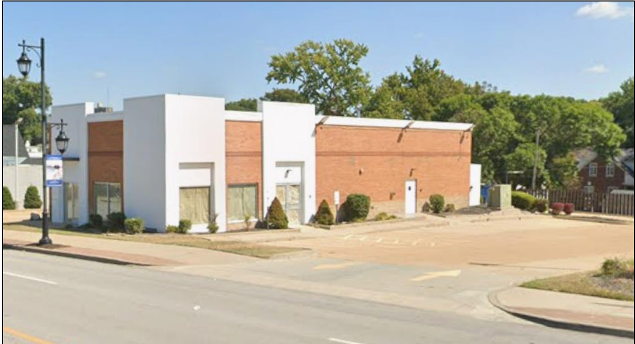
Figure 1: Subject structure seen from South 5 th Street.
