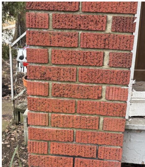
Existing Photo, Feb. 2026 - Brick porch column.
