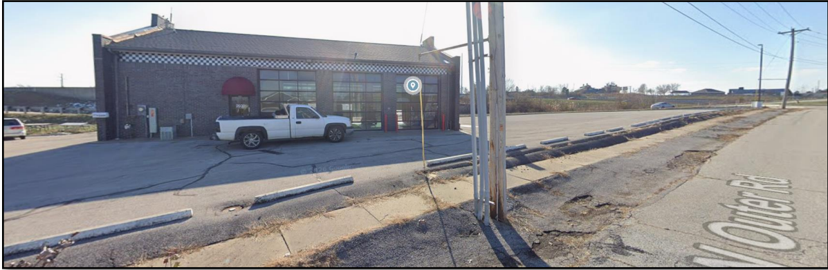
Figure 4: Street view of the subject property.
