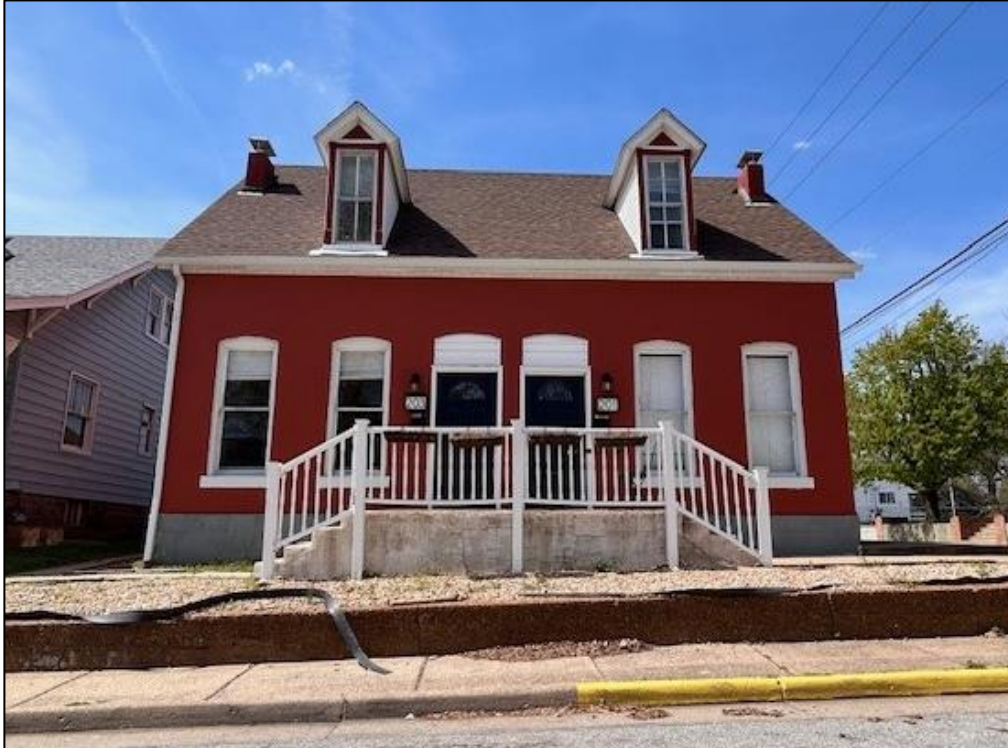
Figure 2: 201 South 7 th Street seen from the roadway.
