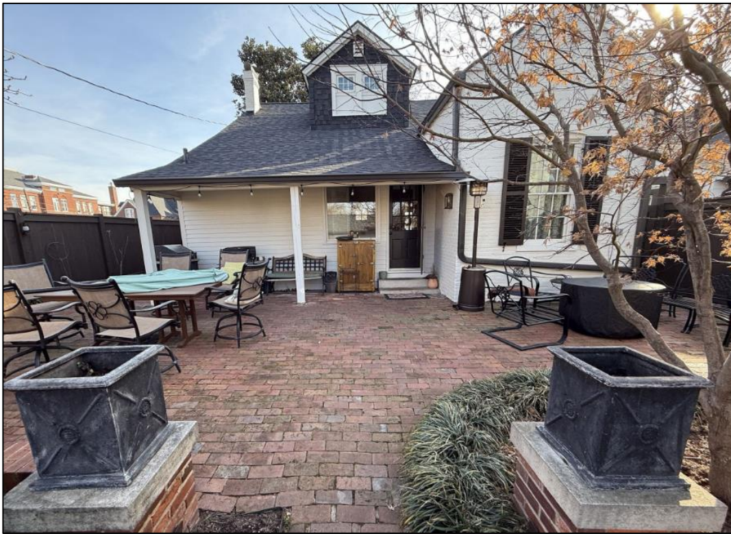
Figure 2: Rear patio currently.
