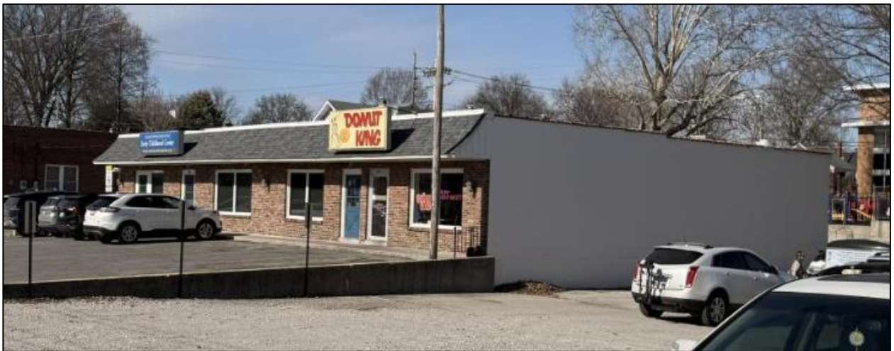
Figure 3: Subject structure seen looking west.
