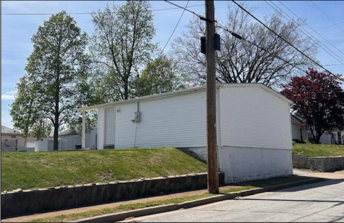
Figure 5: Non-historic rear detached garage.
