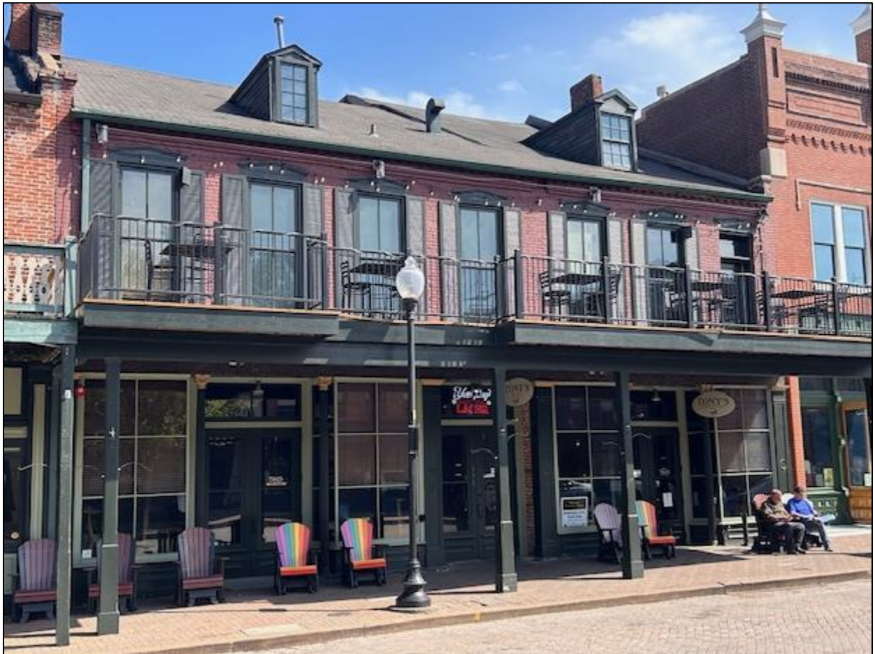
Figure 1: Subject structure seen from Main Street.
