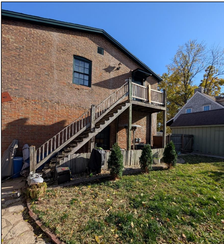
Figure 2: Subject staircase and deck seen currently.
