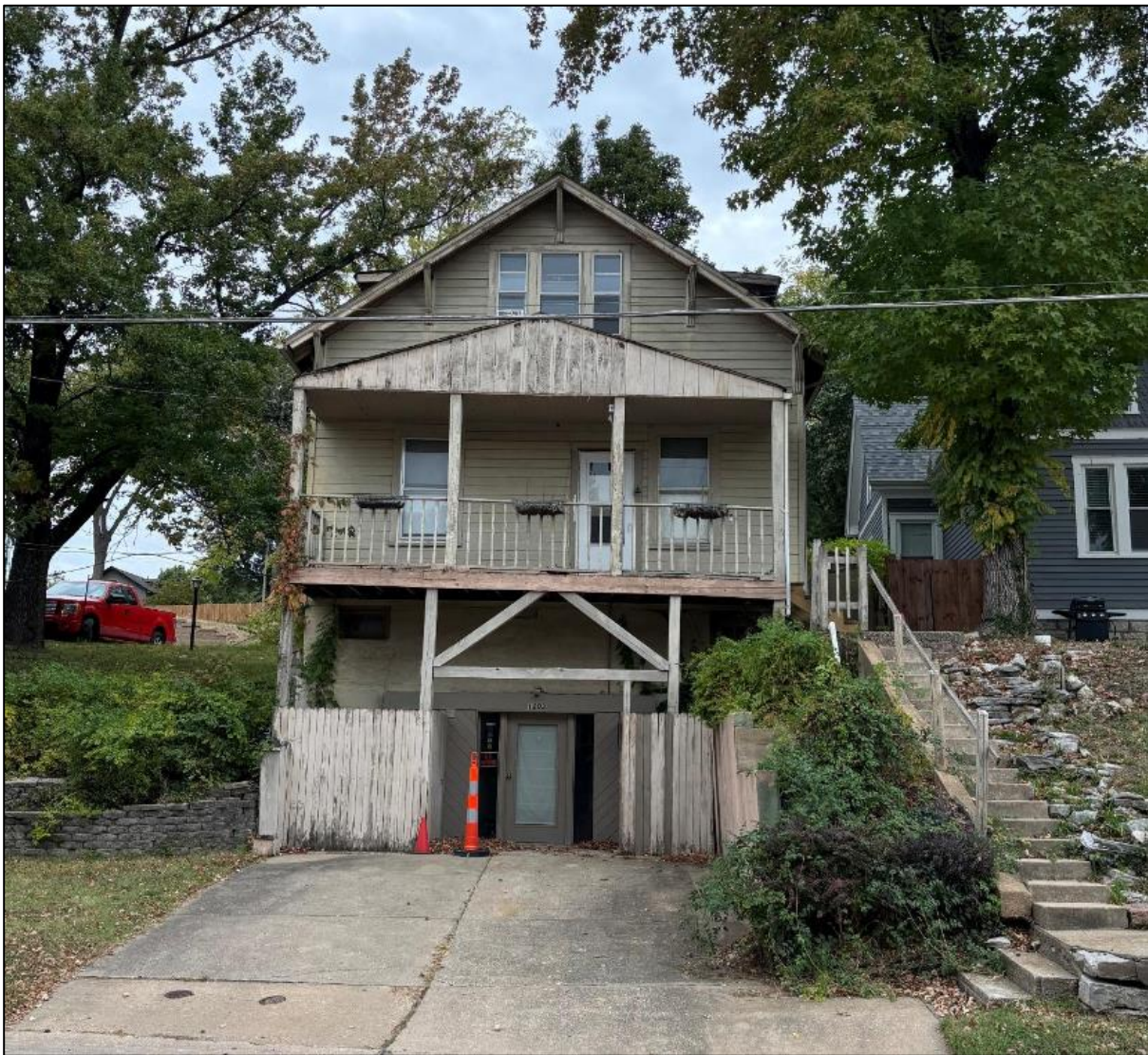
Figure 3: Structure currently on property approved for removal.
