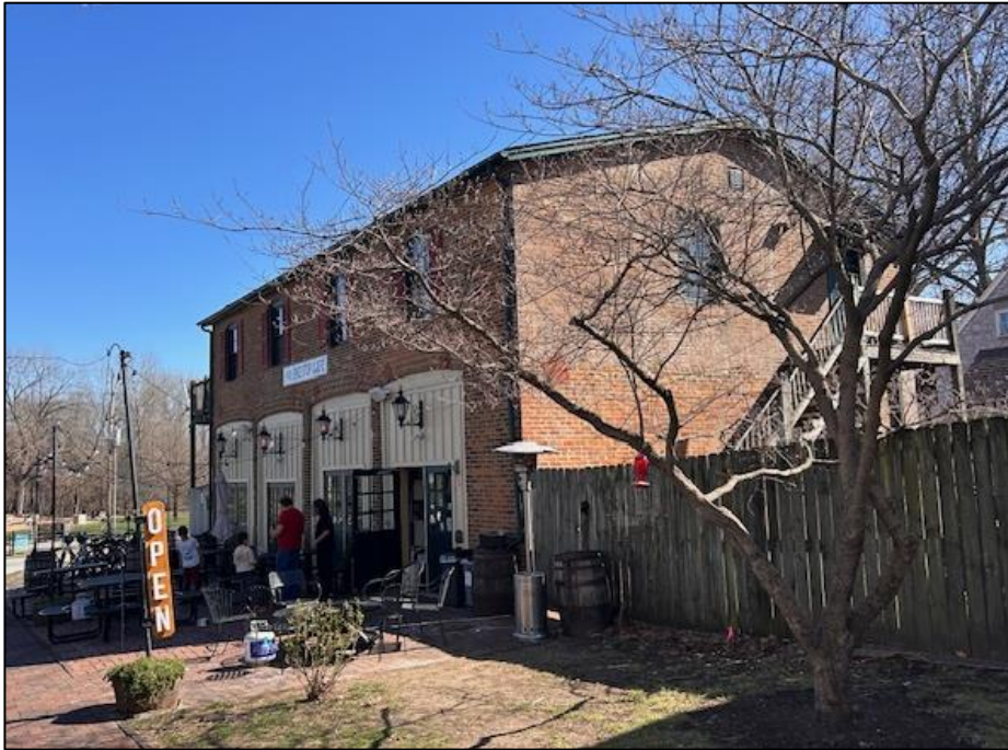
Figure 1: Subject building seen from Perry Street walkway.
