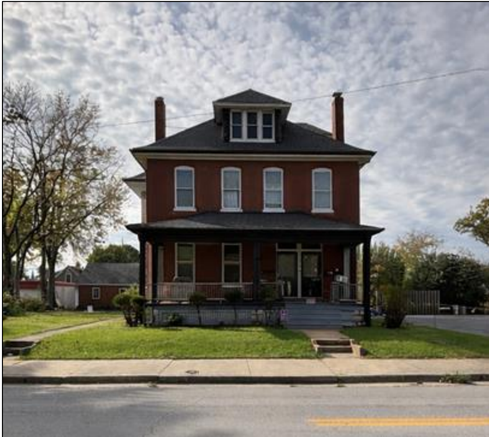
Figure 7: Example of property after completed work.
