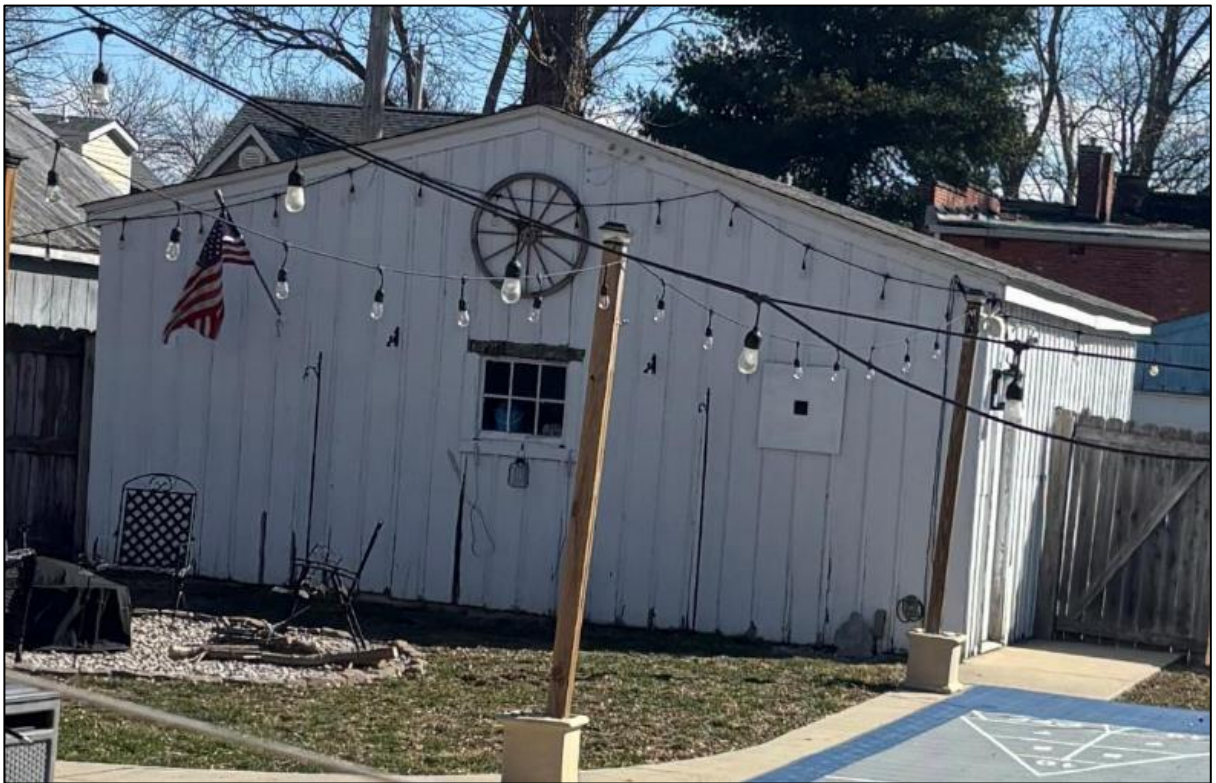
Figure 3: Subject structure seen from rear yard on the property.
