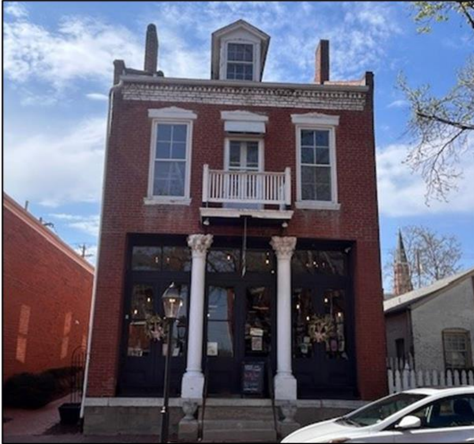
Figure 1: 337 South Main Street seen from the roadway.
