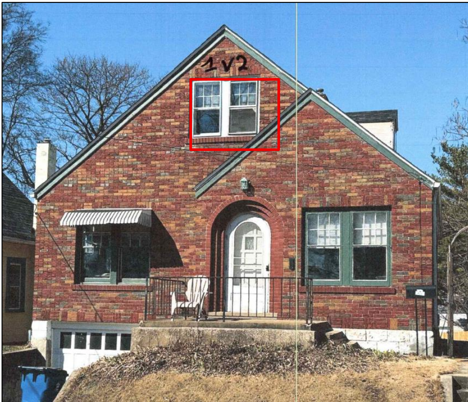
Figure 2: Window 1 and 2 for replacement (exterior muntins).
