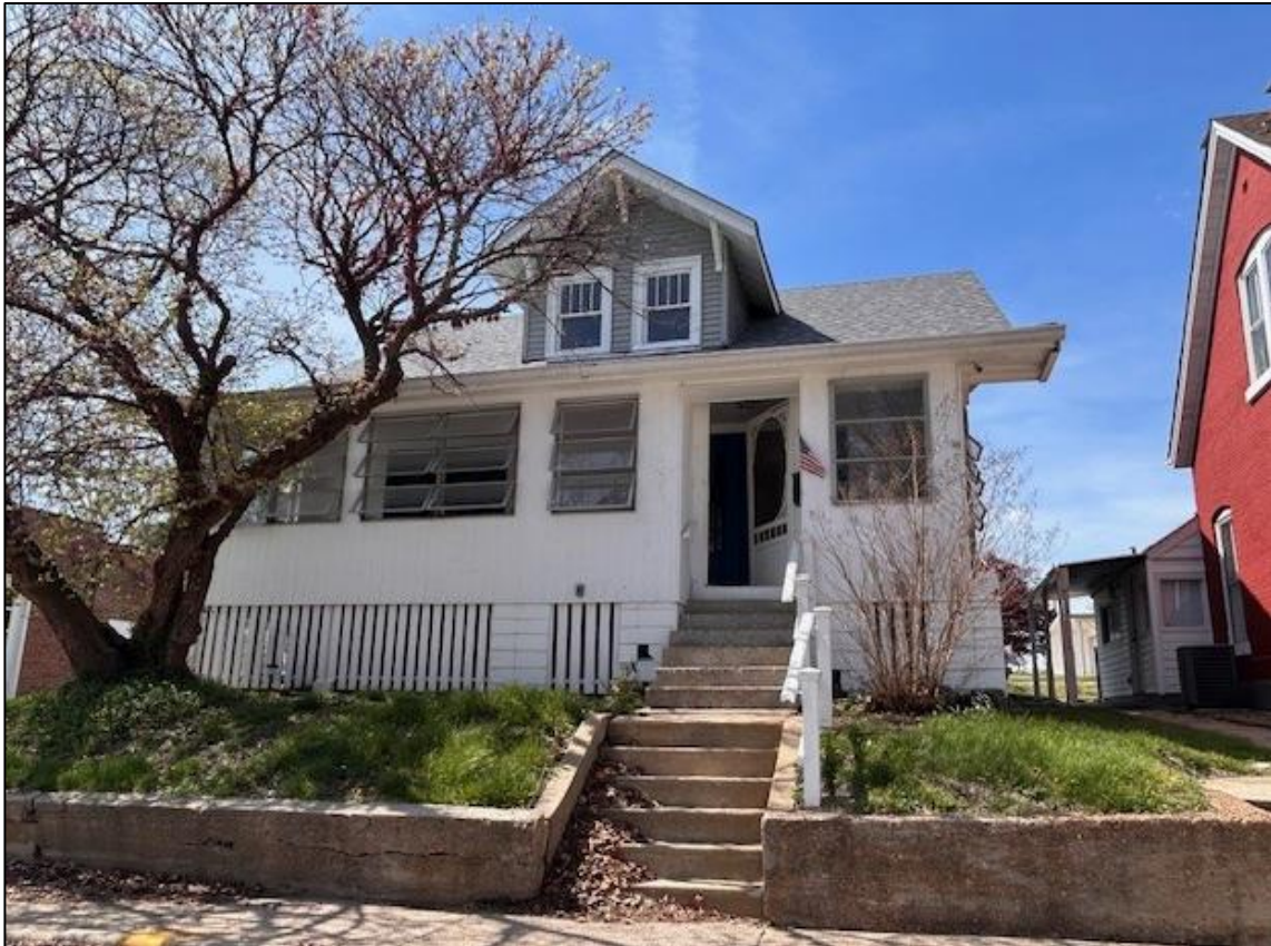
Figure 2: 209 South 7 th Street seen from the roadway.
