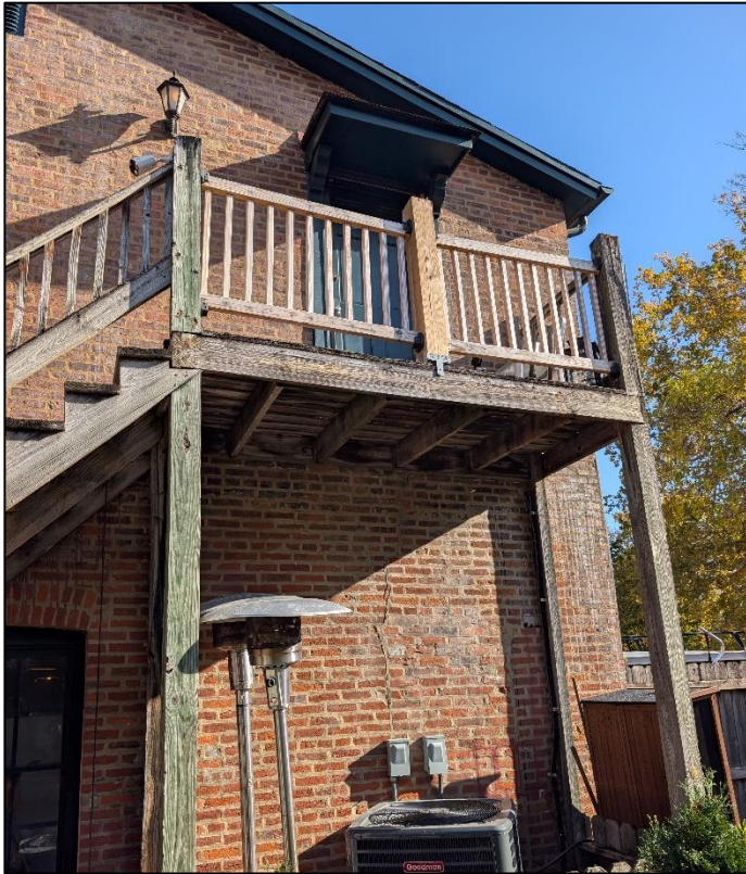
Figure 3: View of existing handrails.
