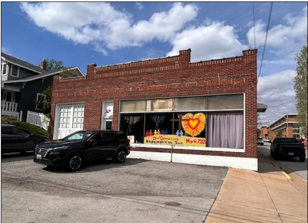
Figure 2: 700 First Capitol seen from the roadway.
