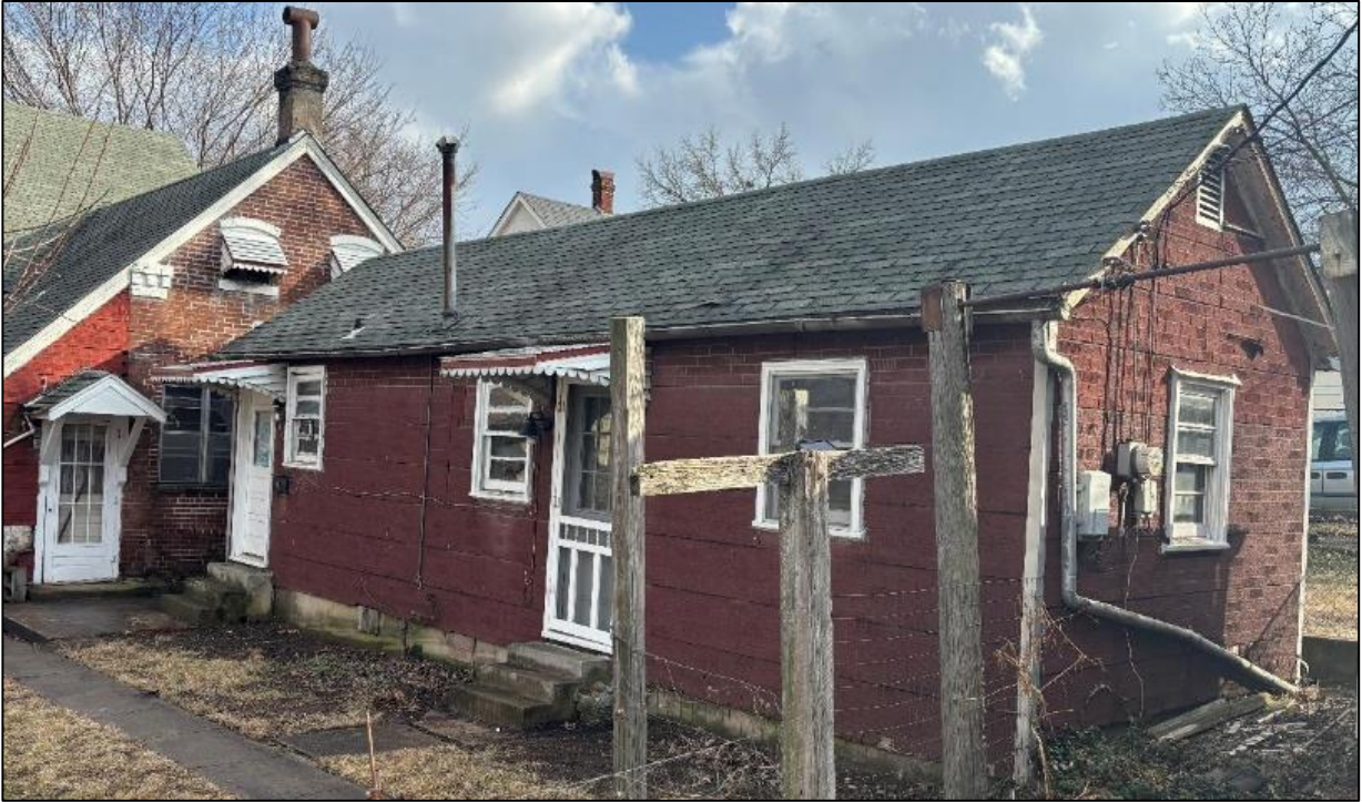
Figure 2: Subject rear addition seen currently.
