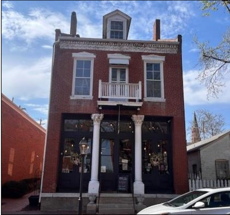
Figure 1: Subject property seen from street.
