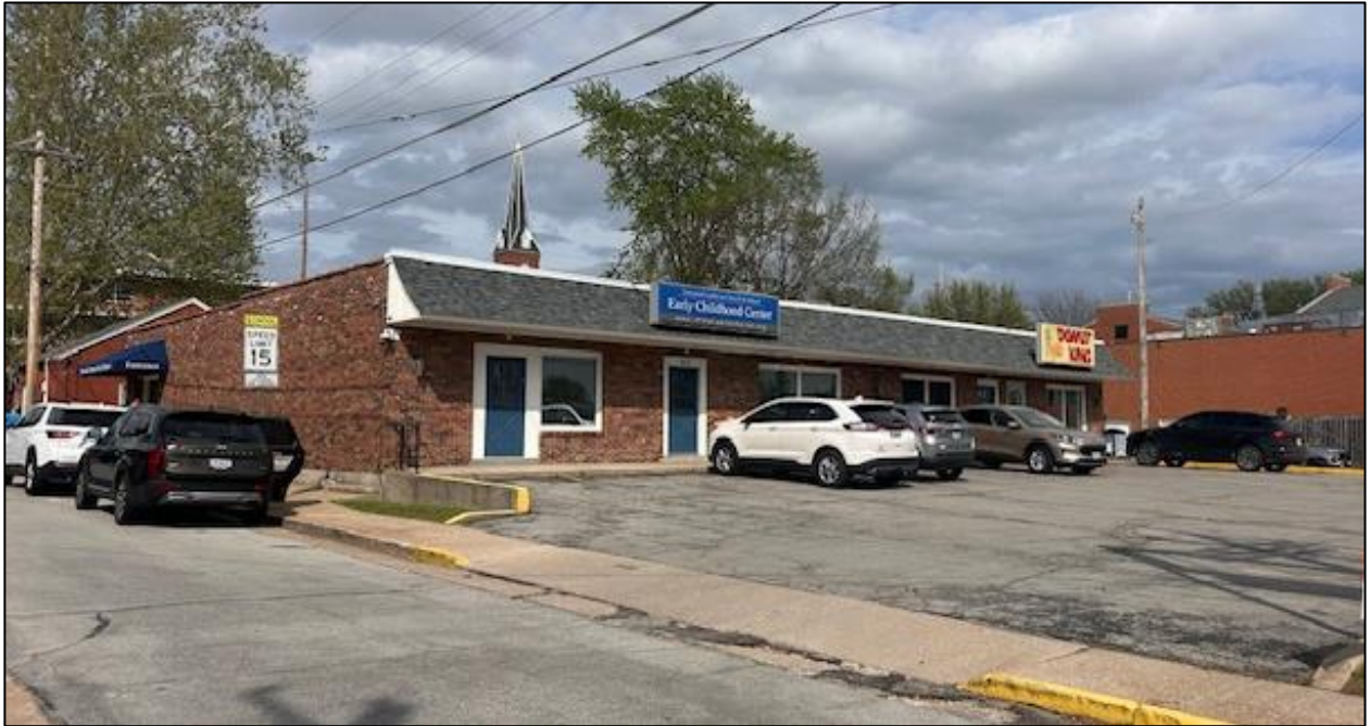
Figure 4: Subject structure looking east.
