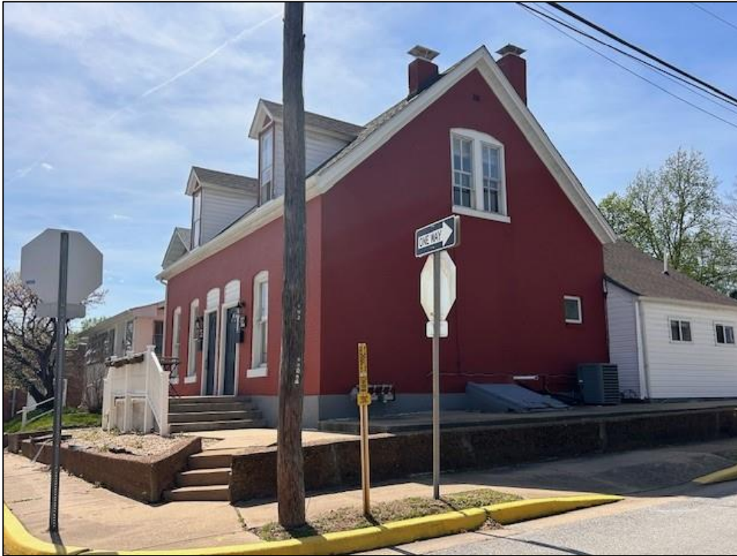
Figure 3: Subject structure seen from the corner of Madison and South 7 th Streets.
