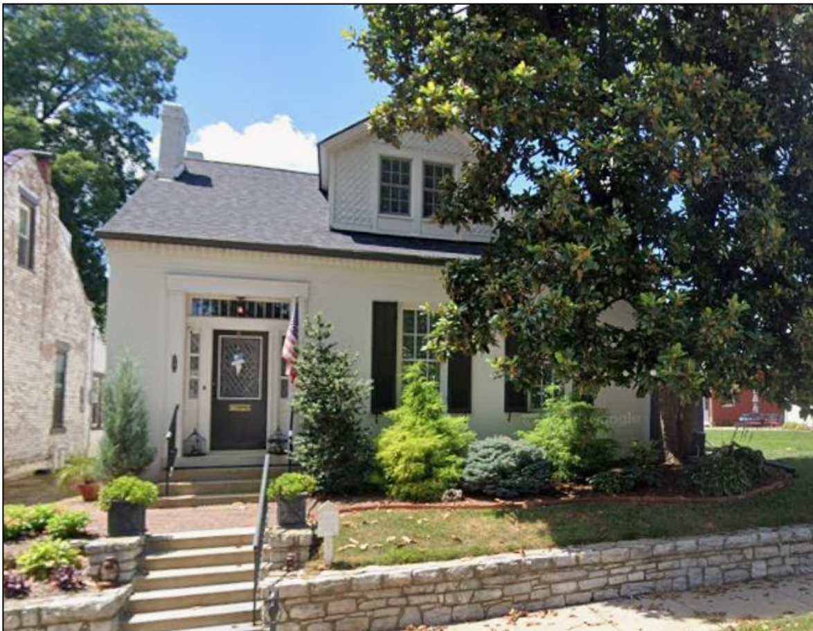
Figure 1: 317 North 6 th Street seen from the roadway.
