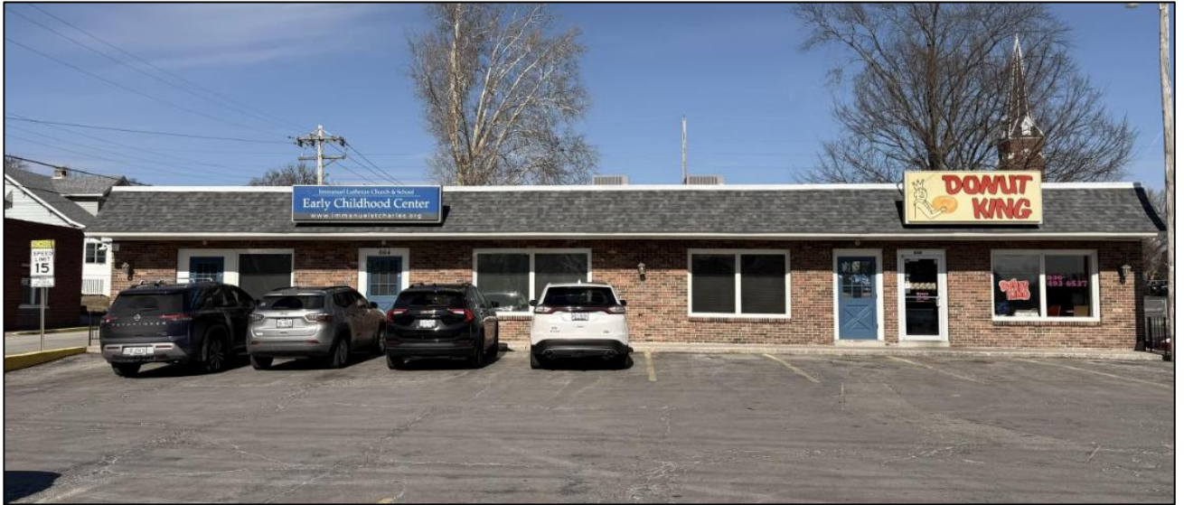
Figure 2: 664 First Capitol seen from the roadway.
