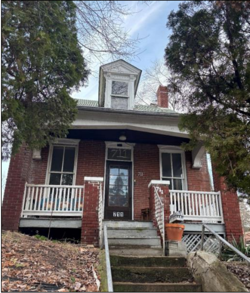
Figure 4: Subject primary structure located on the property.
