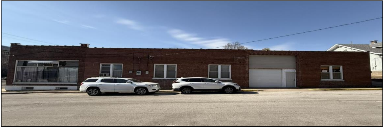
Figure 3: Side elevation of subject structure seen from South 7 th .
