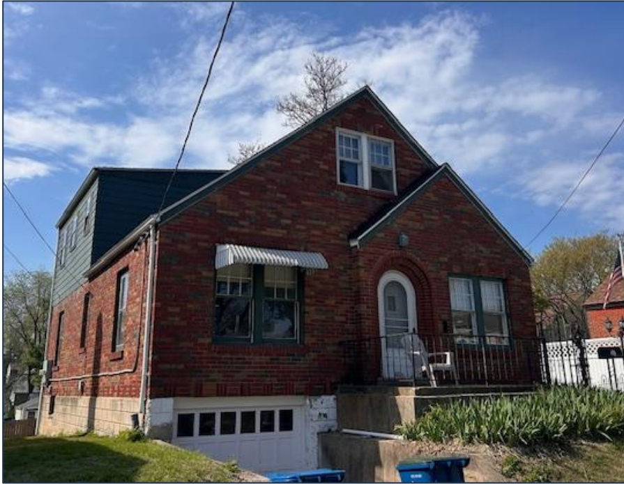
Figure 1: Subject structure seen from South 3 rd Street.
