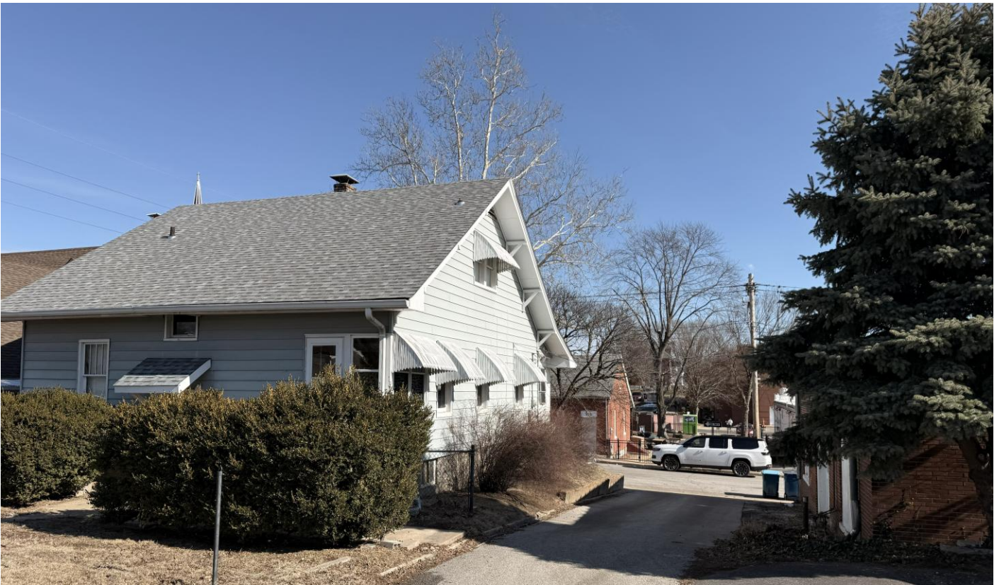
209 S 7 th Street – Rear / Side Elevation
