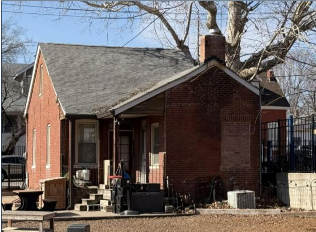
Figure 3: Rear of subject structure.
