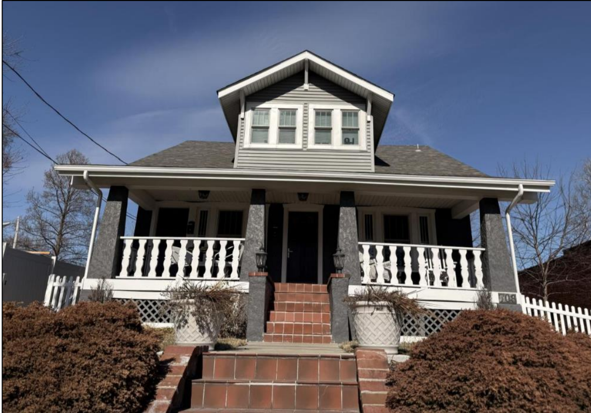
Figure 2: 708 First Capitol seen from the roadway.
