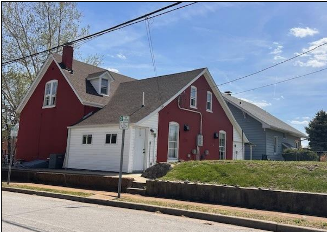
Figure 4: Subject structure's rear seen from Madison Street.
