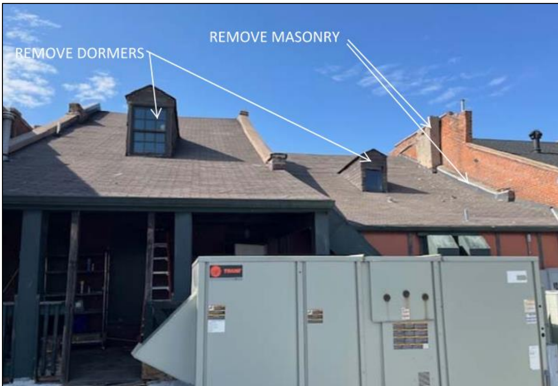
Figure 3: Rear dormers and masonry element seen from rear roof.
