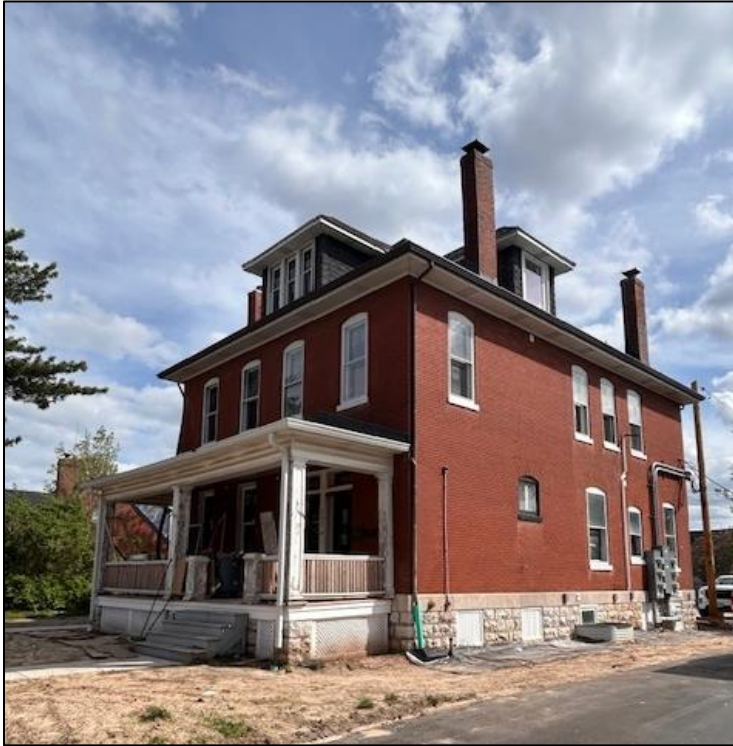
Figure 2: Subject property looking east.
