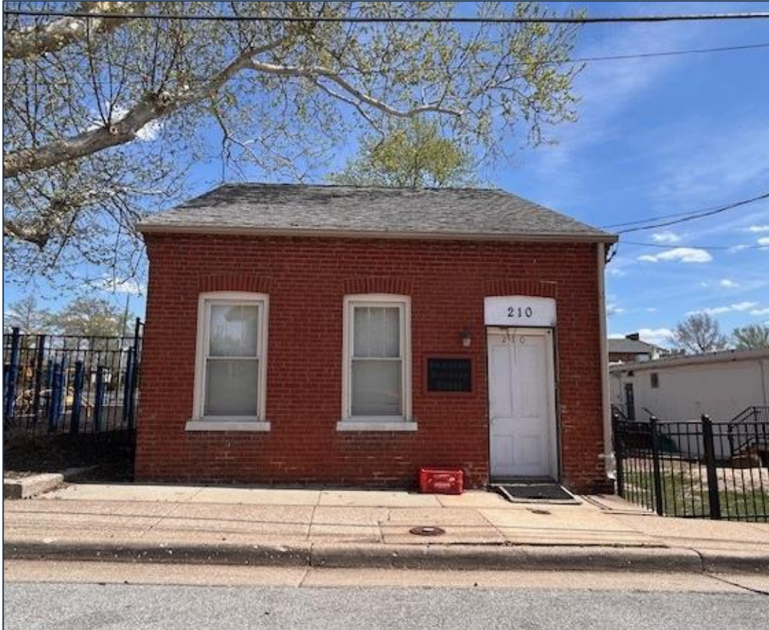
Figure 2: 210 South 7 th Street seen from roadway.
