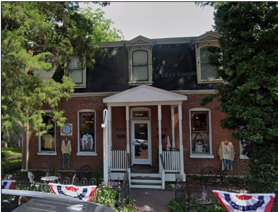
Figure 1: Subject property seen from South Main Street
