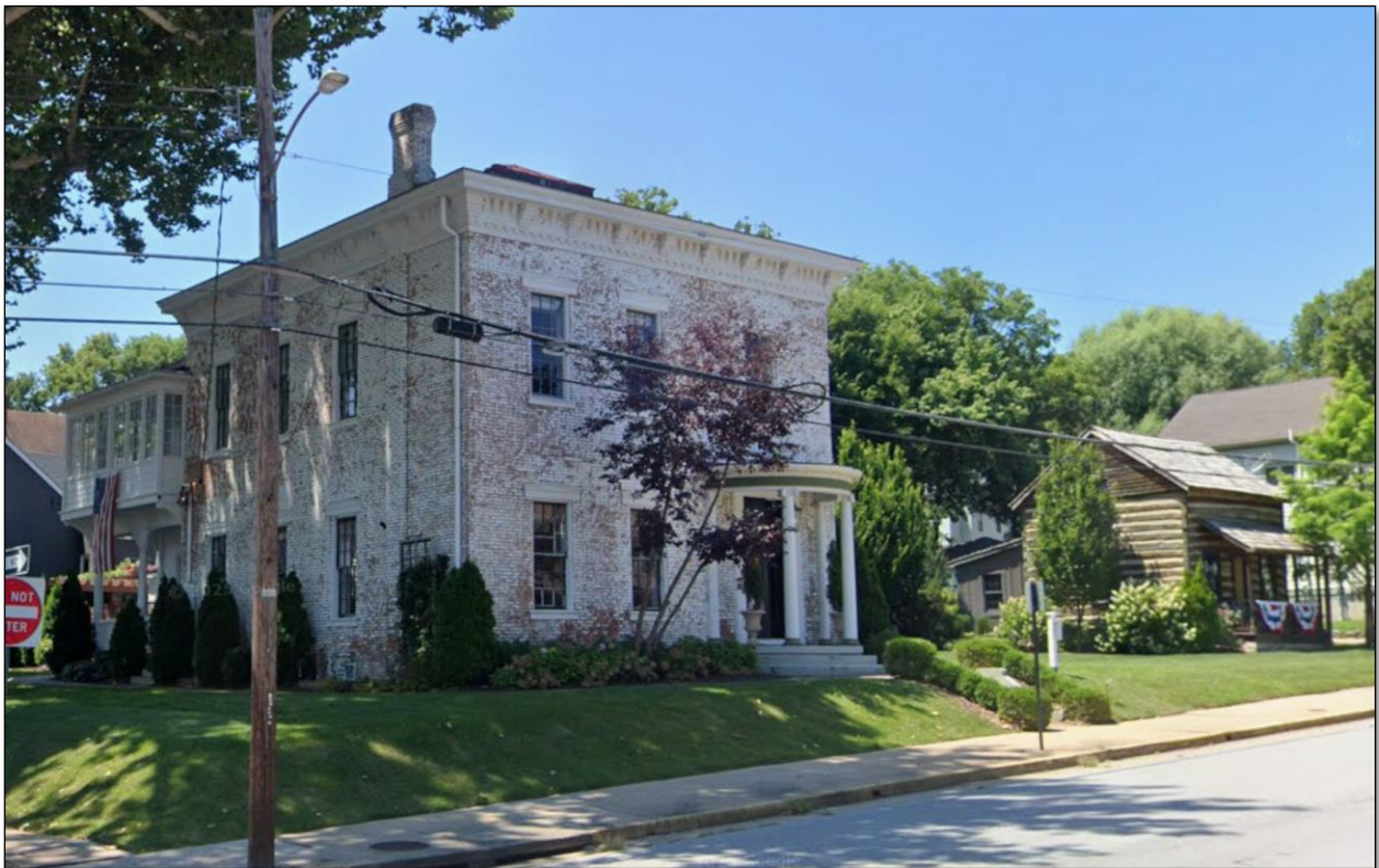
Figure 6: Street view of the subject property.
