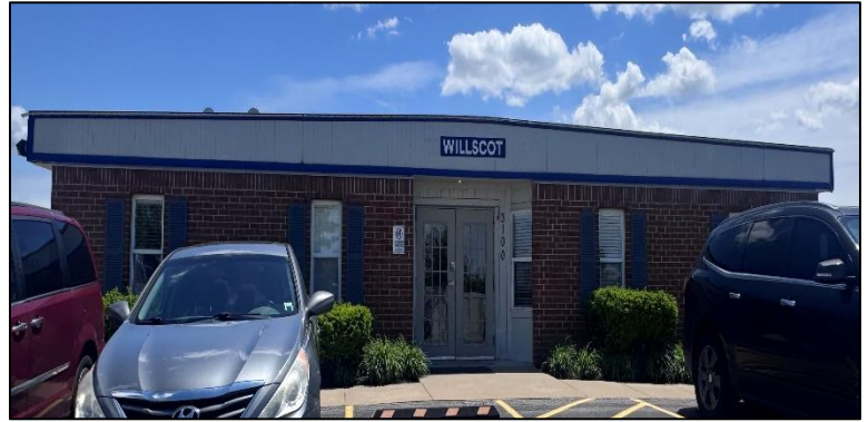
Figure 2: Office building at 3100 Harry S Truman Blvd.
