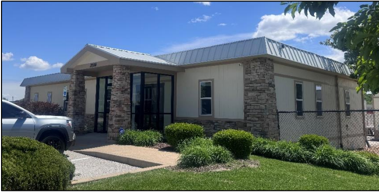
Figure 1: Office building at 2000 Truman Industrial Blvd.
