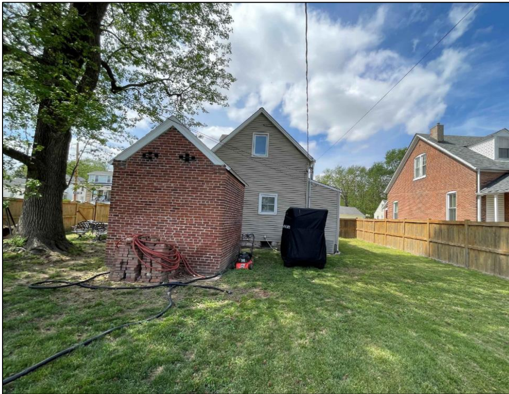
Figure 6: Rear of primary structure seen from back yard.
