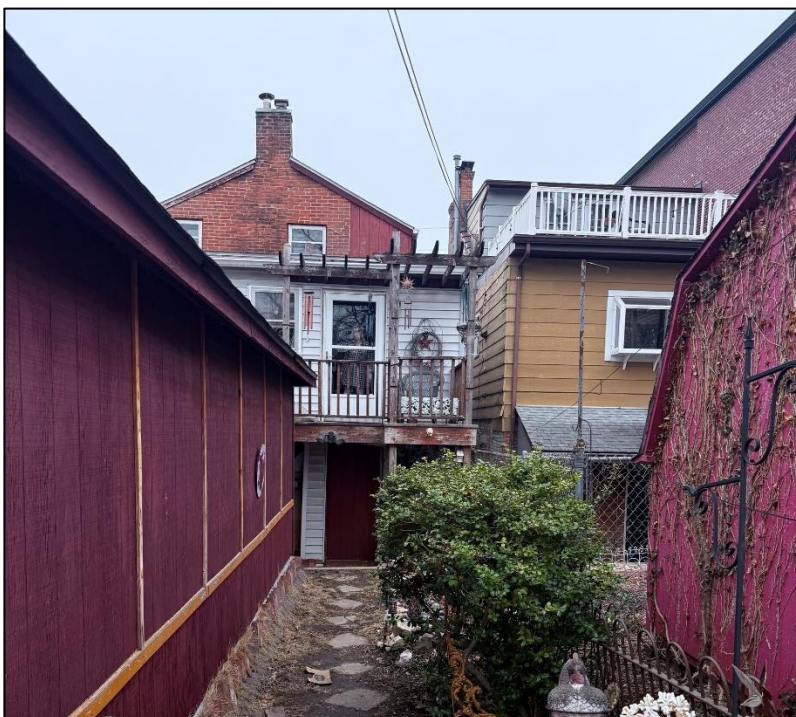
Figure 2: Subject deck seen from rear of property.
