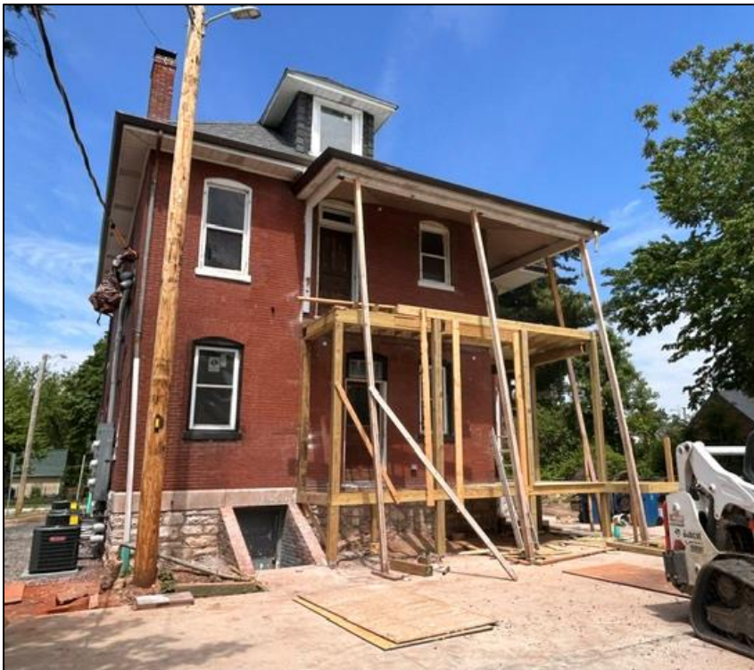
Figure 4: Rear of structure seen currently with two-tier deck construction.
