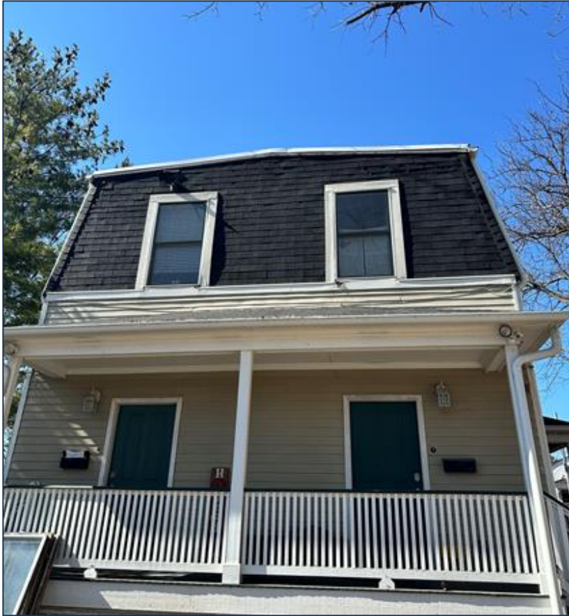
Figure 2: Rear addition with siding on gable.
