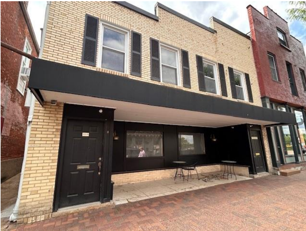
Figure 2: Existing storefront seen on property.
