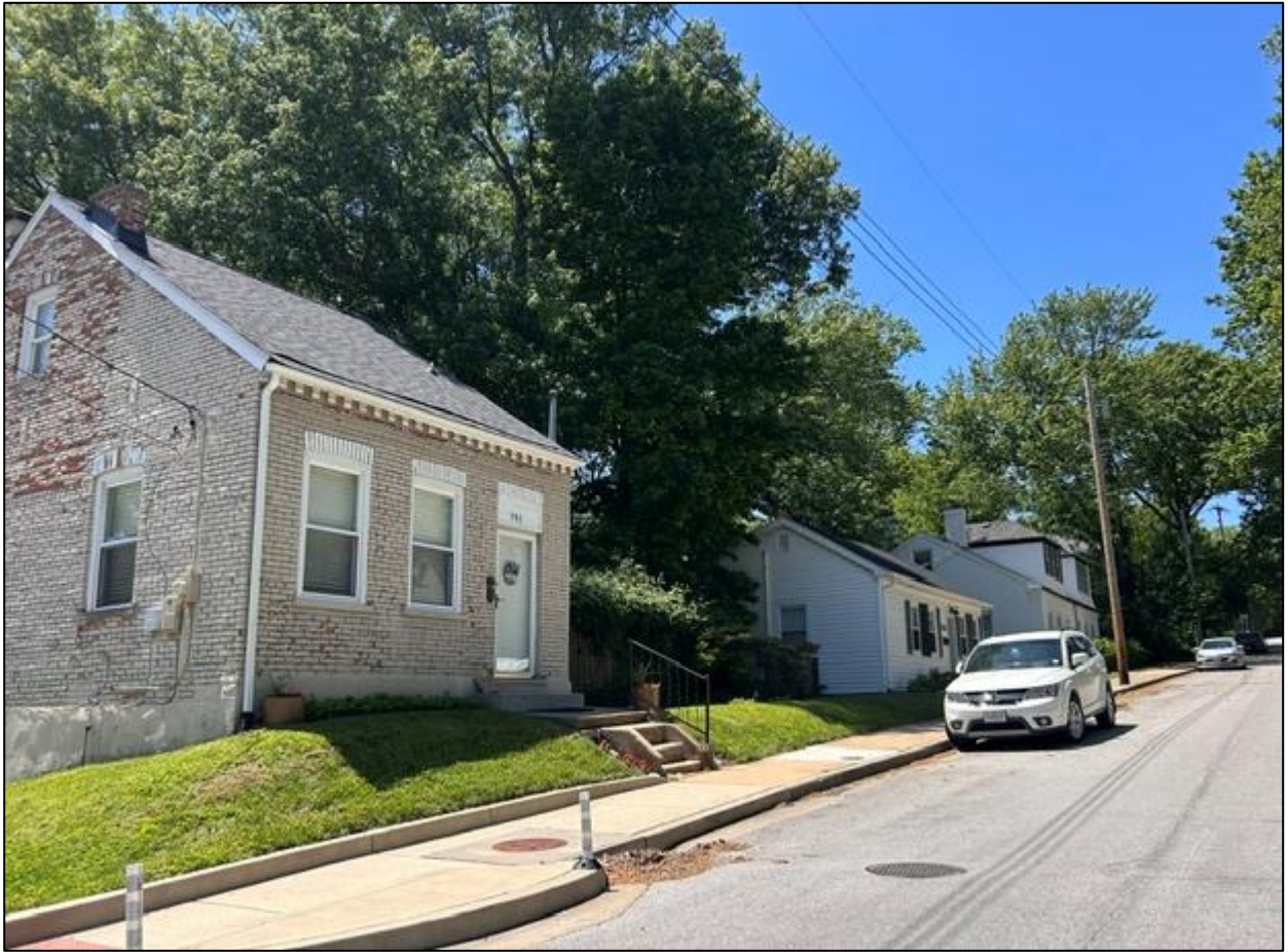
Figure 11: Existing structures looking west.
