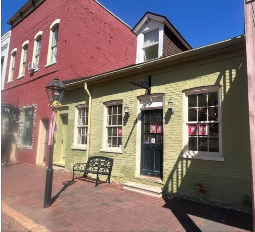
Figure 1: Subject structure seen from South Main Street.
