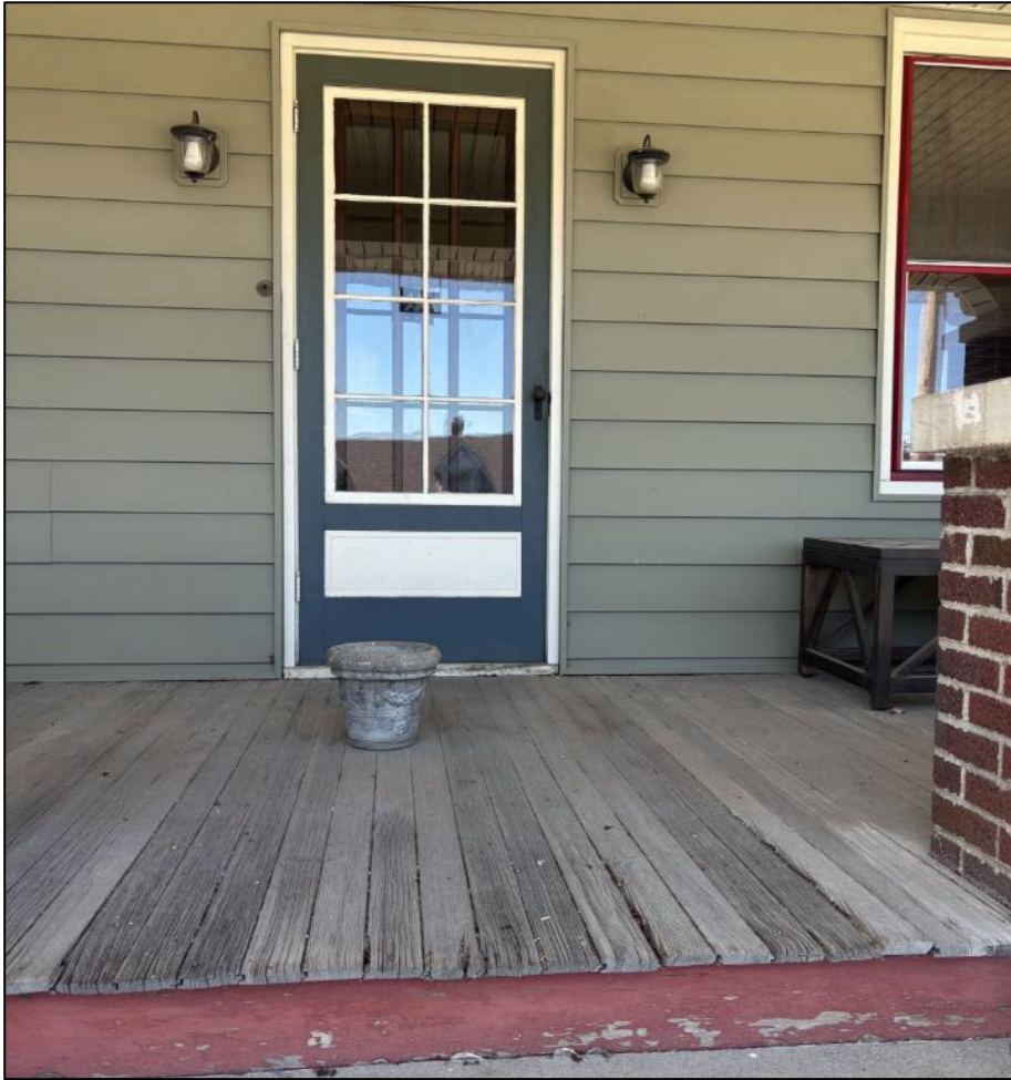
Figure 3: Existing flooring on front porch.
