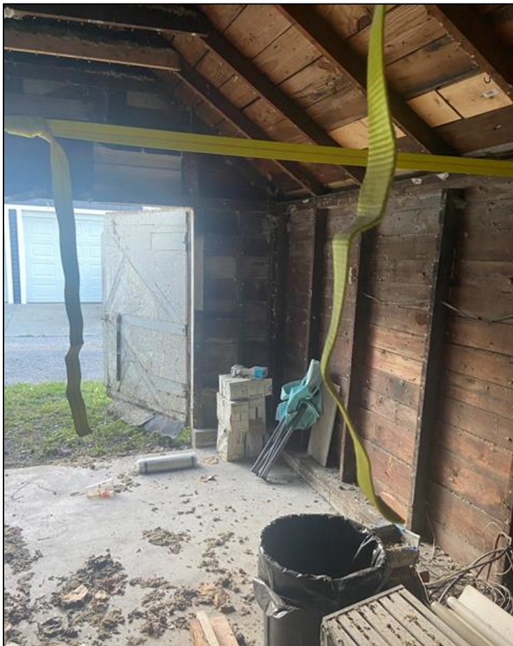
Figure 6: Interior photo of structure.
