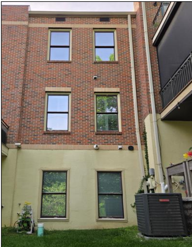
Figure 2: Rear windows on the structure seen currently.
