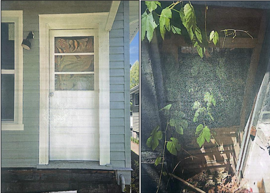
Figure 4: Subject rear doors (leading to deck and basement walkout).
