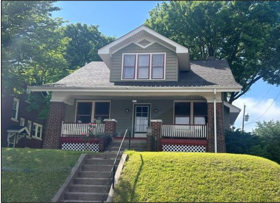
Figure 1: Subject property seen from South 2 nd Street.
