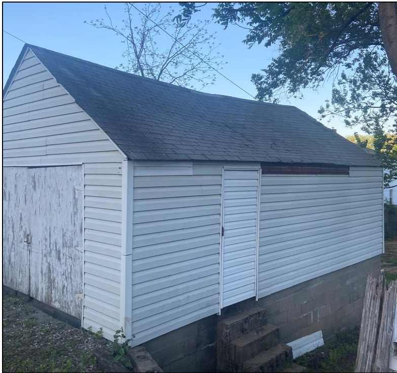
Figure 3: Subject structure's roof seen from alley.
