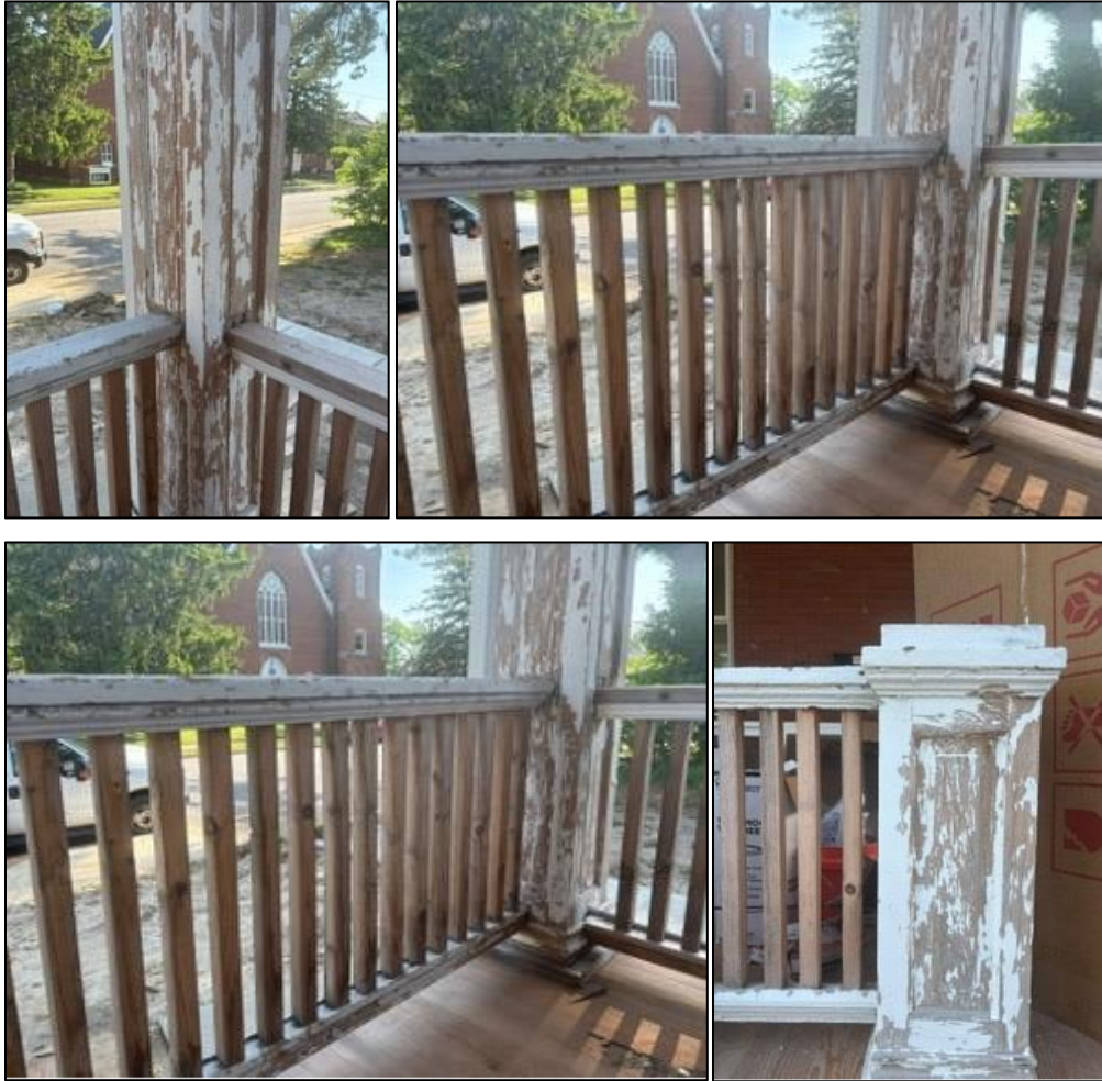
Figure 8: Example photos of existing front porch railing.
