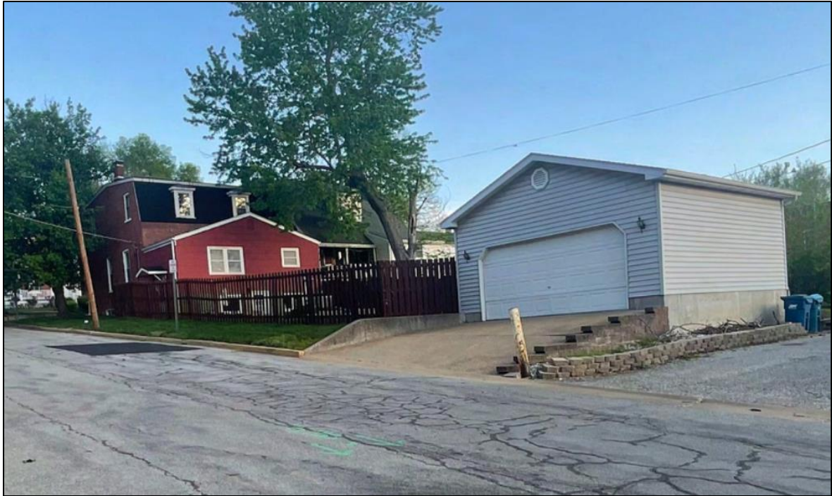
Figure 1: Subject rear garage seen from Decatur Street.
