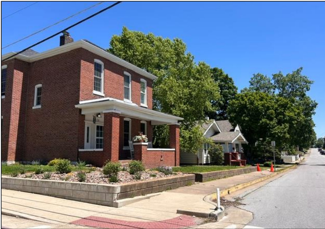
Figure 10: Existing structures looking east.
