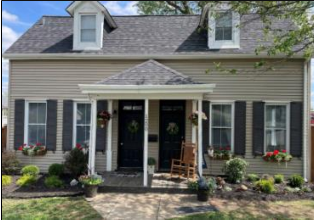
Figure 5: Subject primary structure on the property.
