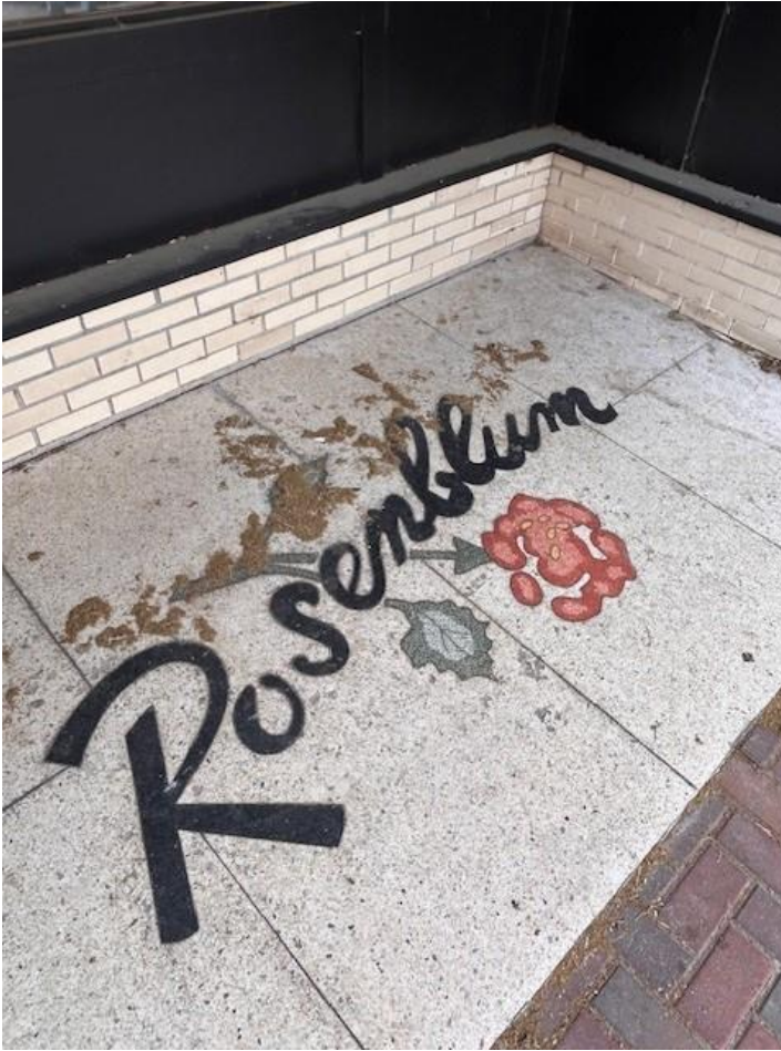
Figure 5: Existing flooring in recessed storefront to be retained.
