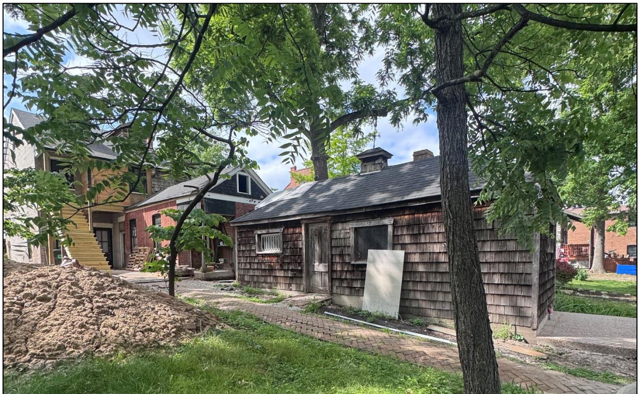
Figure 3: Rear view of subject property.
